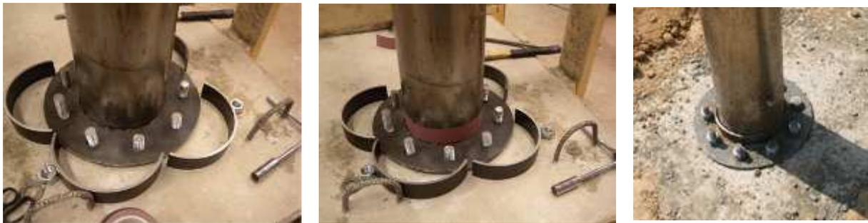
Figure 10: Steel Collar: Components (Left and Middle) and Construction (Right)
