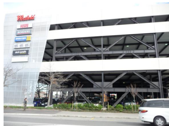
Figure 2: Global elevation of shopping mall on Dilworth St and Clarence St, Christchurch (43°31'53"S-172°36'05"E) [Photo by M. Bruneau].
