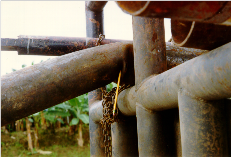
■ Figure 4.1 Local Buckling to RECOPE Pipeline
