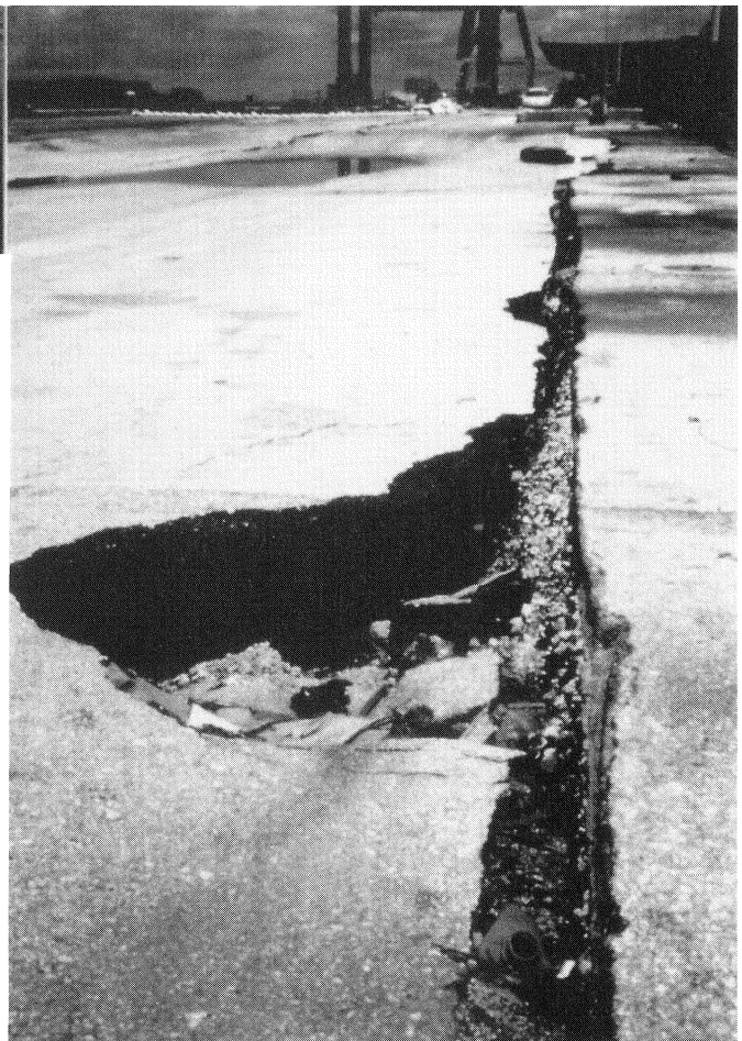
Figure 7: Lateral movement and cracking of the pavement, commercial port facilities
