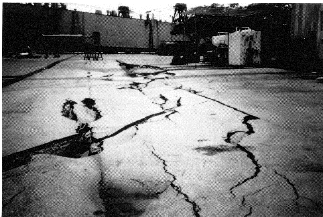
Figure 17: Pattern of lateral soil movement and cracking of the pavement, U.S. Navy port facilities
