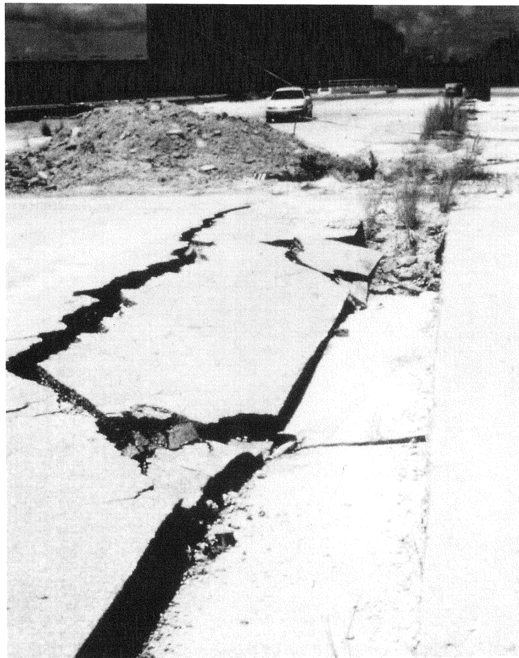
Figure 21: Typical settlement and cracking behind the bulkhead, U.S. Navy port facilities
