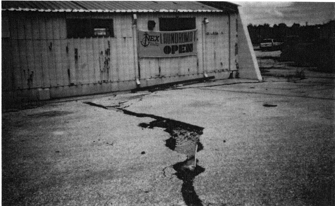
Figure 20: Influence of the presence of the Laundromat building on the pattern of the lateral ground movement
