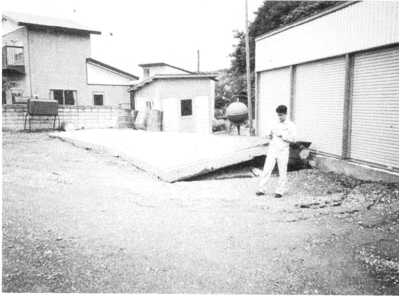
Photo 6 Built-up the Oil pit due to Liquefaction
