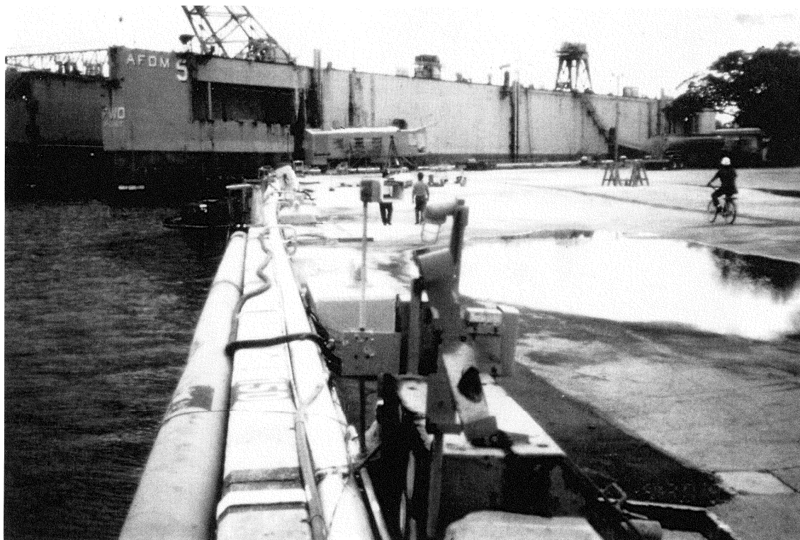
Figure 16: Lateral movement of the bulkhead, U.S. Navy port facilities
