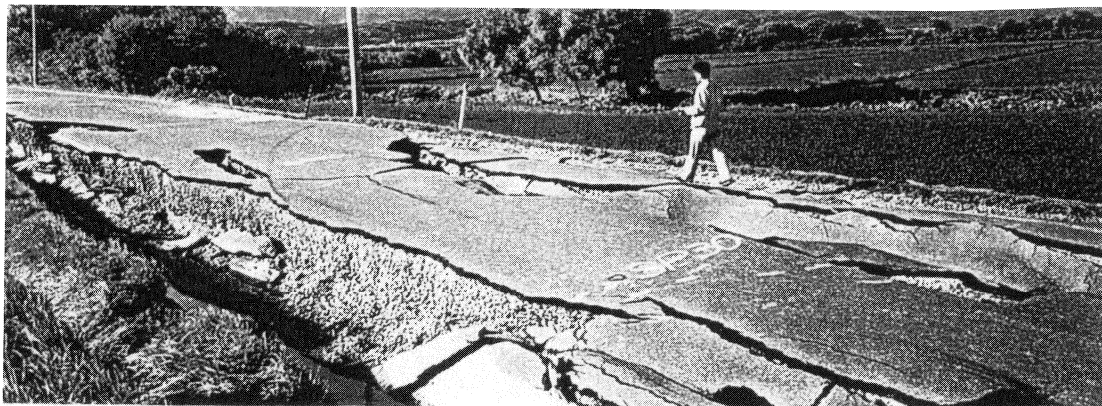
Photo 9 Damage of Road due to Liquefaction
