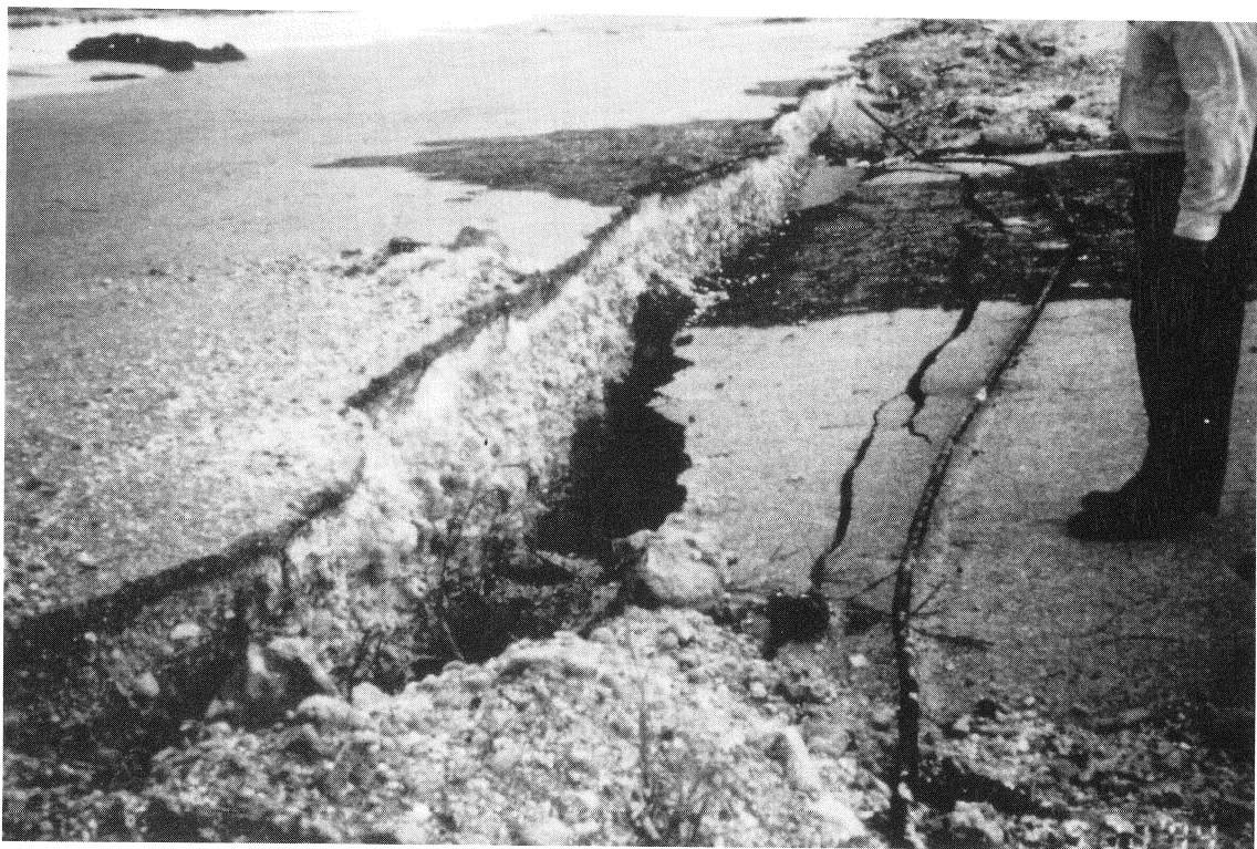
Figure 15: Close-up view of the lateral movement and settlement behind the bulkhead, U.S. Navy port facilities
