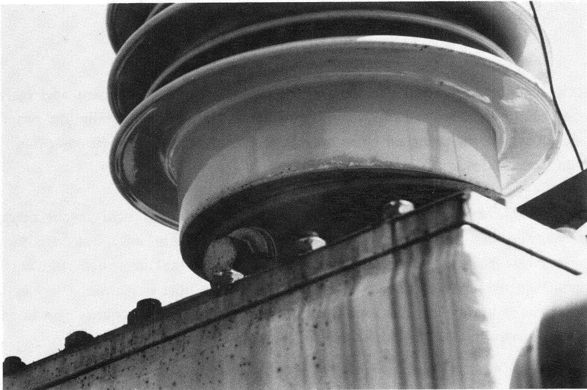
Fig. 1 Shifted Transformer Bushing
