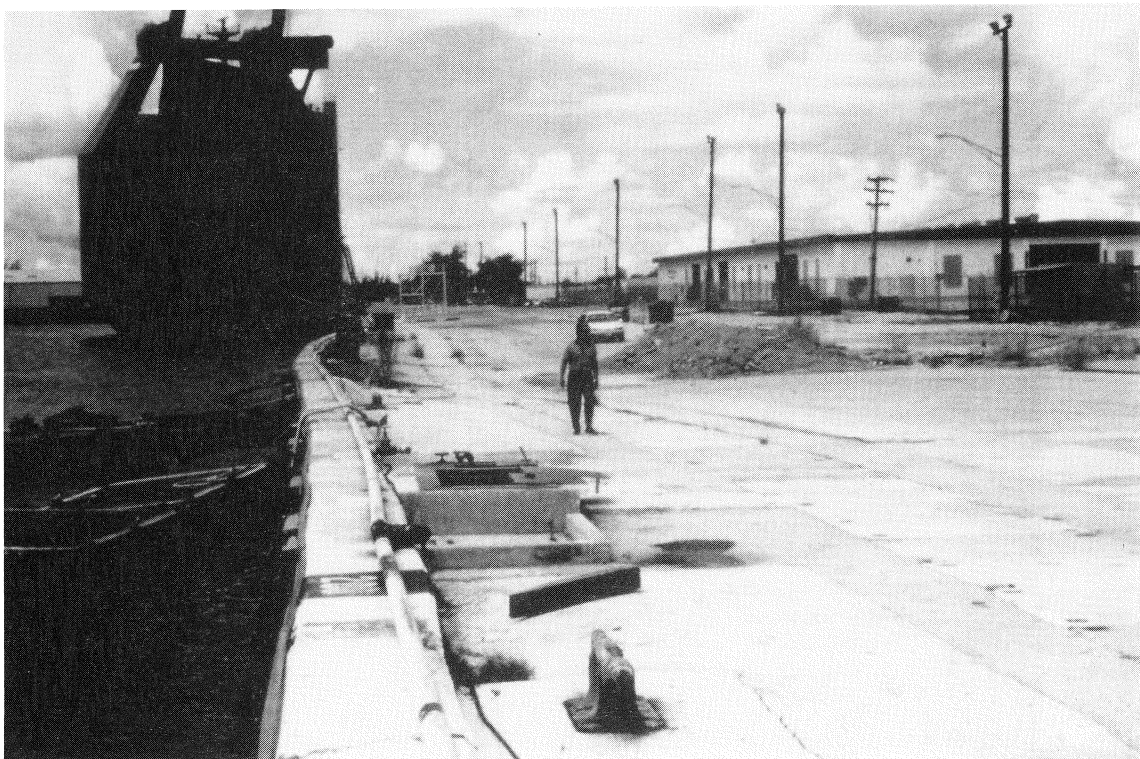
Figure 19: Close-up view of the lateral movement of the bulkhead and settlement at the U.S. Navy port facilities
