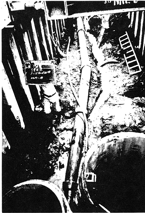
Photo 3 Deformation of a Wastewater Pipeline (Courtesy of Kushiro City Government)
