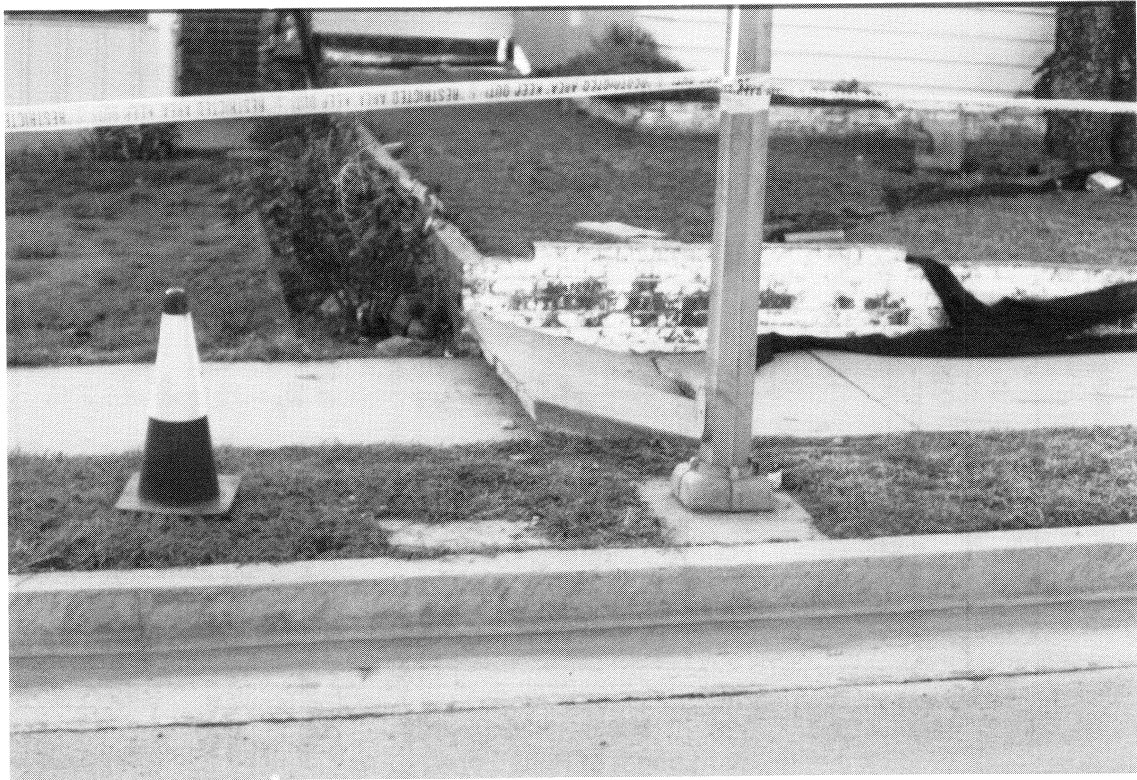
Figure 6 Sidewalk Overlap on West Side of Balboa Blvd., Southern End of PGD Zone
