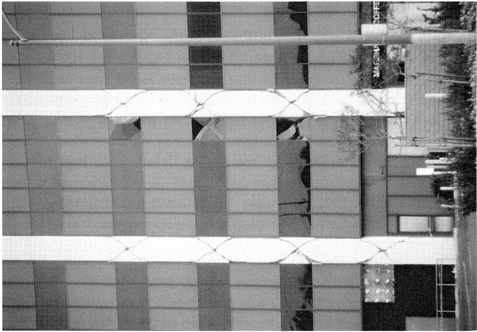
FIGURE 3-33 Typical Shear Cracking Failure from Load Reversals of Short Columns
