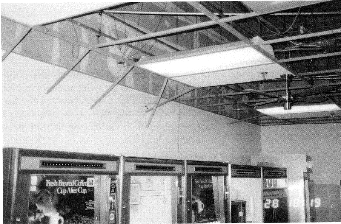
FIGURE 5-1 Typical Post-Earthquake Suspended Ceiling
