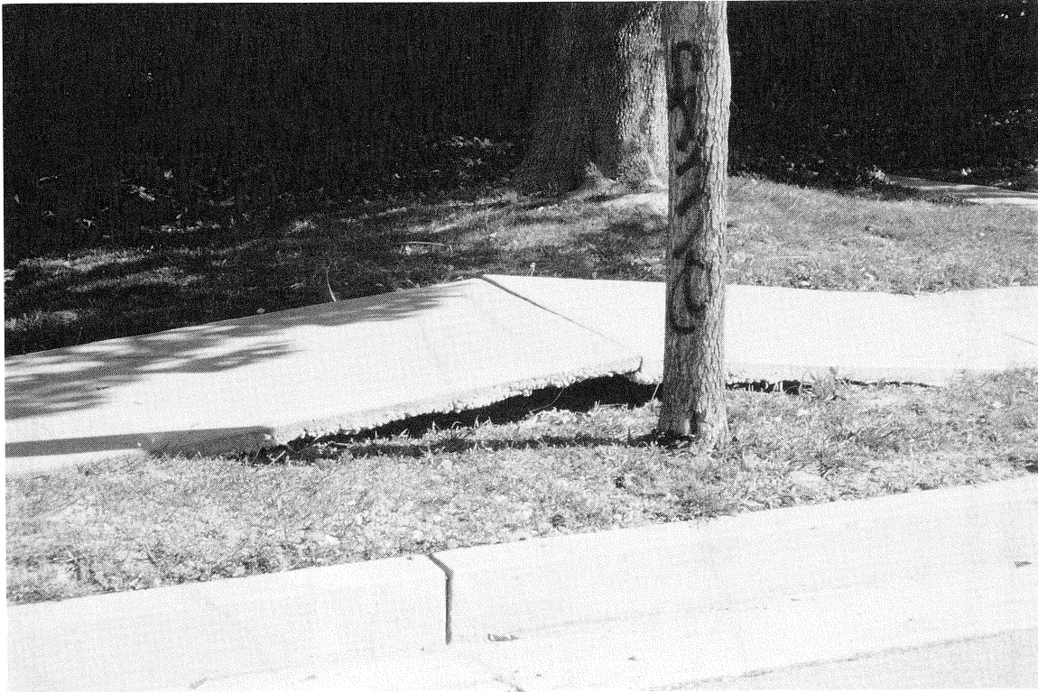
FIGURE 2-14 Compressive Ground Deformation Along Balboa Boulevard in Granada Hills
