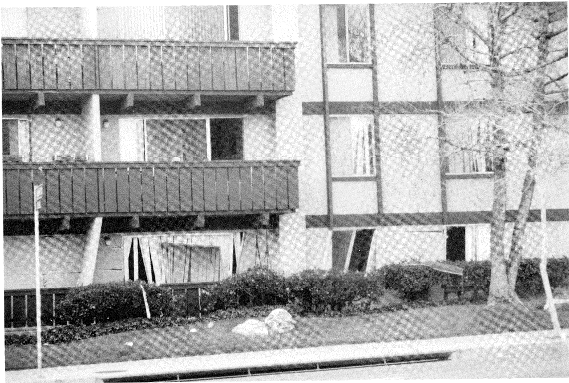
FIGURE 3-19 Lateral Deformations in the Ground Floor of Wood Frame Structure on Reseda Boulevard in Northridge
