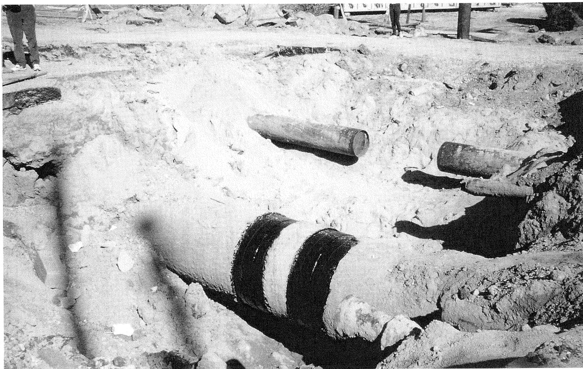
FIGURE 2-15 Section of the Water Main Along Balboa Boulevard that had to be Repaired After the Earthquake
