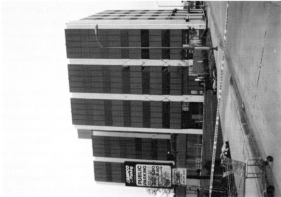
FIGURE 3-32 Nonsymmetric Moment Resisting Space Frame of Barrington Medical Building in Santa Monica
