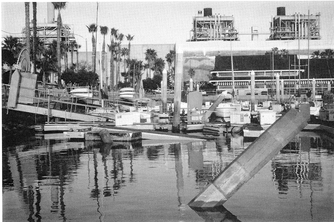
FIGURE 2-8 Tilting of the Mooring Piles at the Top of the Rock Berm of the Pier in Redondo Beach
