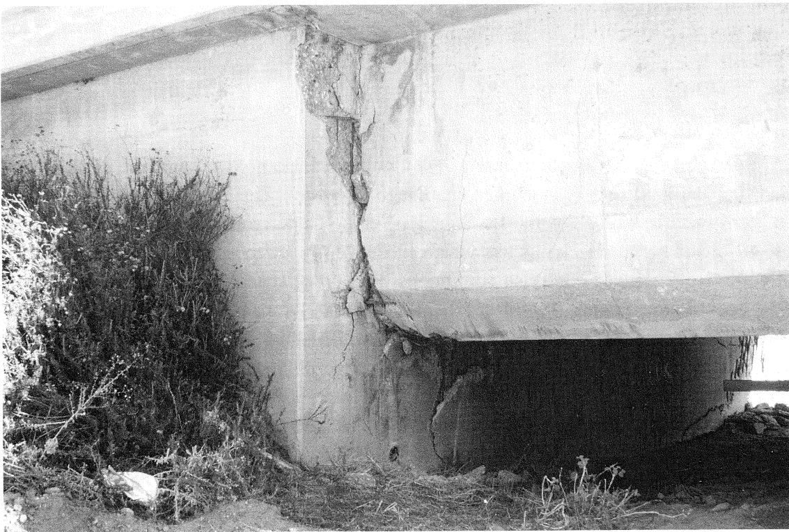
FIGURE 3-7 SR14/I-5 South Connector - Damage to Abutment 10
