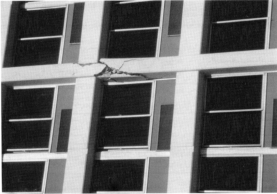
FIGURE 3-25 Damaged Columns in Seven-Story Hotel in Van Nuys
