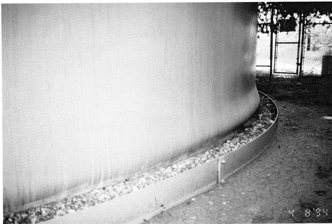
FIGURE 4-9 Elephant's Foot Buckling of Water Storage Tank in the Santa Clarita Valley
