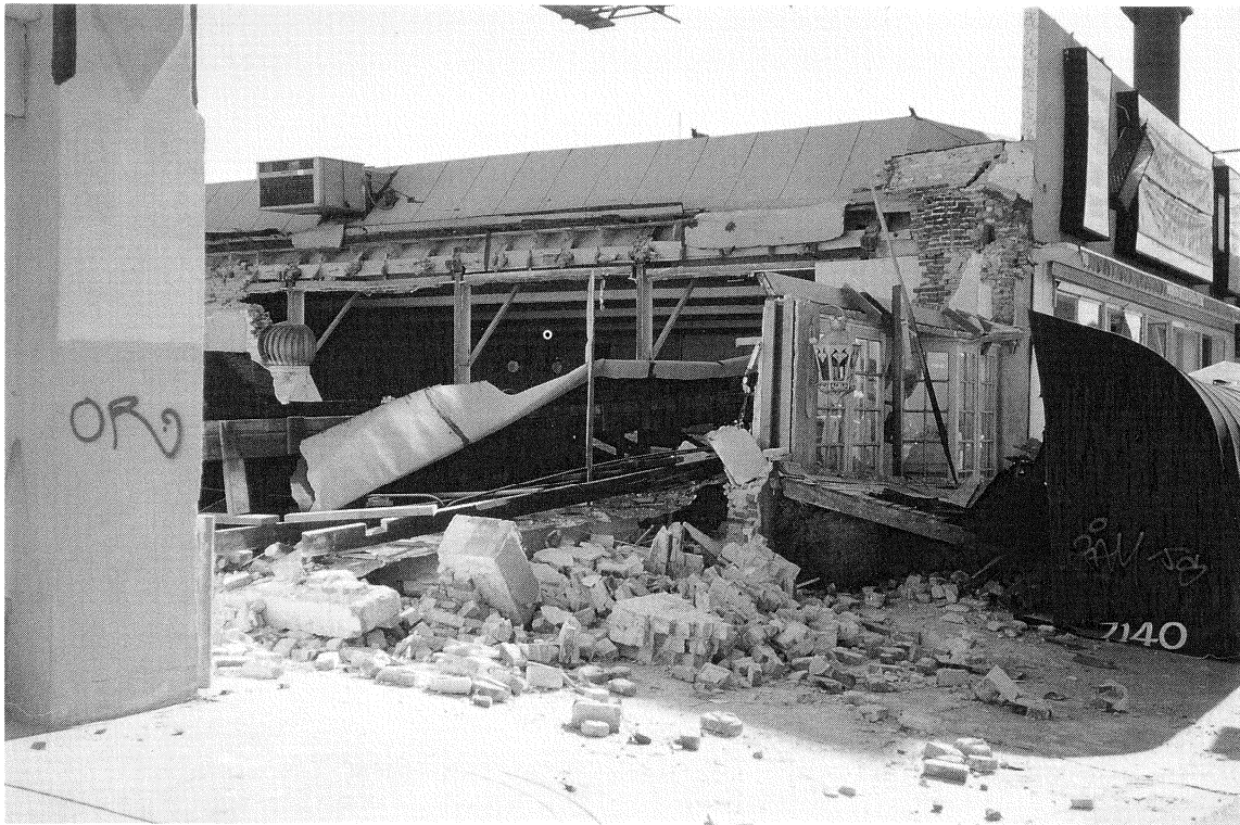
FIGURE 3-42 Collapse of Load Bearing Unreinforced Brick Masonry Wall and Roof in Northridge
