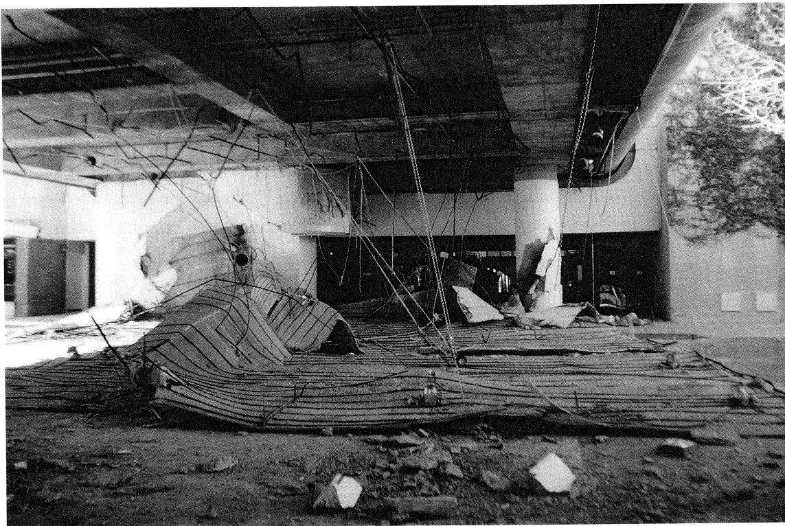
FIGURE 5-2 Stucco Breezeway Ceiling Detached from Concrete Frame at the Northridge Fashion Center
