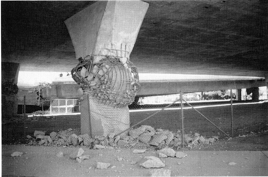
FIGURE 3-10 Mission-Gothic Undercrossing - Hinge Formation Below Flare in Column of Eastbound Bridge (Side View)
