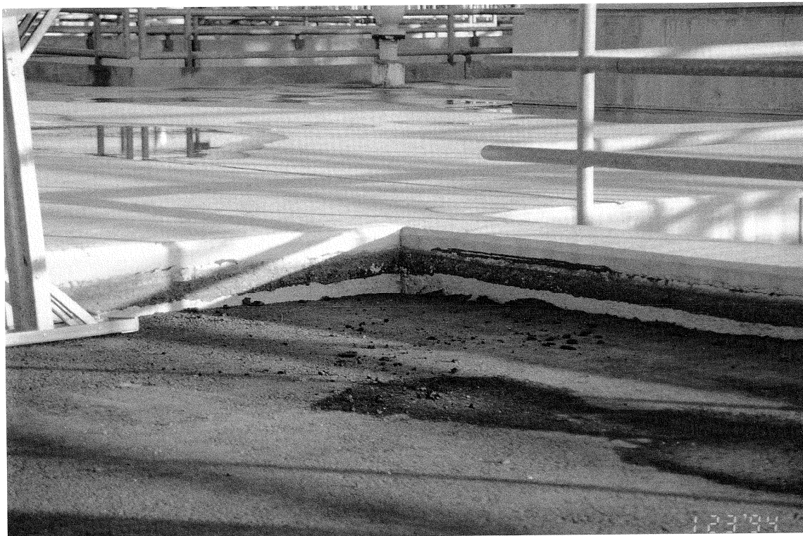
FIGURE 4-4 Typical Six to Eight Inch Settlement of Soils Adjacent to Concrete Basins at the 600-mgd Water Treatment Plant - Settlement Severed Several Buried Electrical Conduits and Chlorine Solution Lines
