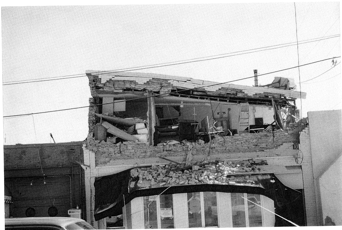
FIGURE 3-41 Collapse of Unreinforced Masonry Wall
