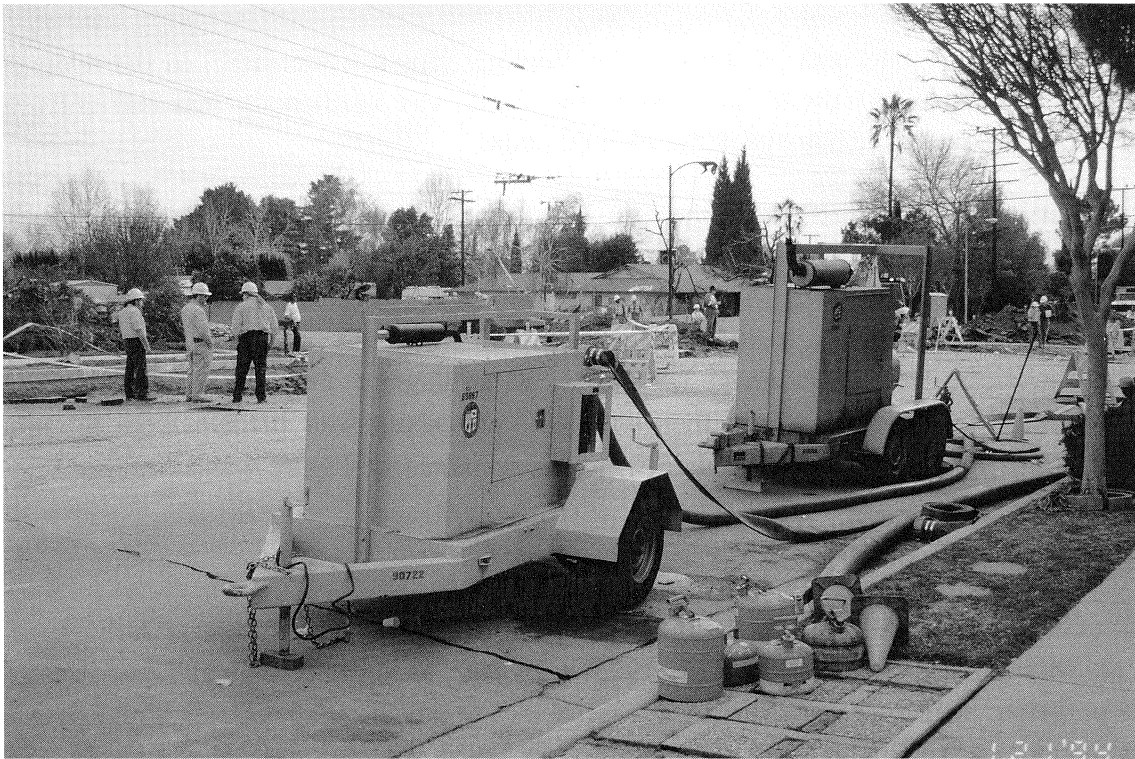
FIGURE 4-14 Portable Bypass Equipment (to Bypass Sewage Flow) Used in Support of Televised Inspection of Underground Sewer Lines
