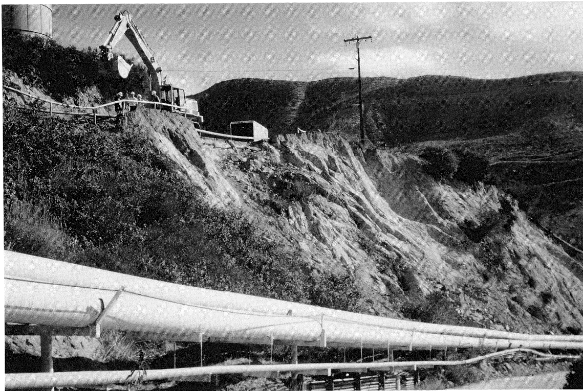
FIGURE 4-21 Local Landslide in Sandstone and Overlying Soil at the Aliso Canyon Gas Storage Facility
