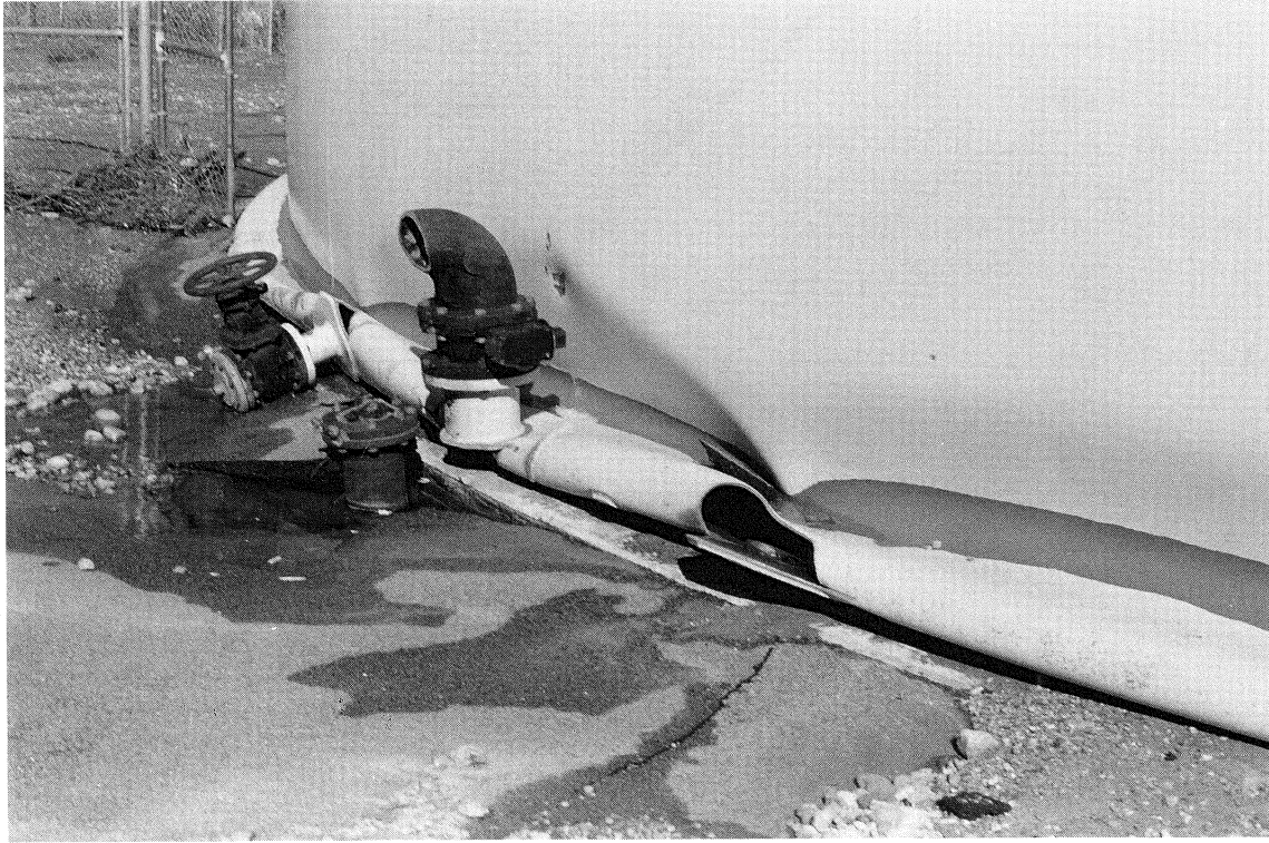
FIGURE 4-10 Damaged Welded Water Storage Tank in the Santa Clarita Valley - Rocking of Tank Caused Elephant's Foot Buckling at the Tank Base and Damaged Inlet and Outlet Lines
