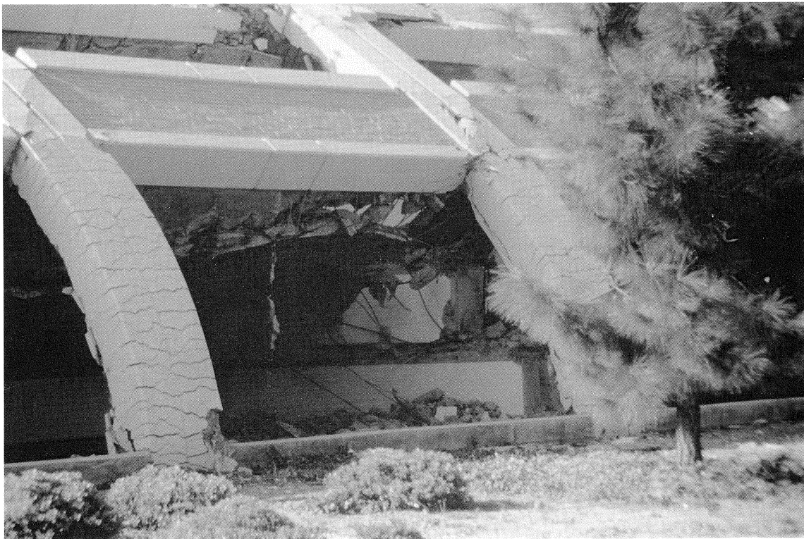
FIGURE 3-49 Curved Unbroken Columns in the Parking Garage at California State University, Northridge
