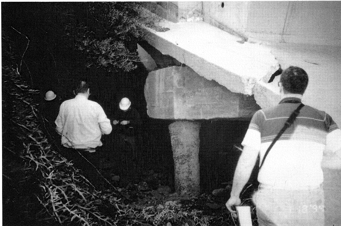
FIGURE 3-11 Balboa Boulevard Overcrossing - Soil Erosion at South Abutment Due to Ruptured Water Lines
