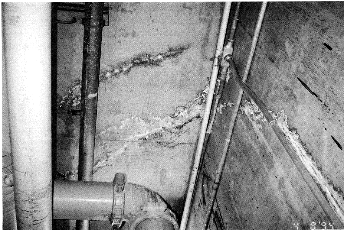
FIGURE 4-13 Repaired Cracks (by Epoxy Injection) in Concrete Basins of 15-mgd Wastewater Treatment Plant in the Santa Clarita Valley
