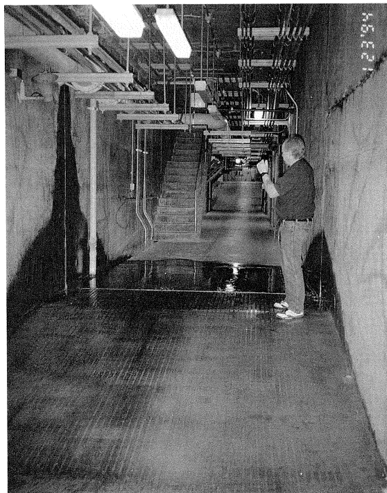
FIGURE 4-7 Utility Gallery in the 600-mgd Water Treatment Plant (Note water leaking out of cracks in concrete basin. Extensive cracking of concrete structures and basins was observed at this facility.)
