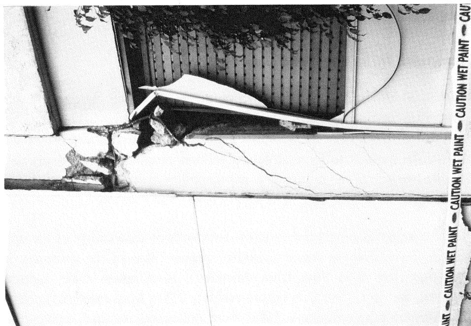
FIGURE 3-27 Column Shear Failure at First Floor of Hotel Building in Sherman Oaks
