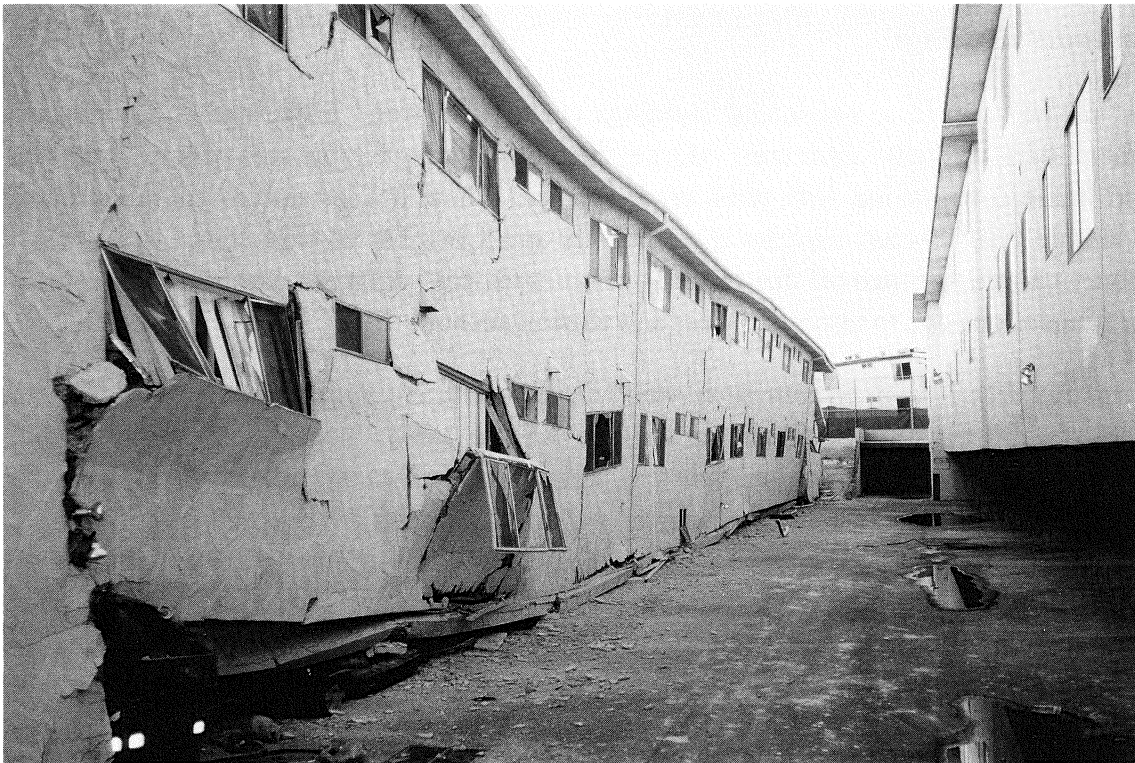
FIGURE 3-17 Wood Frame Apartment House with Collapsed Carport on Reseda Boulevard in Northridge
