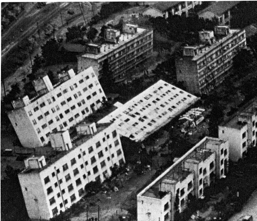
Figure 3: Liquefaction of the underlying soil resulted in the tilting and settlement of these Japanese apartment buildings after the 1964 Niigata earthquake.
