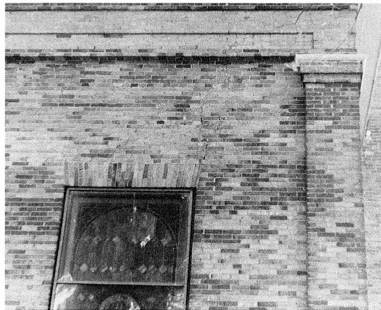
Figure 3: Baptist Church, Massena. Each photo shows where large cracks in unreinforced masonry caused by the 1944 earthquake were repaired.
