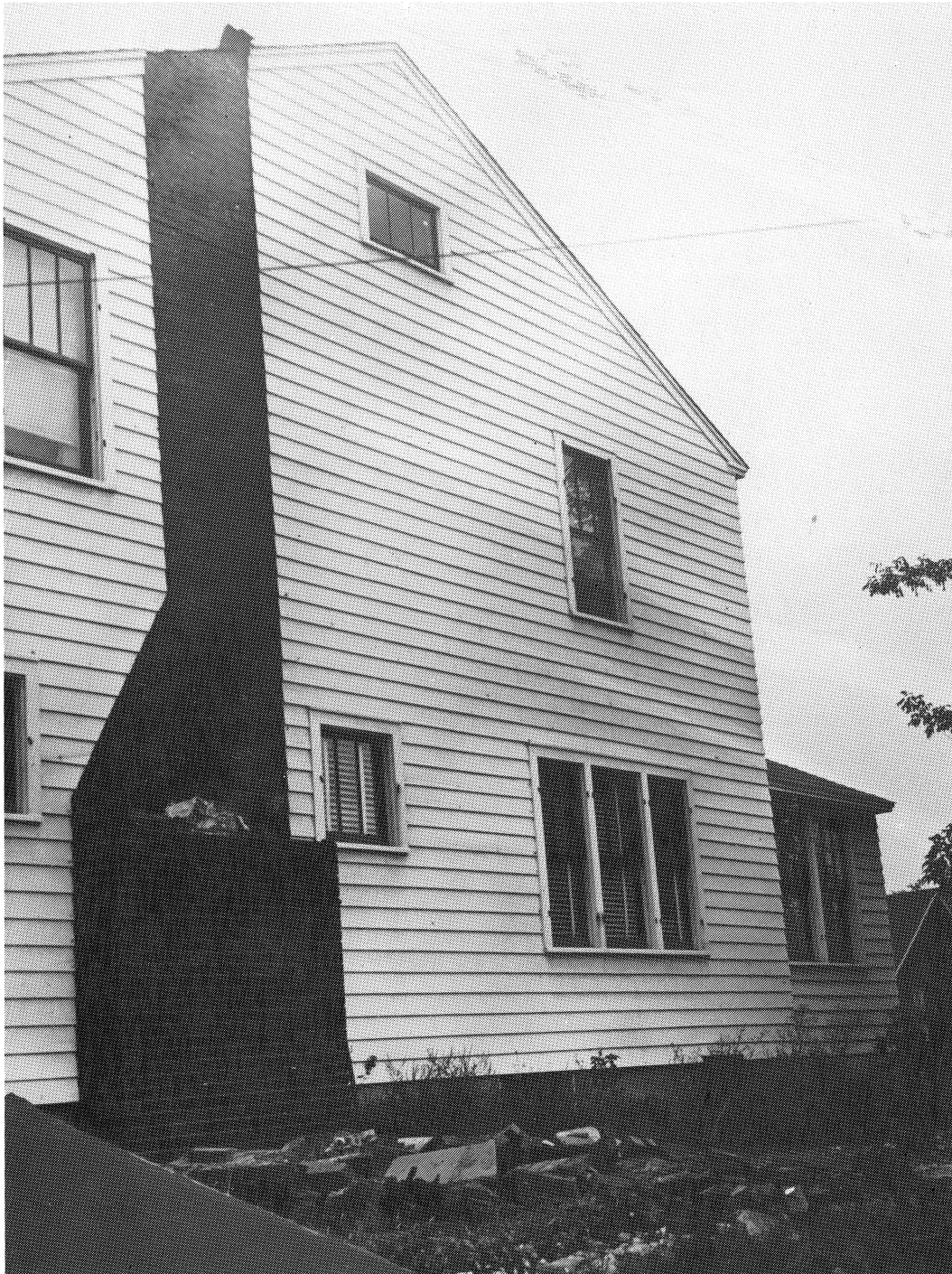
Figure 2: Currently, the only surviving photo of the 1944 earthquake damage is one of this chimney at the Nicola residence, 129 North Main Street. Over 90% of the chimneys in Massena were damaged or destroyed.
