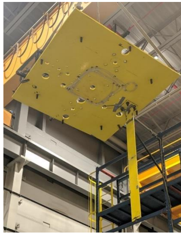
(a) steel plate internal attached to vessel head
