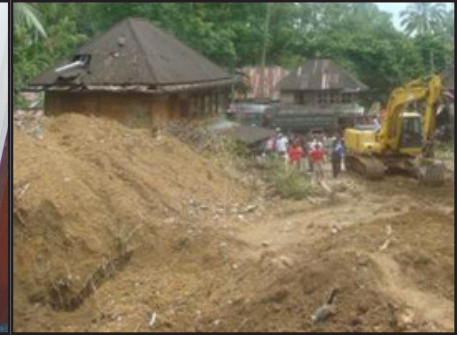
Figure 4. Landslide at Gunung Nan Tigo (Source: Indonesian Department of Education)
