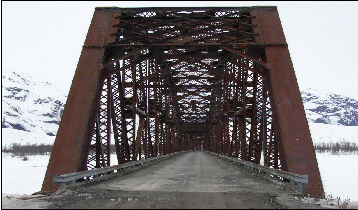
Figure 7-6. Million Dollar Bridge, Alaska, Portal Frame
