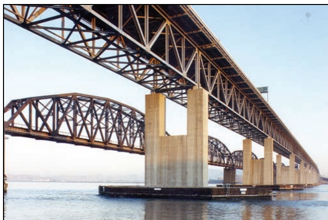
Figure 8-3. Benicia-Martinez Bridge, California, 1960; Gerber Framing, 528-ft truss Spans (1932 RR Camel-Back Truss in the Background)
