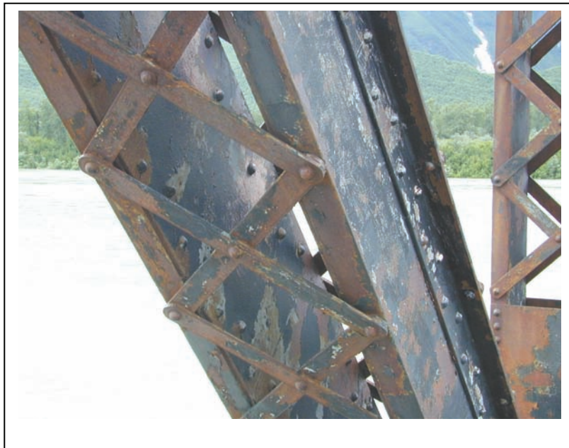
Figure 6-1. Typical Built-Up Member
