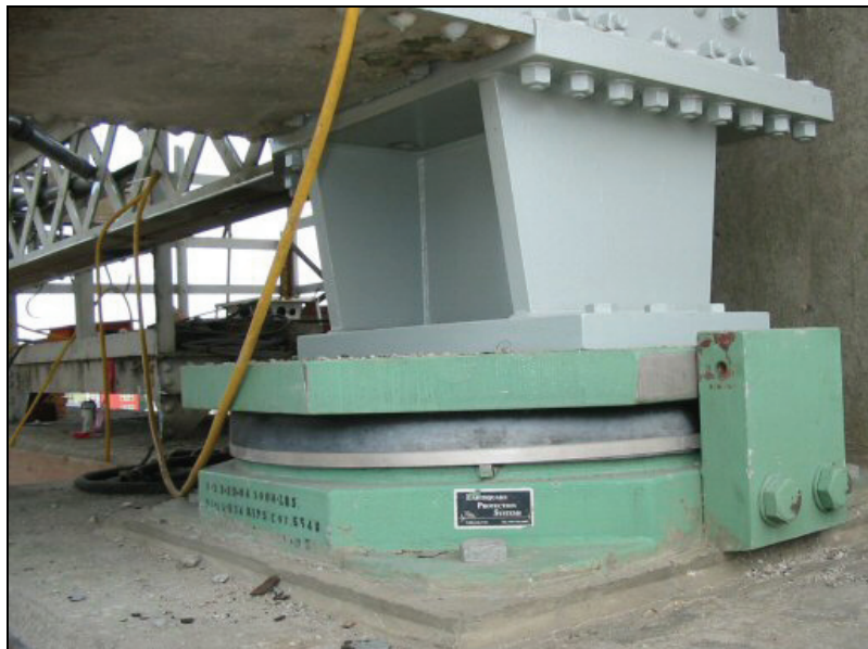
Figure 8-11. Friction Pendulum Bearing Installed
