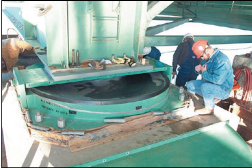
Figure 8-9. Installation of Friction Pendulum Bearing
