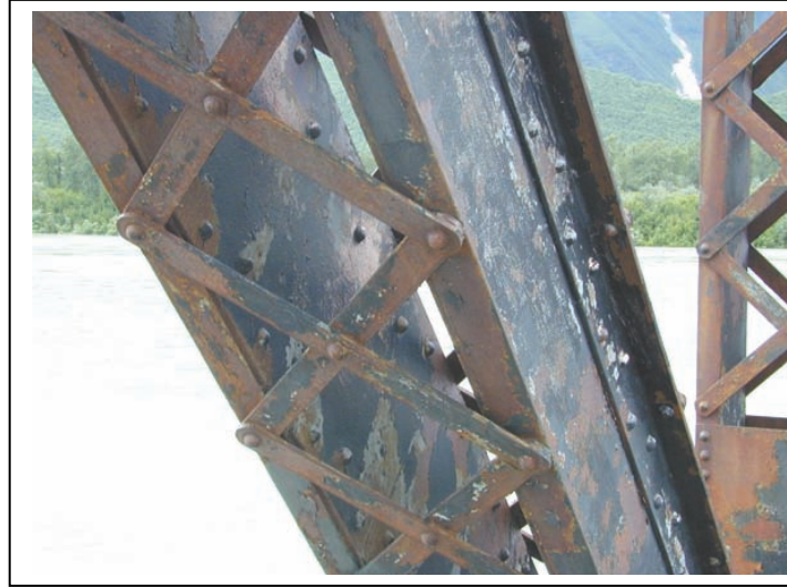
Figure 4-12. Typical Laced Member
