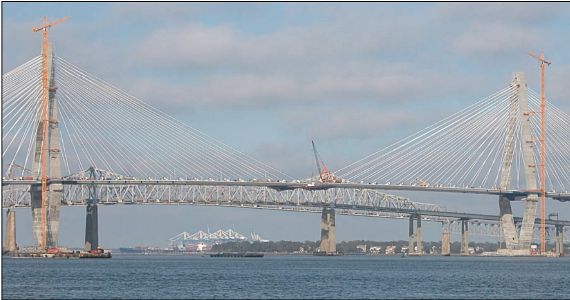
Figure 8-15. Replacement of the Cooper River Bridge, Charleston, South Carolina
