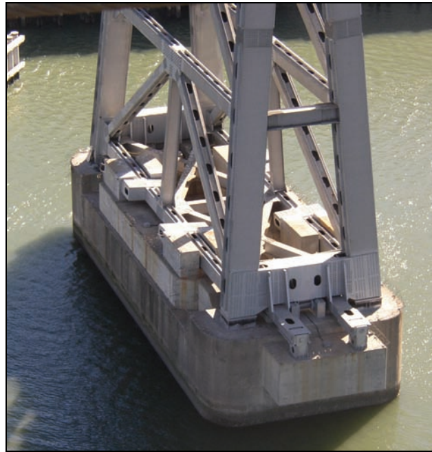
Figure 8-2. Seismic Retrofit of A-Frame Tower Rocking Supports
