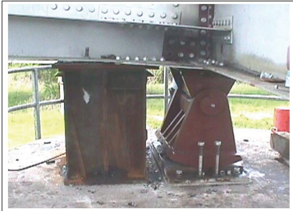
Figure 7-11. Rocker Bearing Replacement
