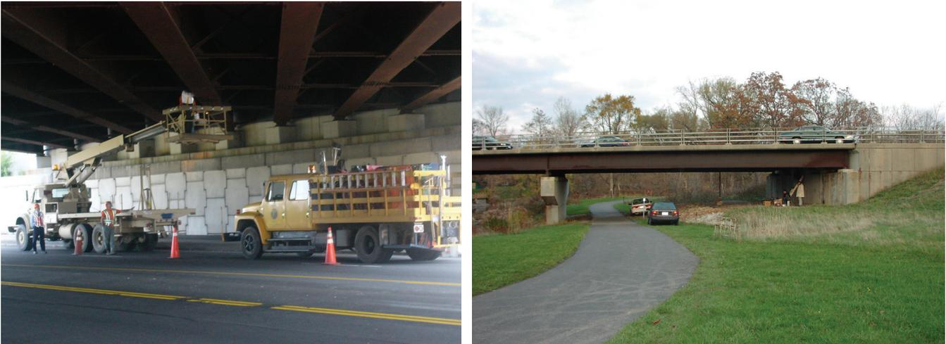
**Figure 3-8. (a) Sensor Installation Site for Condition Monitoring of the Intersection Bridge between the 990 Expressway and Sweet Home Rd., Amherst, New York; and (b) Data Collection Site of the Intersection Bridge between NY Highway 263 and Bikeway, Amherst, New York**
