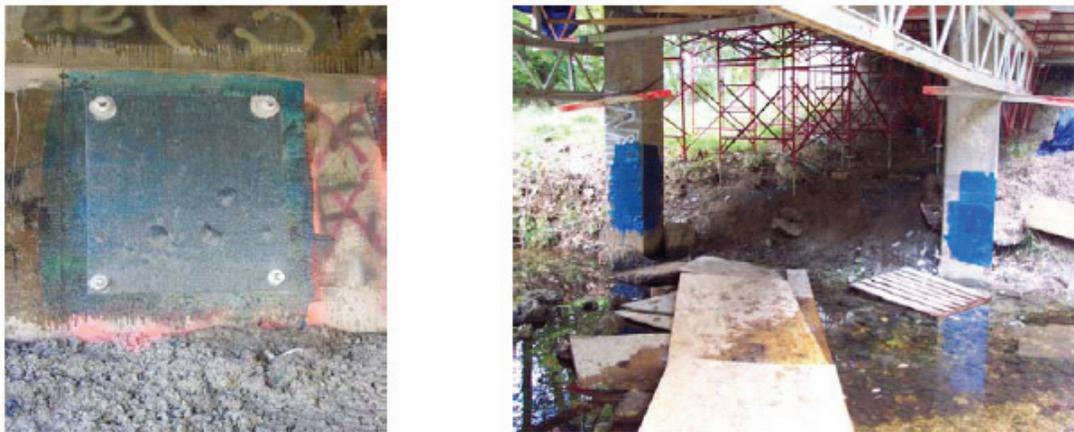
**Figure 4-13. CFRP Laminates with Delaminations on South Abutment and North Bent**
