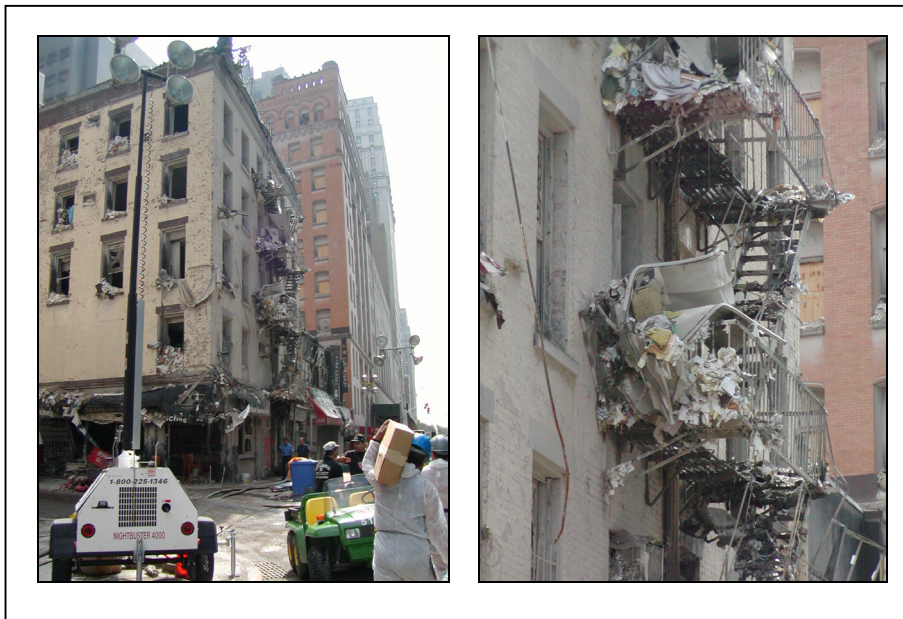
Figure 3.29. Debris in the emergency stairs of a small building near Ground Zero
