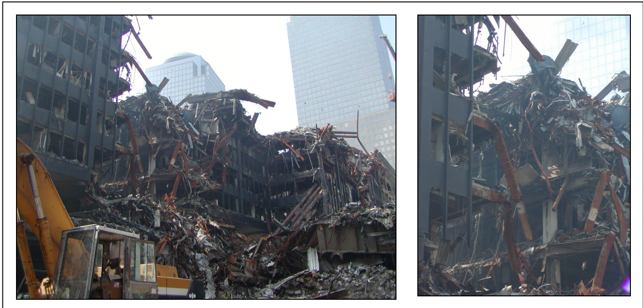
Figure 3.11. Impact and fire-related damage to WTC 6
