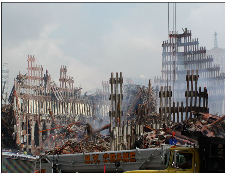
Figure 3.5. (continued). Portions of the perimeter tubes of WTC 1 and 2 that remained standing in the debris pile (as of September 21, 2001)
