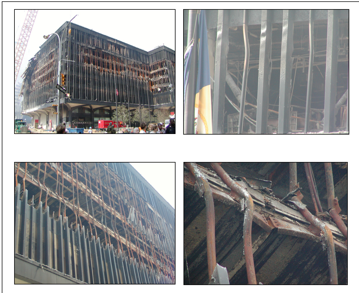
Figure 3.10. Fire related damage to WTC 5
