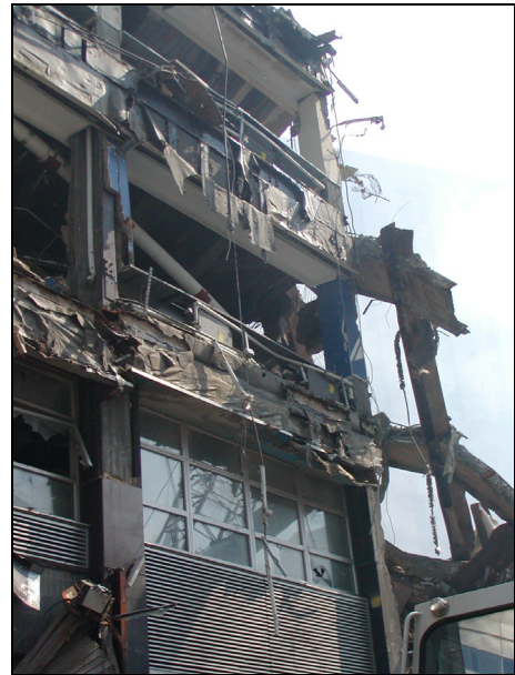
Figure 3.16 Damage to the west face of a building at 30 West Broadway due to impact from the collapse of WTC 7
