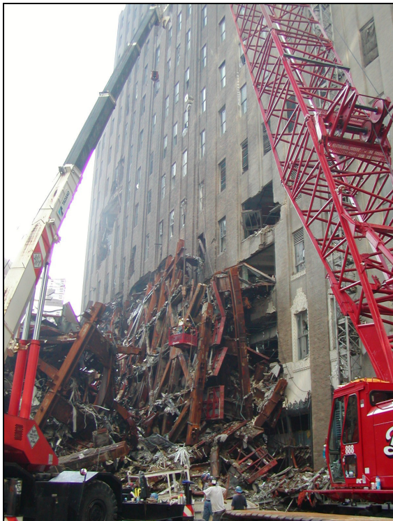
Figure 3.18. Damage to the west façade of the Verizon Building
