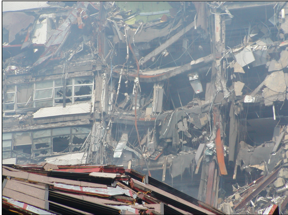
Figure 3.17. Beams in the building at 30 West Broadway were permanently distorted by the impact of falling debris
