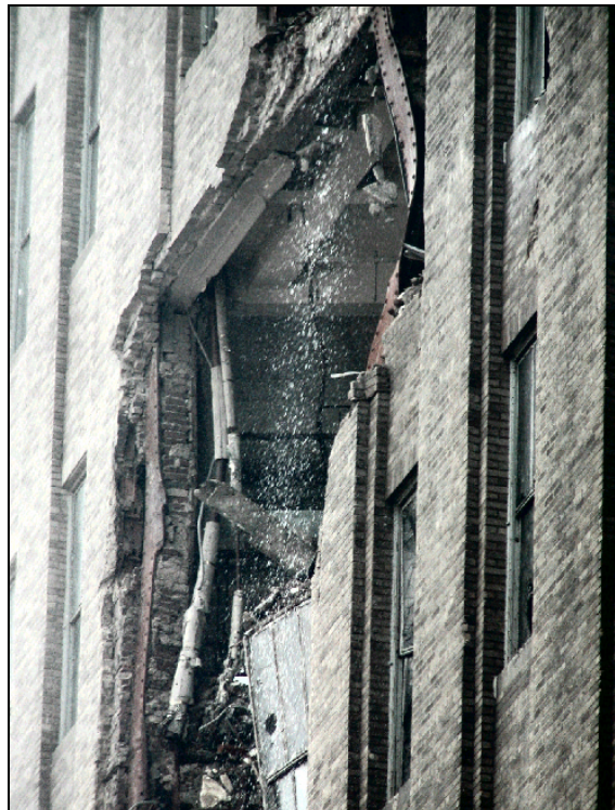
Figure 3.18. Damage to the west façade of the Verizon Building
