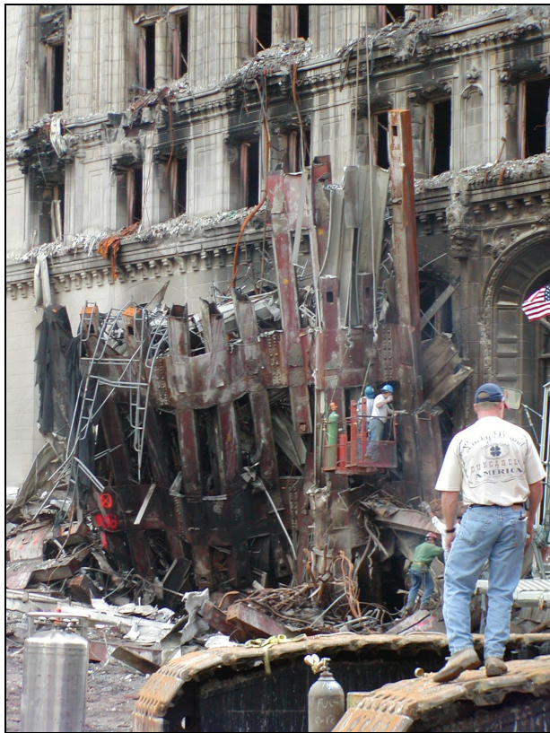
Figure 3.23. Large multi-ton segment of the façade of the WTC 2 lodged at base of the 90 West Street building
