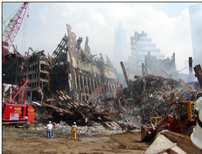
Figure 3.5. Portions of the perimeter tubes of WTC 1 and 2 remained standing in the debris pile (as of September 21, 2001)
