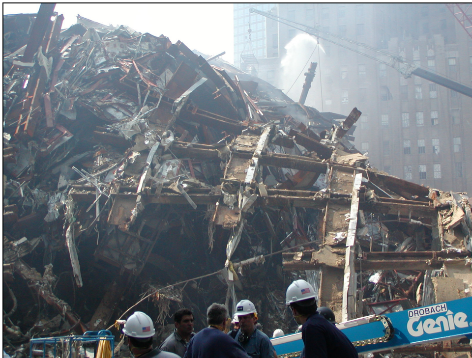
Figure 3.13. Portions of conventional steel moment-resisting frames were observed in the debris pile
