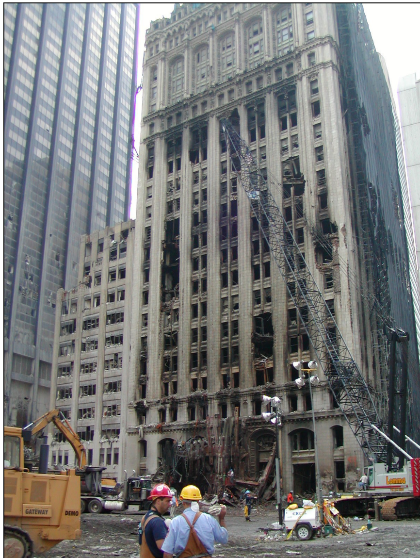
Figure 3.22. 90 West Street building
