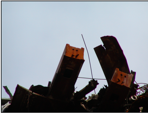
Figure 3.7. Typical four-bolt column splices and access holes on the side of hollow rectangular columns
