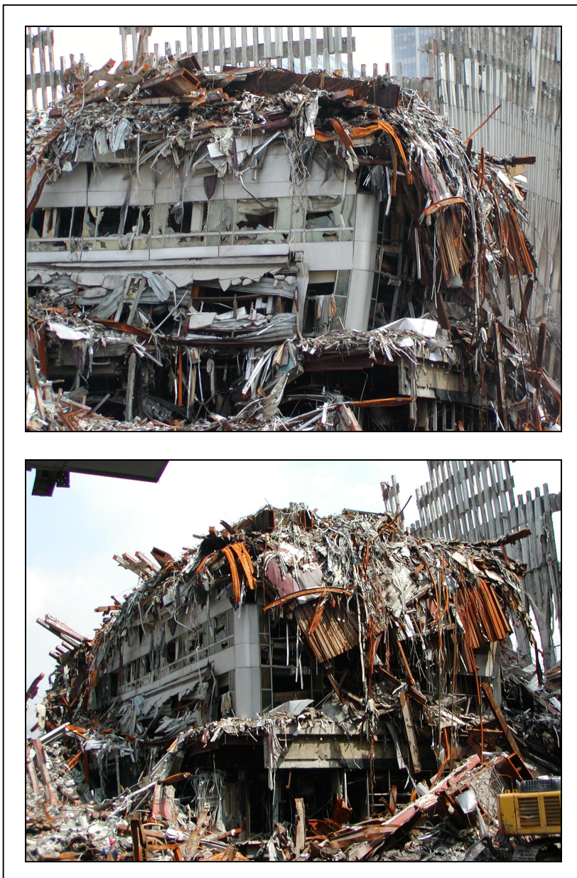
Figure 3.8. Debris falling destroyed WTC 3
