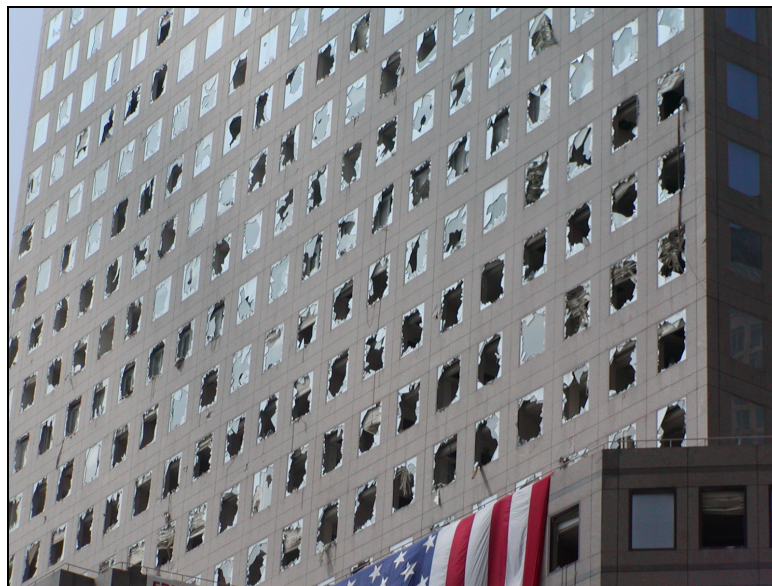
Figure 3.27. Broken windows in 2 World Financial Center
