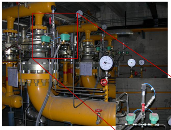
Fig. 15. Flow dividers installed in a M/R station
