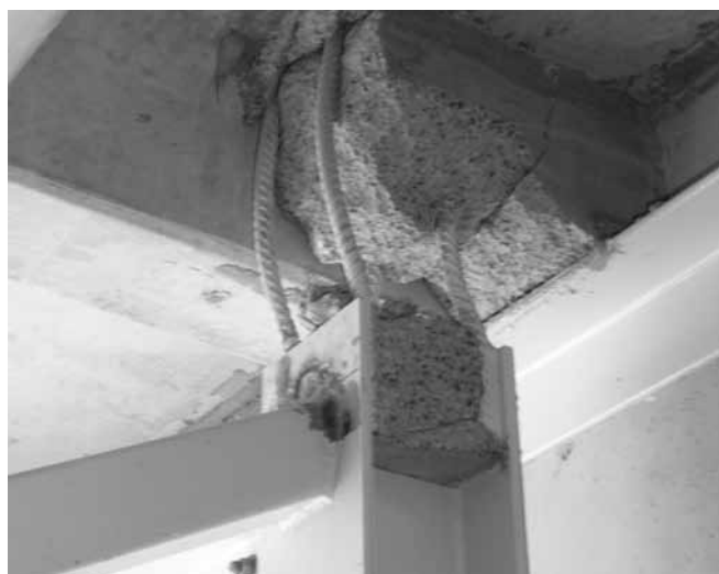
(a) Poor column connection detail
