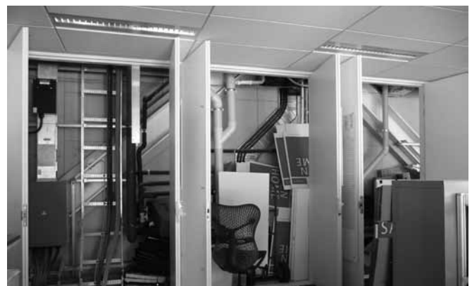
d) Global view of EBF braces obstructed by various utility runs
