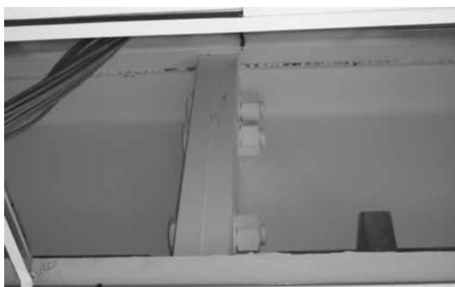
(b) Flush moment endplate splice connection
