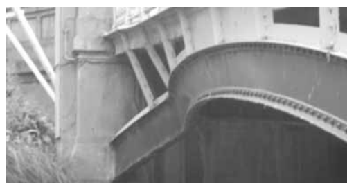
(b) Buckling of fascia arches
