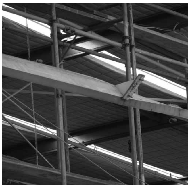
(b) Close-up view of fractures connection
