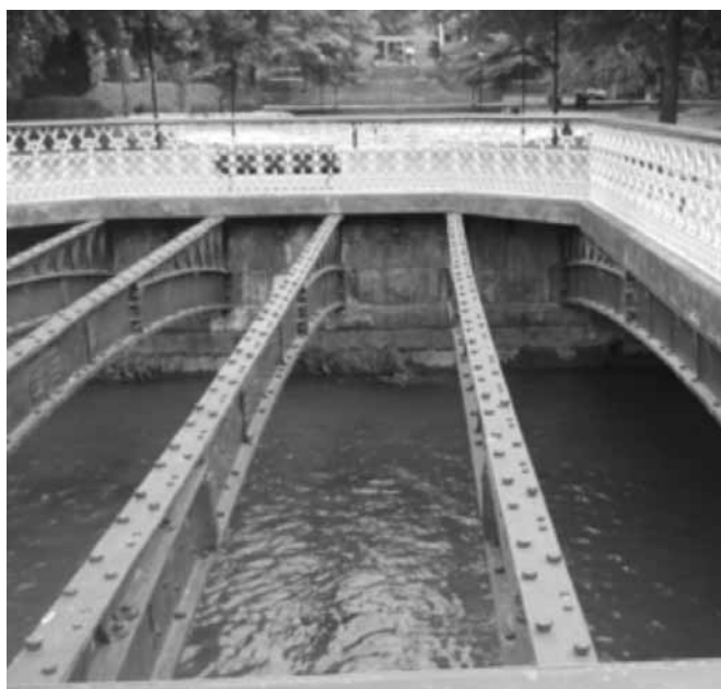
Figure 20 – Undamaged older steel pedestrian bridges on the Avon River near the CBD (Leon)
