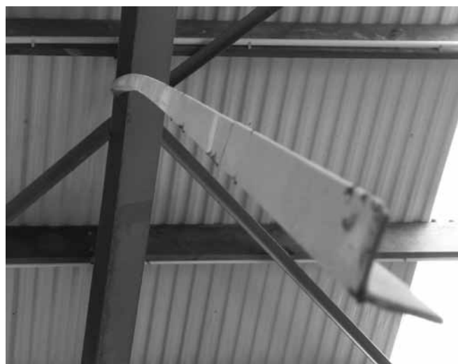
(b) Close-up view of fractures weld of tension brace
