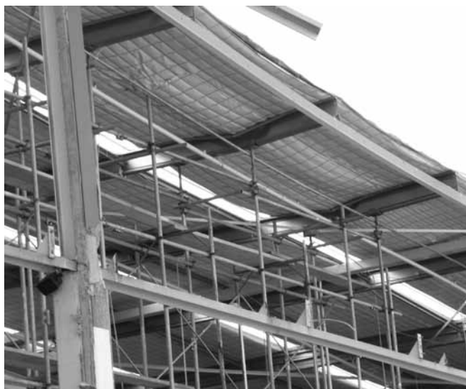
(c) Global view of buckled beams
