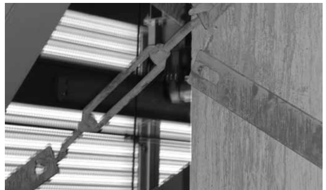
(b) and (c) Multistorey mechanical garage failed braces
