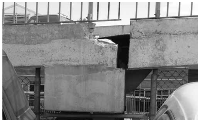
(f) Displacement at expansion joint, top ramp
