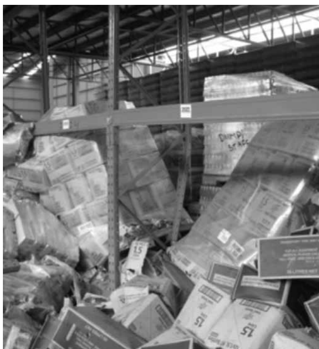
Figure 13: Example of collapsed industrial storage racks [Photos by M. Bruneau and G C Clifton]
