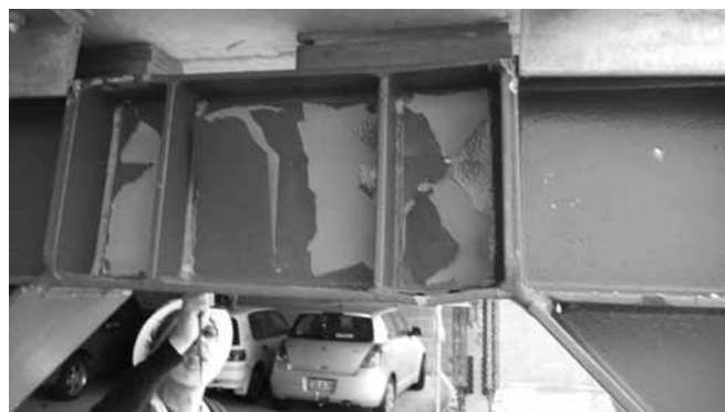
(d) Evidence of inelastic deformations at top level EBF
