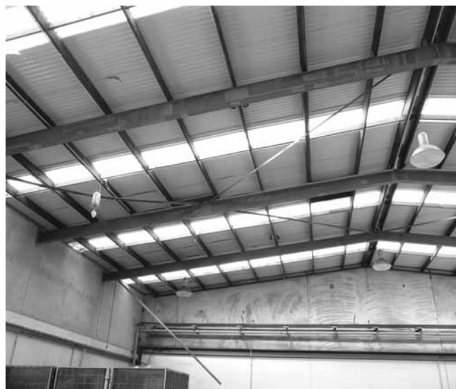
(a) Global view, showing buckled brace and fractured brace
