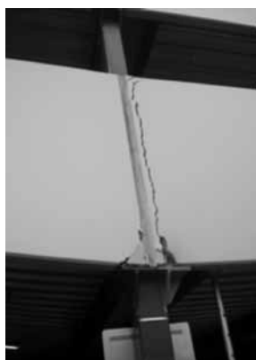
(b) Fracture of precast spandrel beams on south side
