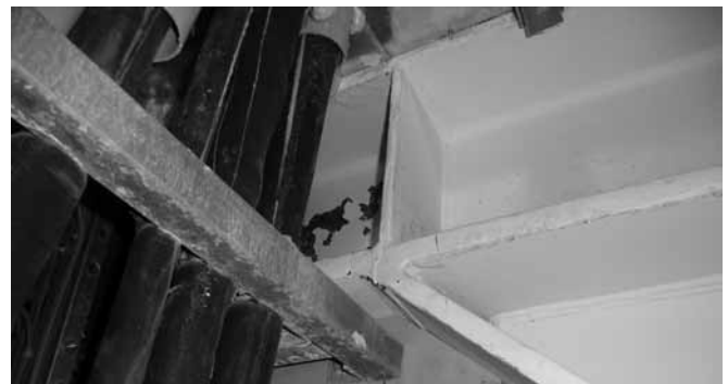
c) Paint flaking of partially hidden EBF link
