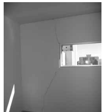
b) Cracking of partition in cantilevering portion of story
