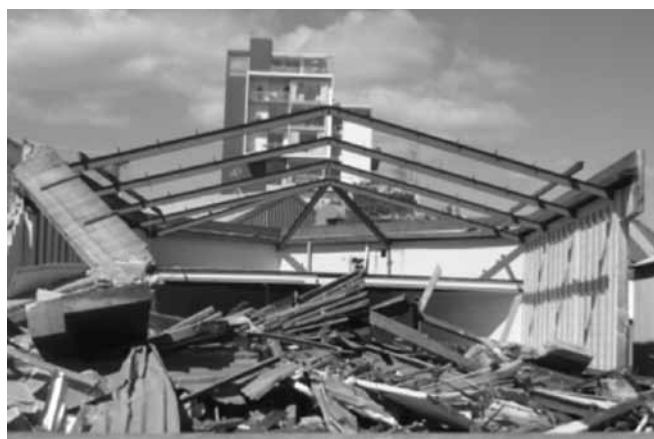
Figure 17 : Failure of roof and walls in older industrial facility on Salisbury Street [Photos by G. MacRae]
