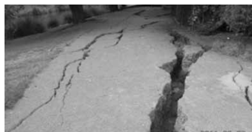
(a) Slumping of riverbank close to bridge
