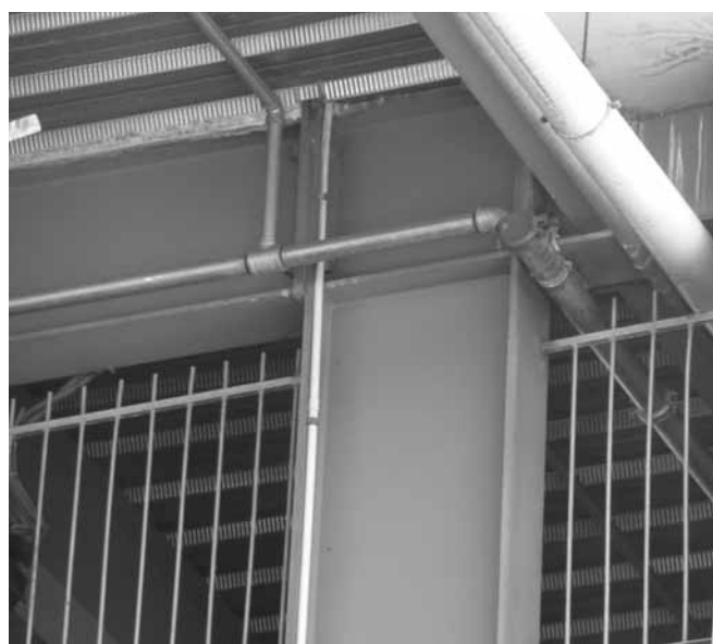
(b) Typical moment connections
