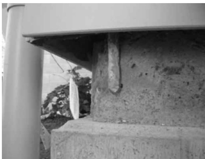
(b) Baseplate bolt at SE corner of the building
