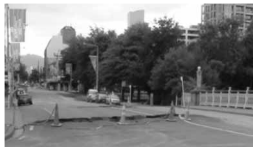
(c) Slumping of abutments at end of bridge
