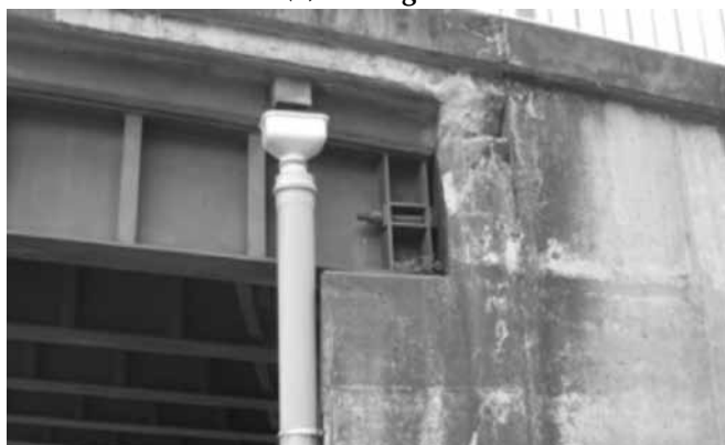
(b) Abutment spalling
