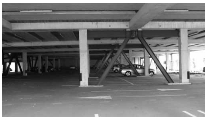
(a) Redundancy provided by multiple EBF bays
