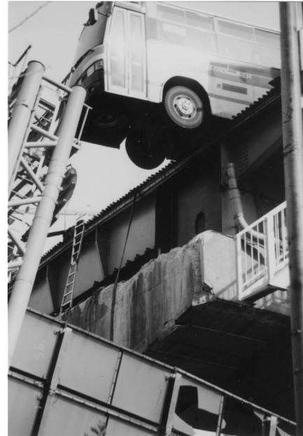
Figure 14 Example of collapsed span as a result of insufficient support length: (a) global view; (b) close-up view of top pier
