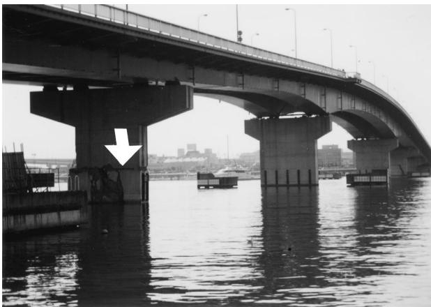
Figure 5 Sliding failure along construction joint of reinforced concrete pier supporting a steel superstructure (first pier on left of photo)
