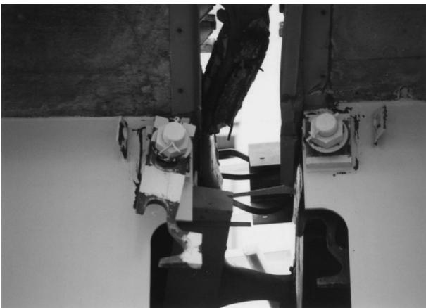
Figure 13 Example of unsatisfactory seismic restrainer behaviour
