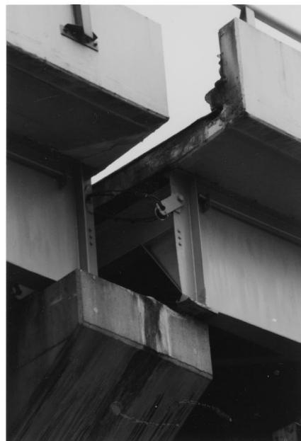
Figure 16 Examples of severe bearing damage: (a) near-collapse of span due to bearing keeper-plate failure; (b) near-collapse of span due to sliding in transverse direction following bearing failure
