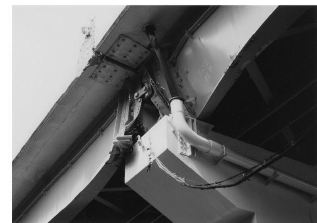
Figure 17 Severe lateral-bending of steel girders as a result of bearing failure in the transverse direction
