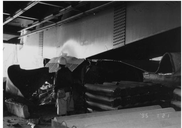
Figure 6 Example of collapse as a result of steel pier failure: (a) failed pier; (b) close-up view of split steel plates
