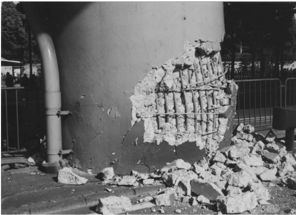
Figure 4 Two examples of flexural failure due to lack of confinement at bottom of reinforced concrete piers supporting a steel superstructure
