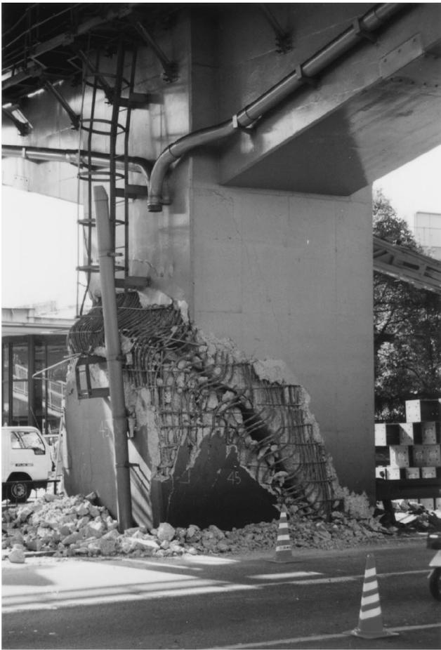
Figure 2 Shear failure at bottom of reinforced concrete pier supporting a steel superstructure
