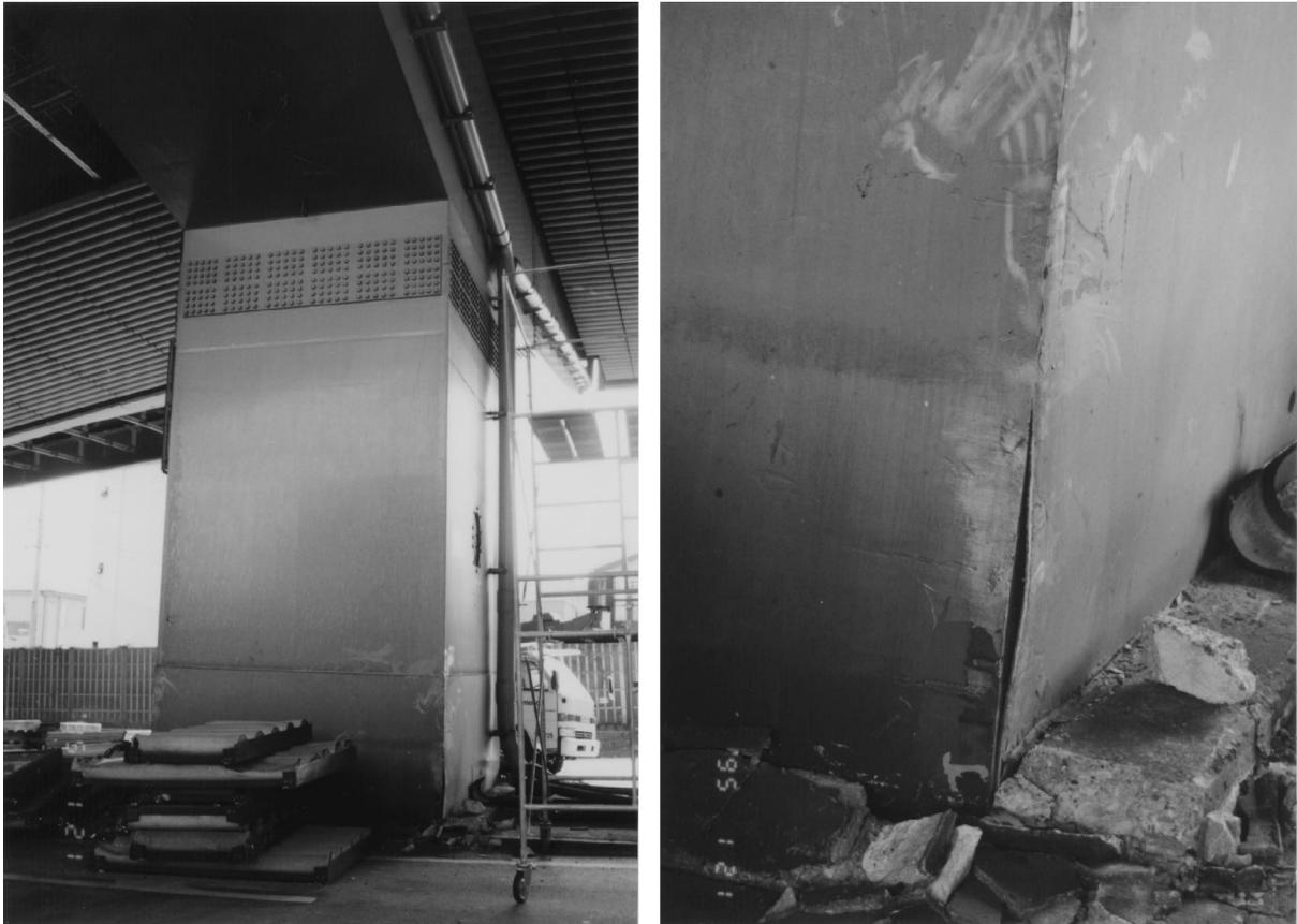
Figure 7 Condition of steel pier at other end of collapsed span: (a) global view of pier; (b) close-up view of failure of a weld-seam at bottom corner of box-column
