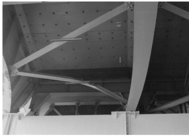
Figure 18 Failure of connection between end-diaphragm and steel girder
