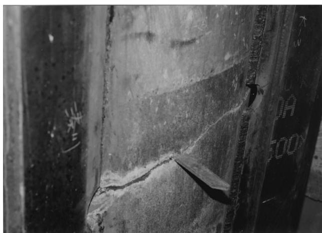
Figure 10 Brittle fracture in steel pier: (a) global view of pier (tall truss-towers) are emergency temporary span supports); (b) crack in steel plate, wide enough to permit insertion of a small steel plate (large steel plate stiffeners are temporary repairs)
