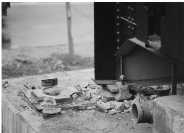
Figure 15 Example of damaged bearing and collapsed span: (a) global view, looking at the West direction; (b) close-up view of bearing damage, looking at the North-East direction (almost reversed view)
