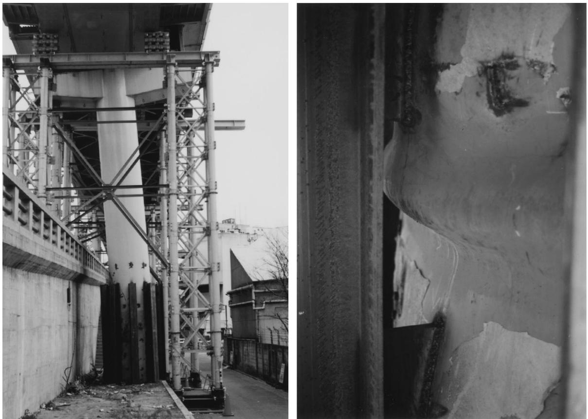
Figure 8 Severe buckling of circular hollow steel pier: (a) leaning pier as a result of buckling near base (steel plates stiffeners there are temporary repair measures, and tall truss towers are temporary span supports); (b) close-up view of severe buckling
