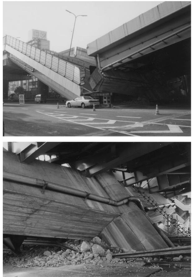
*Figure 1* Example of non-ductile reinforced concrete substructure supporting a steel superstructure: (a) span collapse; (b) close-up of fatal damage to non-ductile pier
