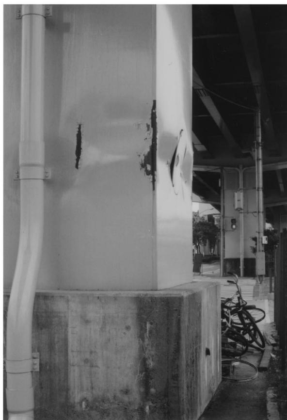
Figure 9 Examples of buckling in rectangular hollow steel piers: (a) mild buckling at pier base; (b) severe buckling at pier base; (c) buckling at the discontinuity created by door-hatches in steel pier
