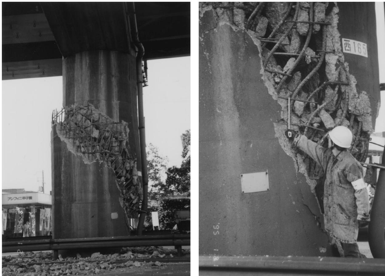
Figure 3 Shear failure at middle of reinforced concrete pier supporting a steel superstructure: (a) global view; (b) close-up showing large spacing of transverse reinforcement
