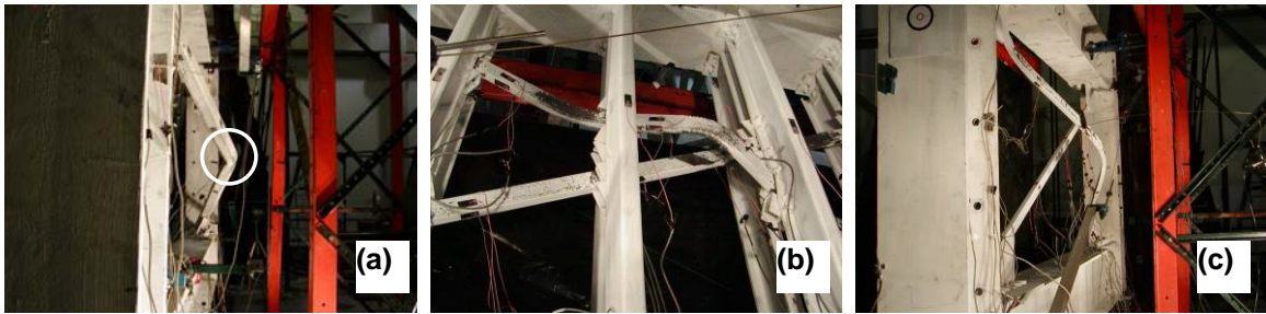
Figure 6: Damage level in specimens: (a) F2 ( -5\delta_y , Cycle 21); (b) F3 ( -4\delta_y , Cycle 19); (c) F4 ( -4\delta_y , Cycle 19)
