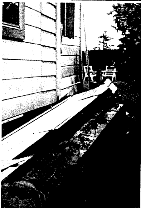
FIG. 17. Older residential structure on "pony-walls," not properly connected to its foundation (Hollister).
