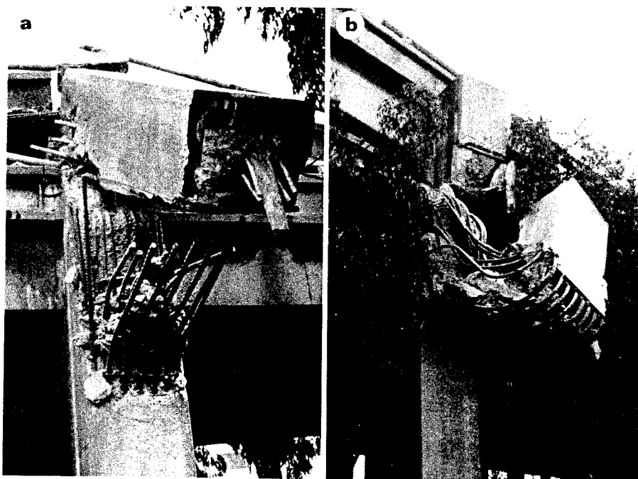
FIG. 8. Typical joint failure at (a) base of hinged upper column and (b) base of continuous upper column.
