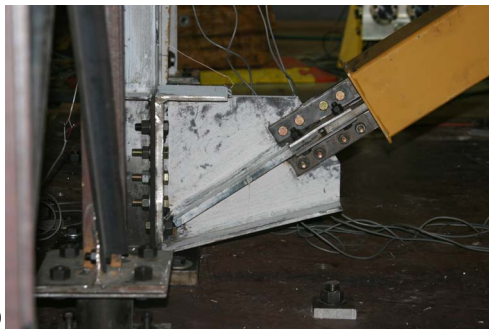
Fig. 8. BRB-to-column connection detail (a) as designed; (b) after setup (only on bottom story)
