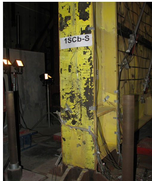
Photo 6 Column flange yielding
