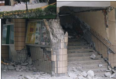
Figures 1 and 2. Failure of non-ductile details.
