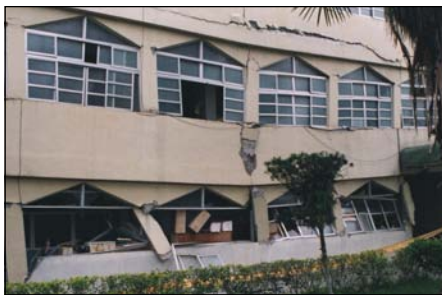
Figures 1 and 2. Failure of non-ductile details.
