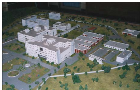
Figure 3. An overview model of the Veterans Hospital in Puli. The two white buildings are the newest and both sustained considerable damage.
