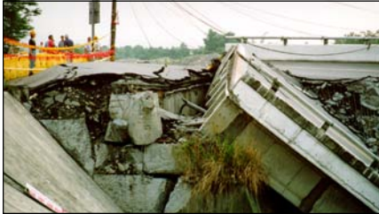
Figure 2 (below). Failure of the back-wall of the south abutment of the Ming-tsu bridge (Route 3), leading to the unseating of adjacent spans. Figure 3 (right). Shear crack in Pier 1 of the Wu-shi bridge (Route 3).
