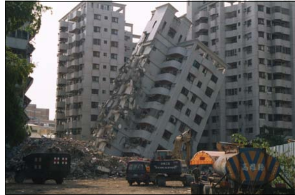
Figure 3. Failure of new construction.
