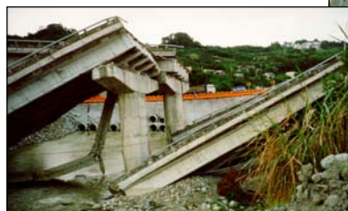
Figure 4 (right). Rigid-body rotation of Pier 10 due to ground failure under the E-jian bridge (Route 129). Figure 5 (below). Tilting of Pier 2 and subsequent collapse of three spans of the Shi-wei bridge (Route 3).
