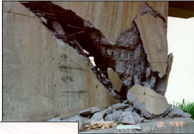
Figure 2 (below). Failure of the back-wall of the south abutment of the Ming-tsu bridge (Route 3), leading to the unseating of adjacent spans. Figure 3 (right). Shear crack in Pier 1 of the Wu-shi bridge (Route 3).
