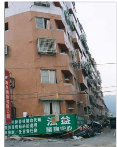
Figure 4. Failure due to soft first story.
