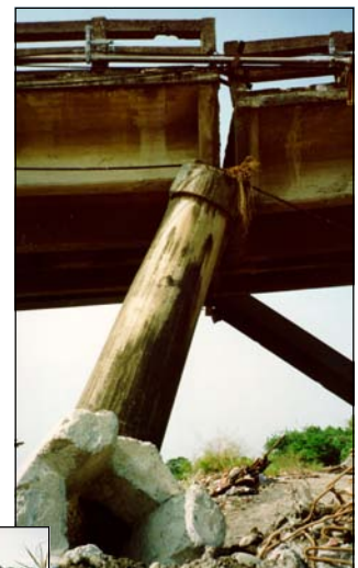
Figure 4 (right). Rigid-body rotation of Pier 10 due to ground failure under the E-jian bridge (Route 129). Figure 5 (below). Tilting of Pier 2 and subsequent collapse of three spans of the Shi-wei bridge (Route 3).
