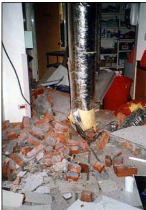
Figure 5. Interior damage in the Shiu-Tuan Hospital. Shown are (top) fallen brick inside the hospital and (right) a damaged interior glass brick wall.
