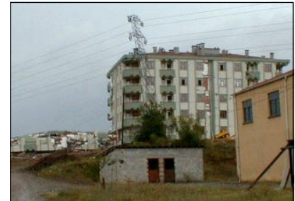
Figure 1. Electric transmission tower pulled to left due to conductors being put in tension due to right lateral fault displacement (fault is to north, or left, of the tower).
