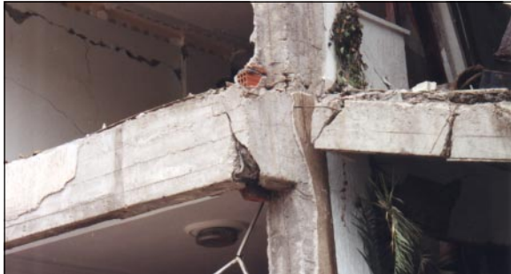
Figure 3. Eccentric beam to column connections induced severe torsion in short perpendicular stub beams.
