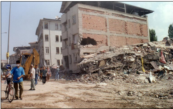
Many residential buildings were severely damaged.
