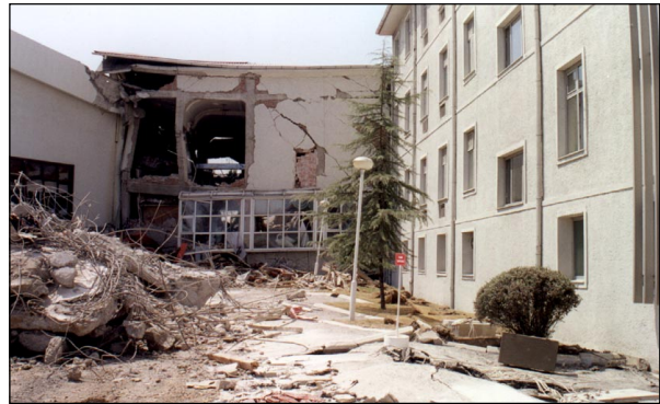
One building is totally collapsed while another is hardly damaged on the Naval Base in Golcuk.
