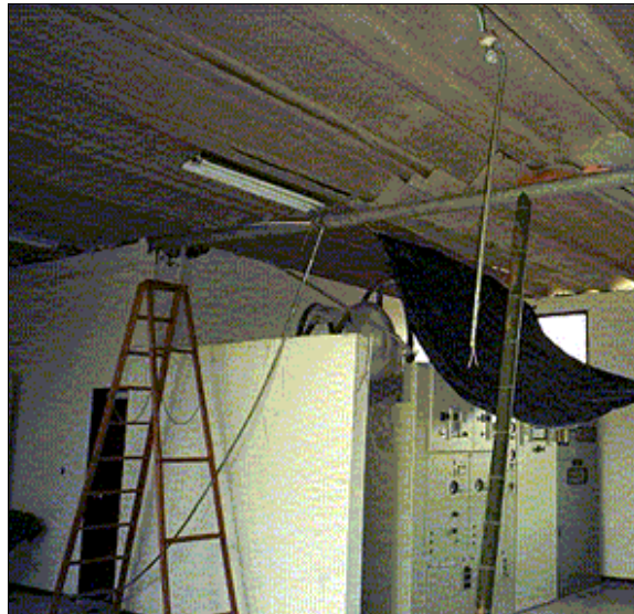
Figure 4-2 Substation Sur (33 kv/13.2 kv, 15 mva, 1982) in Armenia: Roof Control Room Almost Collapsed Due to Truss Failure, Temporary Support
