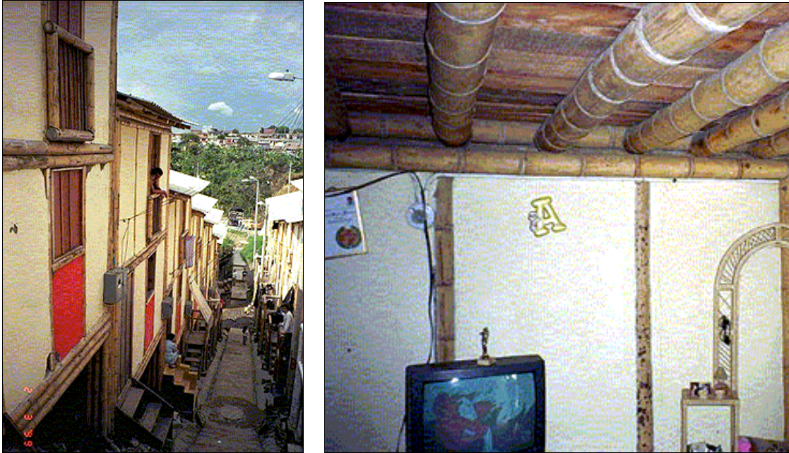
Figure 3-11 Miraflores Neighborhood, Armenia: 73 Houses Built with Guadua Frames, No Damage
