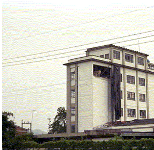
Figure 4-10 Industrial Building in Dos Quebradas was Damaged and Repaired in 1995, Suffered Damage in Nonstructural Panels and Some Deep Beams
