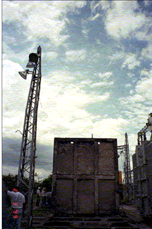
Figure 4-1 Substation Regivit (115 kv/33 kv, 60 mva, 1960) in Armenia: Damage on Tower Due to Transformer Fall
