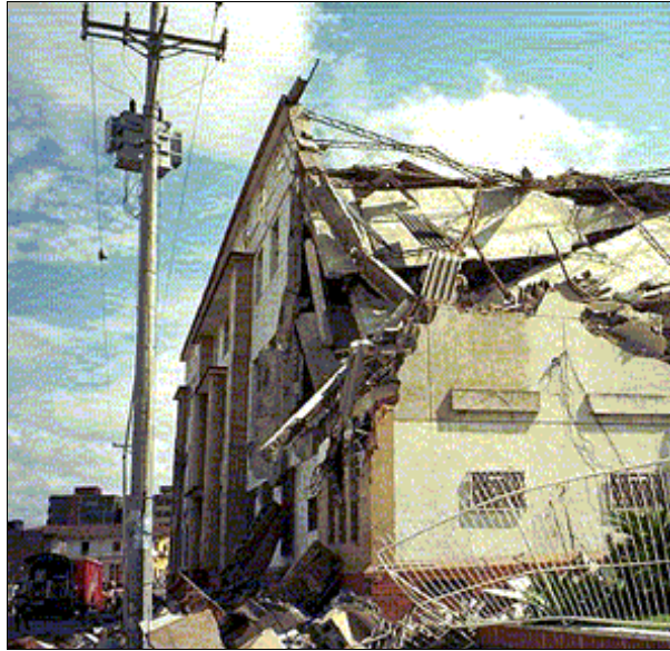
Figure 3-14 Damage to San Francisco Solano School in Armenia. URM Building
