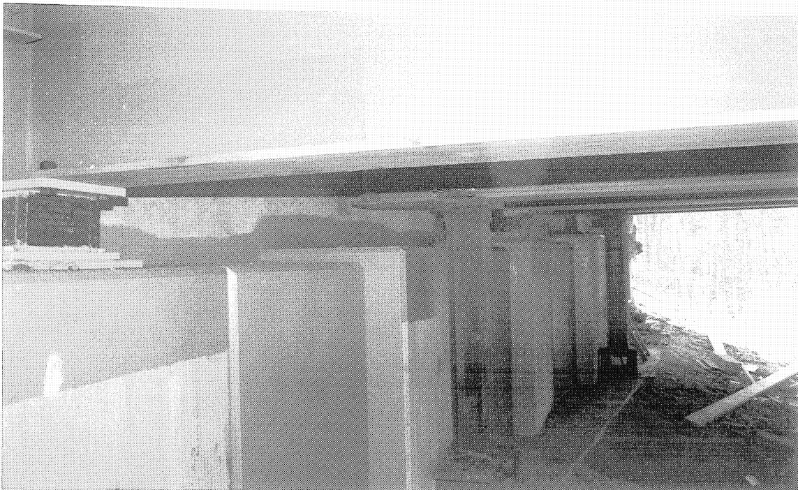
(b) Bearing Installation Procedure at the Abutment
