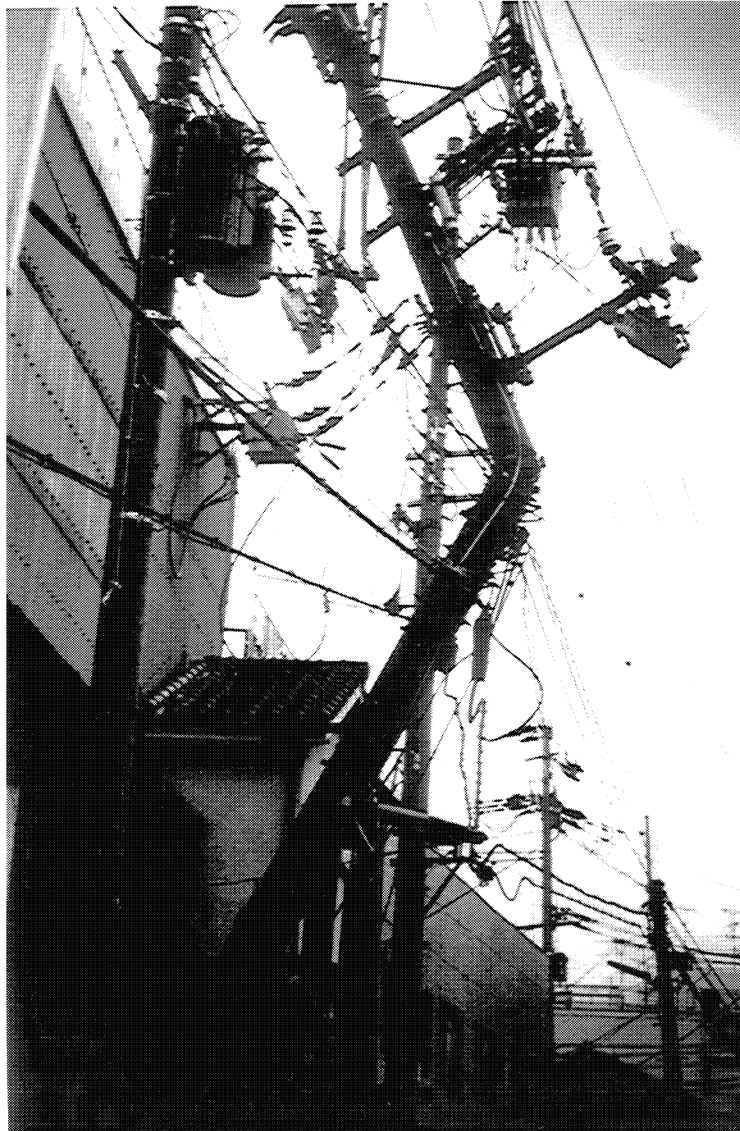
Figure 24 This concrete power pole failed due to induced vibrations in Kobe, Japan earthquake.
