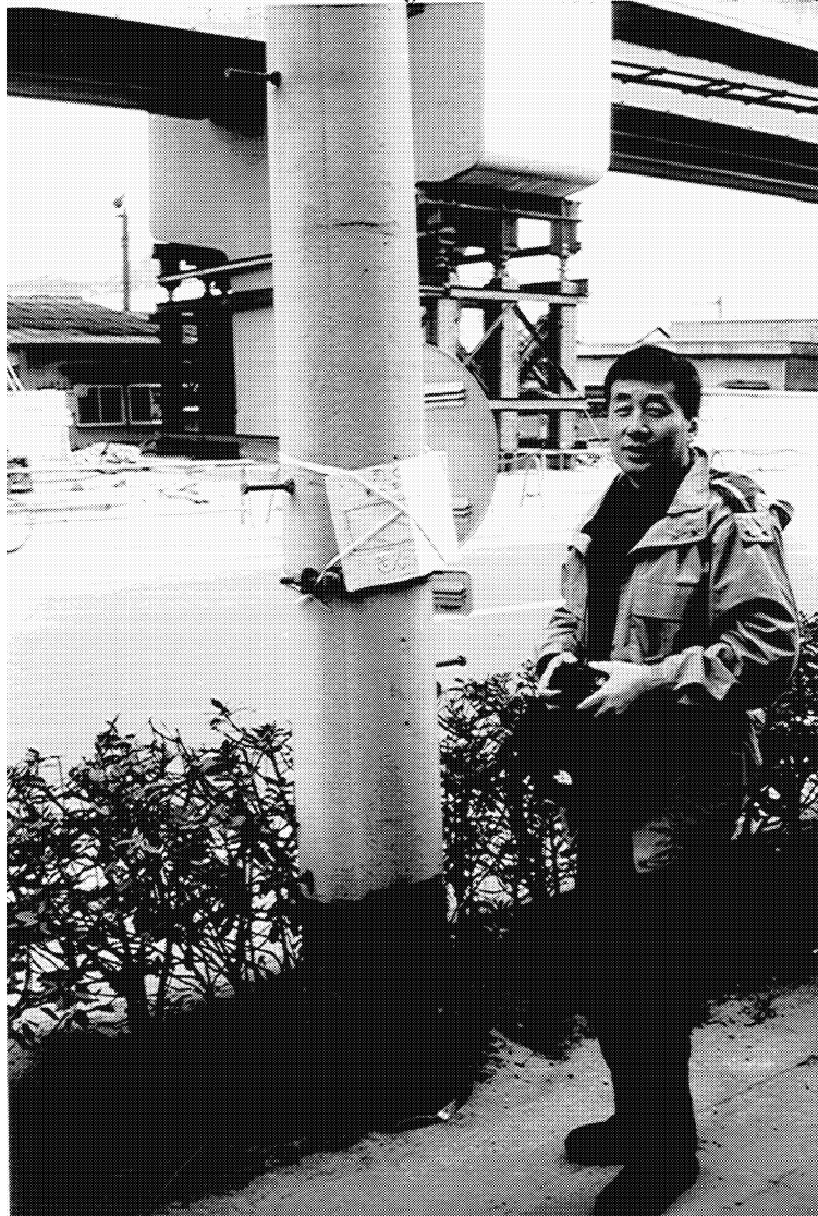
Figure 22 This pole sank about five feet when the soil supporting it liquefied.
