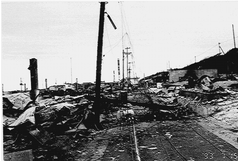
Figure 19 Large areas were destroyed by fire after the Kobe, Japan earthquake. Aerial cables and their wood support poles are vulnerable to fire.
