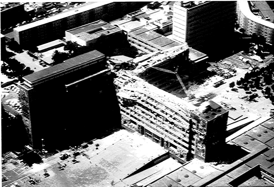
Figure 14 Collapse of top floors of CO in Mexico City disrupted all international calls to and from Mexico.
