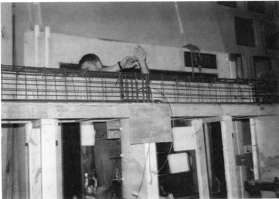
(b) Cap beam reinforcement with forms
