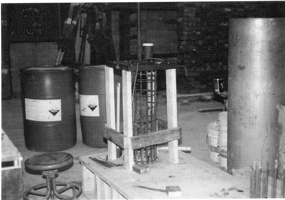
(b) Bottom half-column reinforcement with forms
