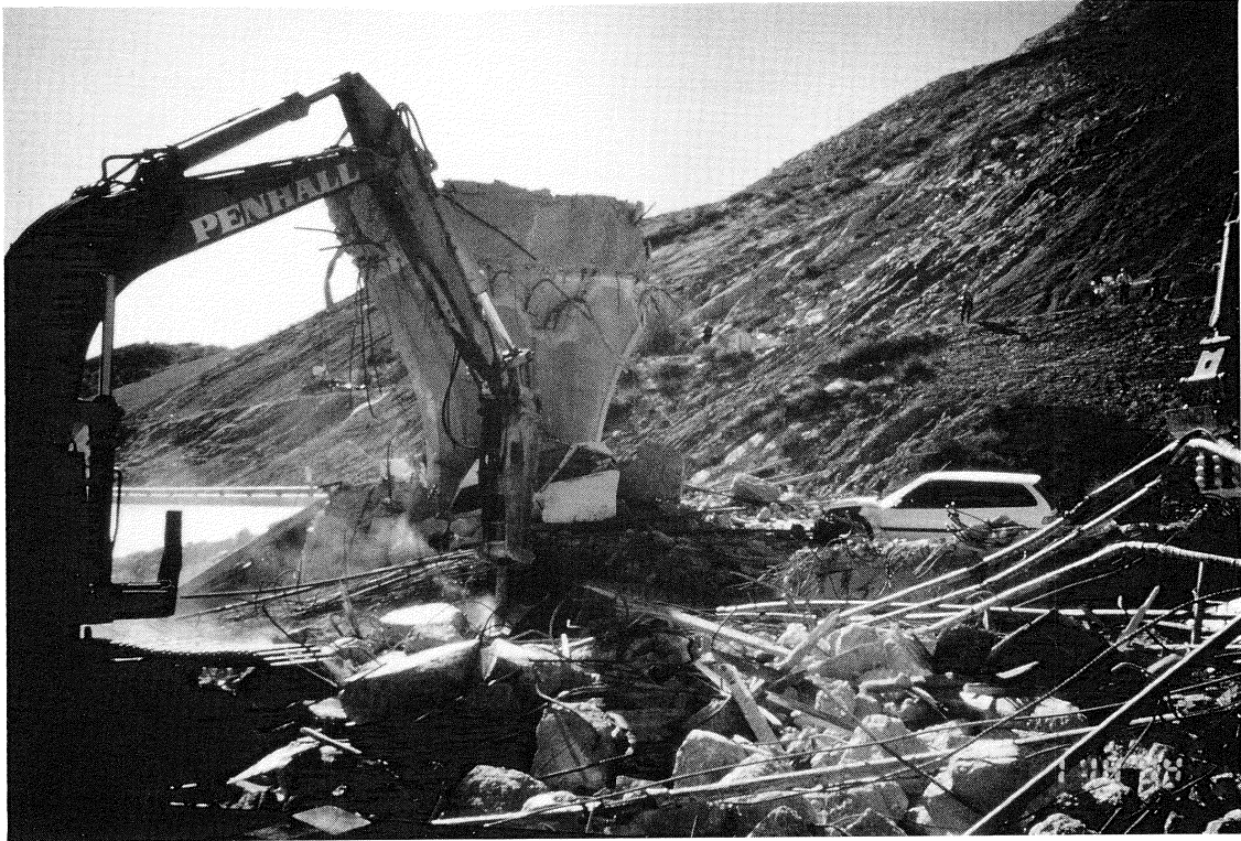
FIGURE 4-12 SR14/I-5 Separation and Overhead (Southbound) - North Side of Pier 3 and Cap
