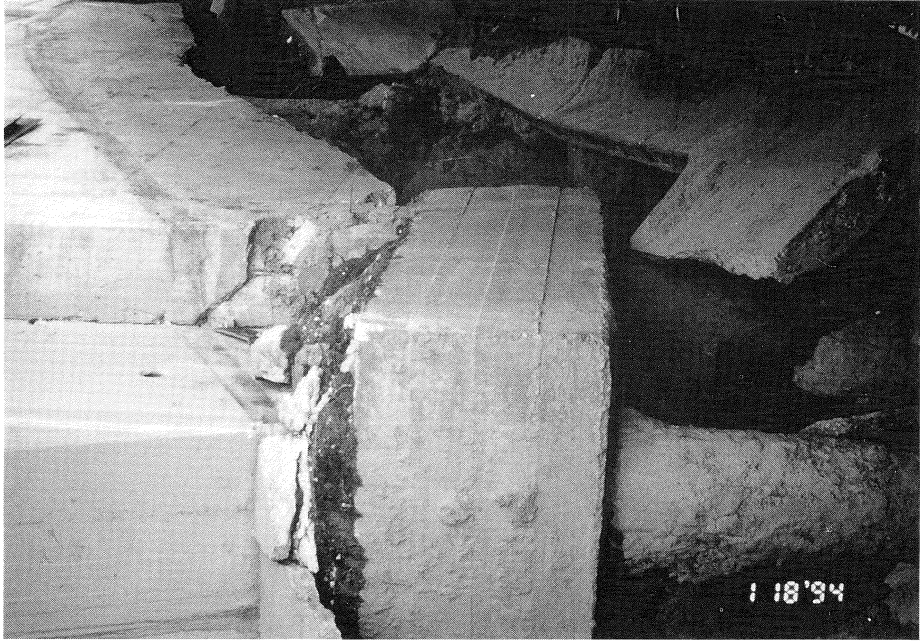
FIGURE 8-5 Balboa Boulevard Overcrossing - CIDH Pile and Cap at Abutment 2
