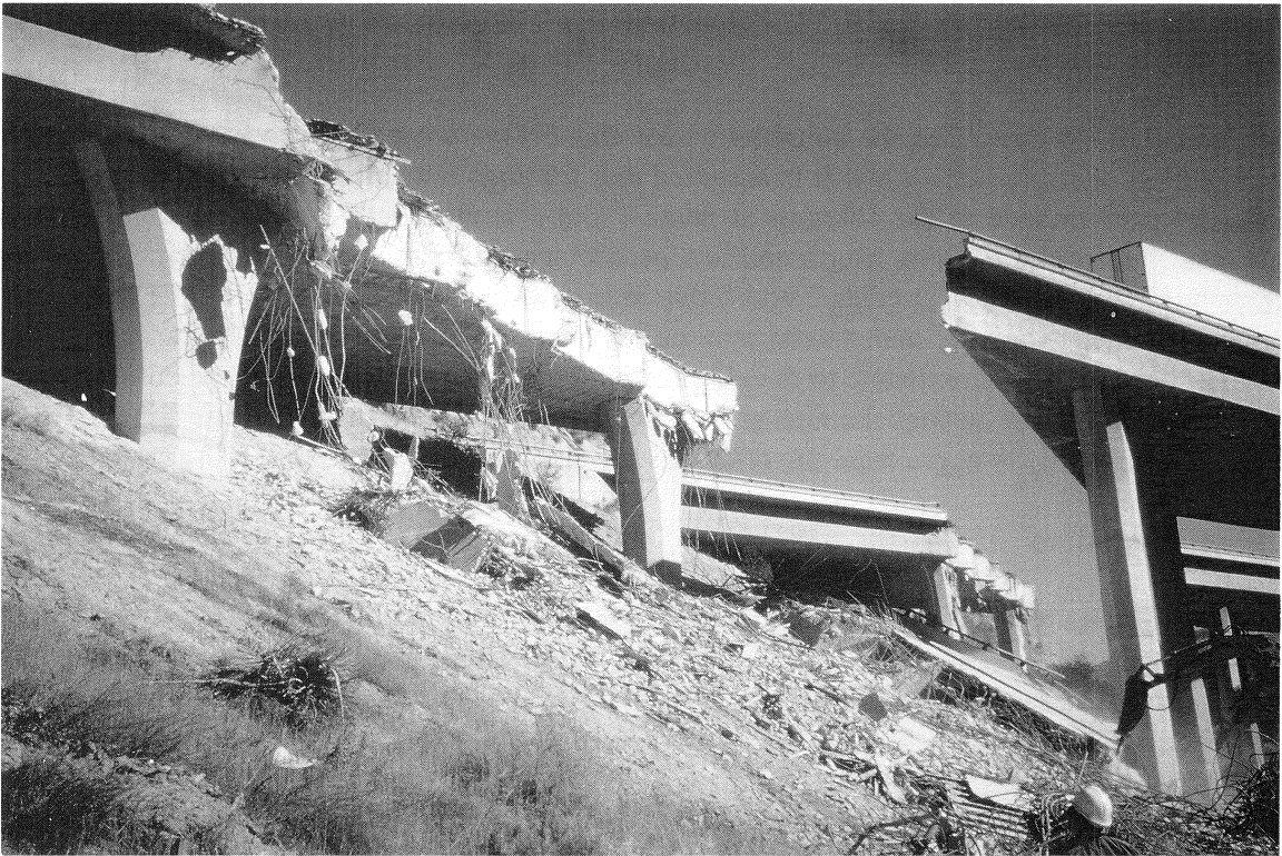
FIGURE 3-6 Gavin Canyon Undercrossing - Collapsed End Spans After Demolition
