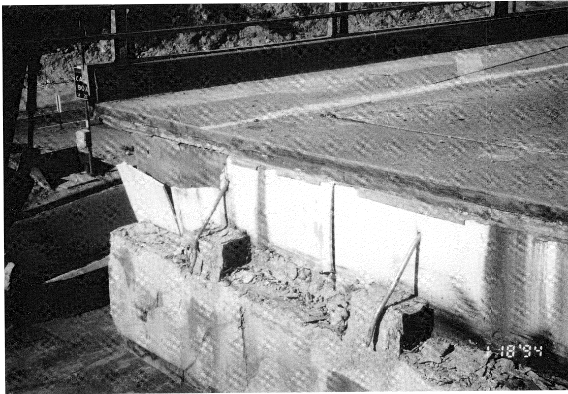
FIGURE 5-3 SR14/I-5 North Connector - Seat and Transverse Shear Keys at Abutment 1
