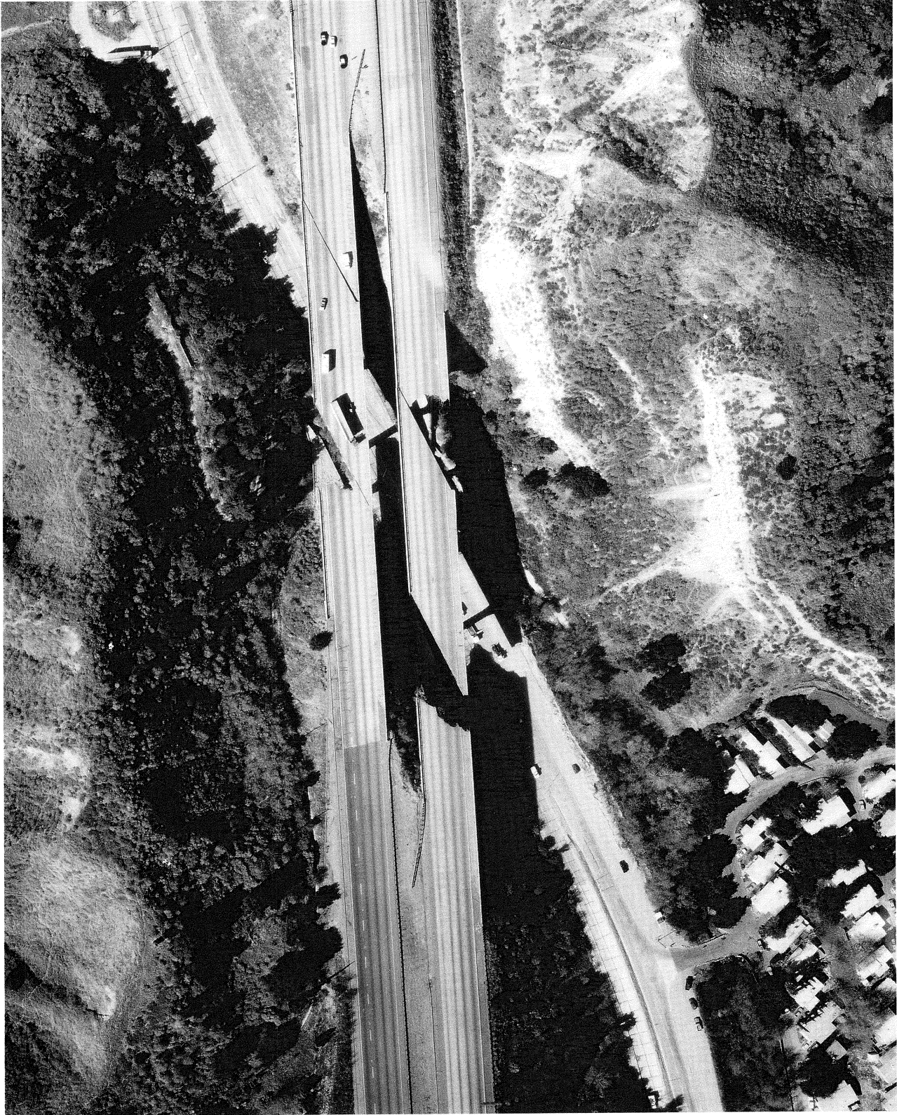
FIGURE 3-4 Gavin Canyon Undercrossing - Aerial View of Collapse
