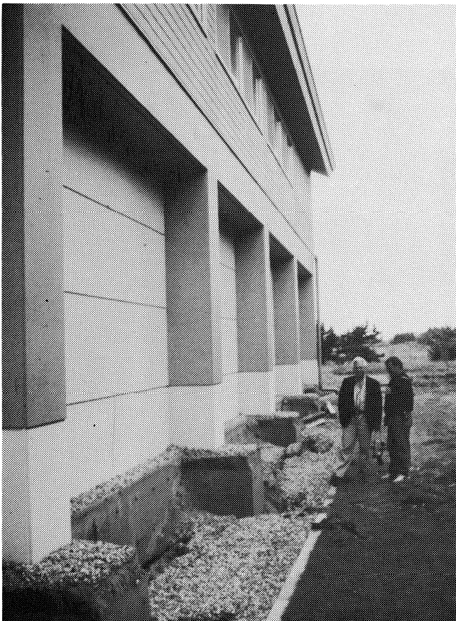
Figure 10-5: Oshamanbe Elementary School--note that the settlement exposed the pile caps.
