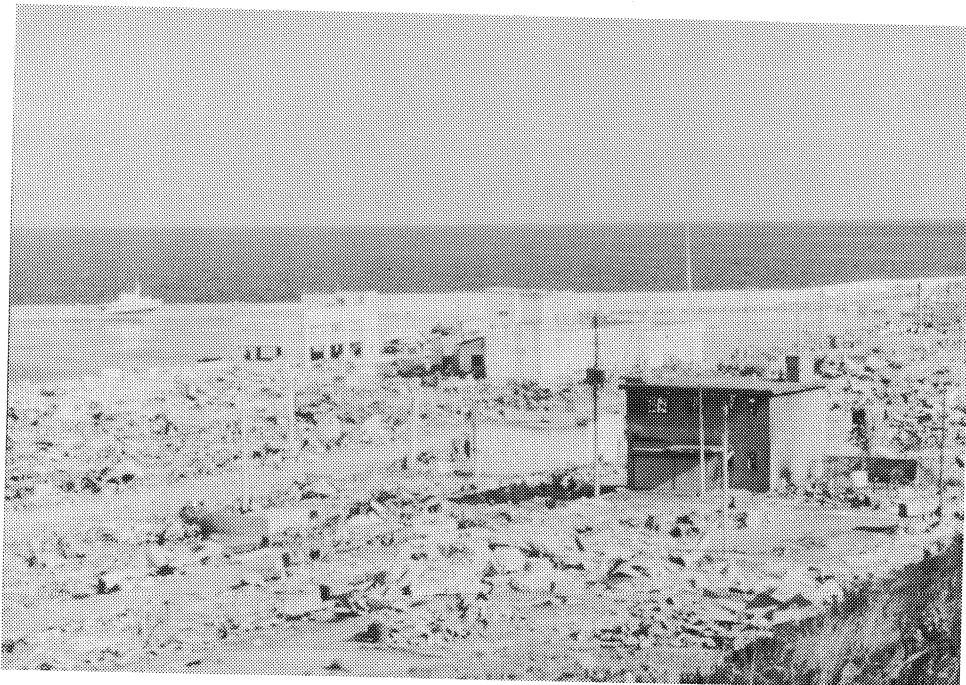
Figure 7-8: A view, looking southeast, of the central port area of Aonae showing tsunami and fire devastation. The only surviving buildings are more substantial concrete-frame buildings. No steel buildings were found in this area.
