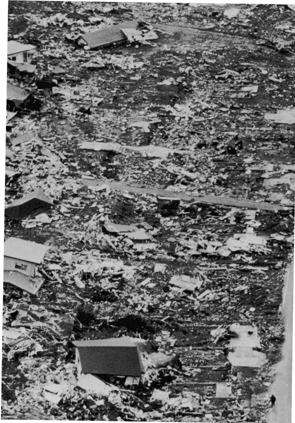
Figure 6-5: A partial view of the area in the previous photograph. The somewhat intact remains are roofs and the upper floors of two (or more) story buildings. These remains have been transported many meters away from their original locations.
