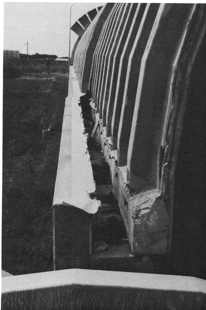
Figure 9-20: Damage at the seat of the precast planks onto the stem wall. The photograph is from the front one-third of the snow shed structure that did not collapse.
