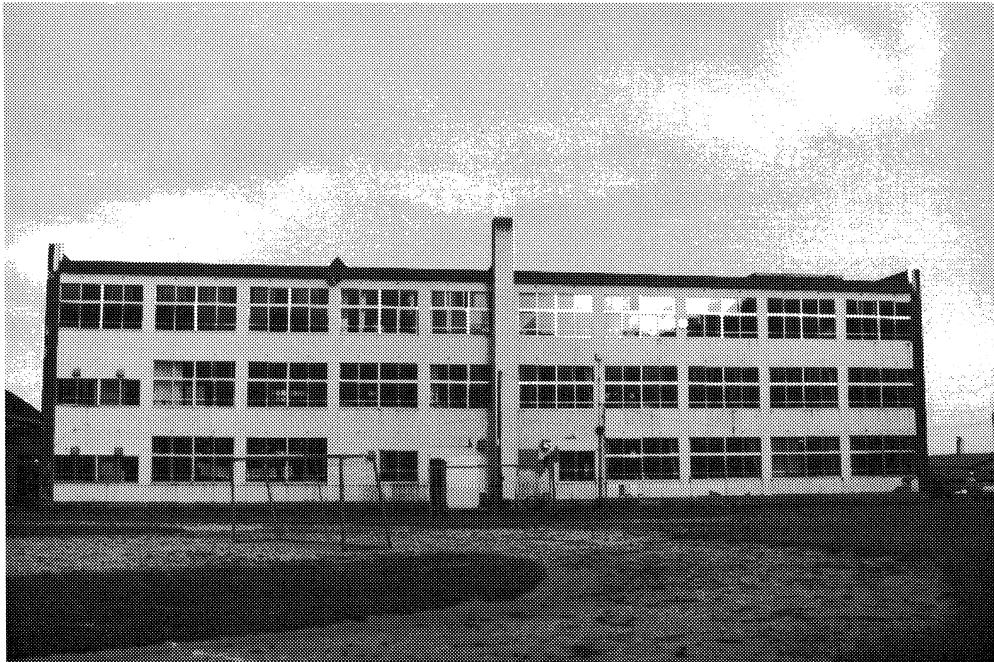
Figure 8-9: Aonae Elementary School, a typical 1950s through early 1970s nonductile concrete-frame building (preceding the lessons learned from the 1971 San Fernando, California, Earthquake). The school, on level ground at sea level, suffered extensive cracking of frame and concrete-block infill-wall elements. These types of buildings have historically suffered extensive damage in Japan (Sendai Earthquake of 1978) and California in 1971, 1979, 1989, etc.). Extensive strengthening of these kinds of buildings has been carried out for all California public schools of similar construction.
