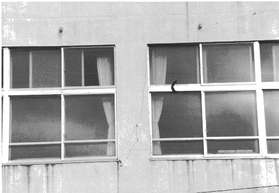
Figure 8-11: The damaged west facade of the Aonae Elementary School. Spandrel and other infill wall cracking has propagated into the columns.
