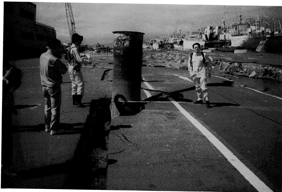
Figure 10-13: Liquefaction effects at the port of Hakodate--a tilted reinforced concrete silo and a buoyant manhole. Photographs courtesy of T. Leslie Youd.
