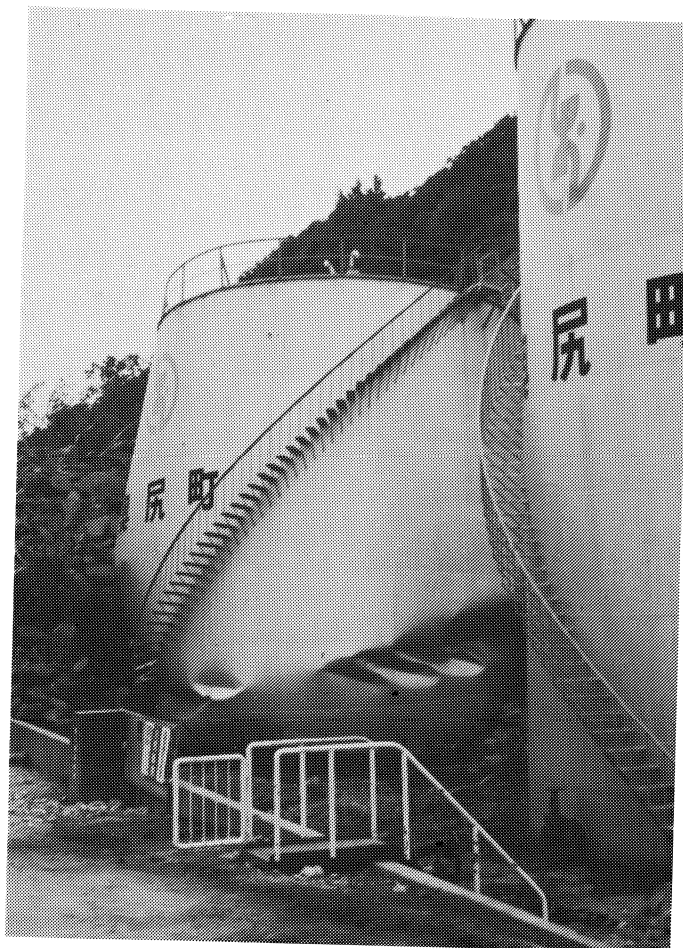
Figure 9-39: Fuel oil tanks in the port of Okushiri-cho; the tank on the left buckled due to landslide impact (the same landslide which caused the collapse of the Hotel Yo Yo)--note that the tank on the right is undamaged.
