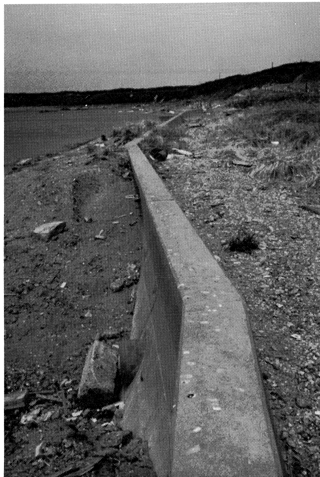
Figure 6-6: Two views of the tsunami walls surrounding the west side of the southern tip of Aonae. Note how the walls have been partially backfilled with sea-borne debris--much of it before the tsunami of the July 12, 1993, earthquake.
