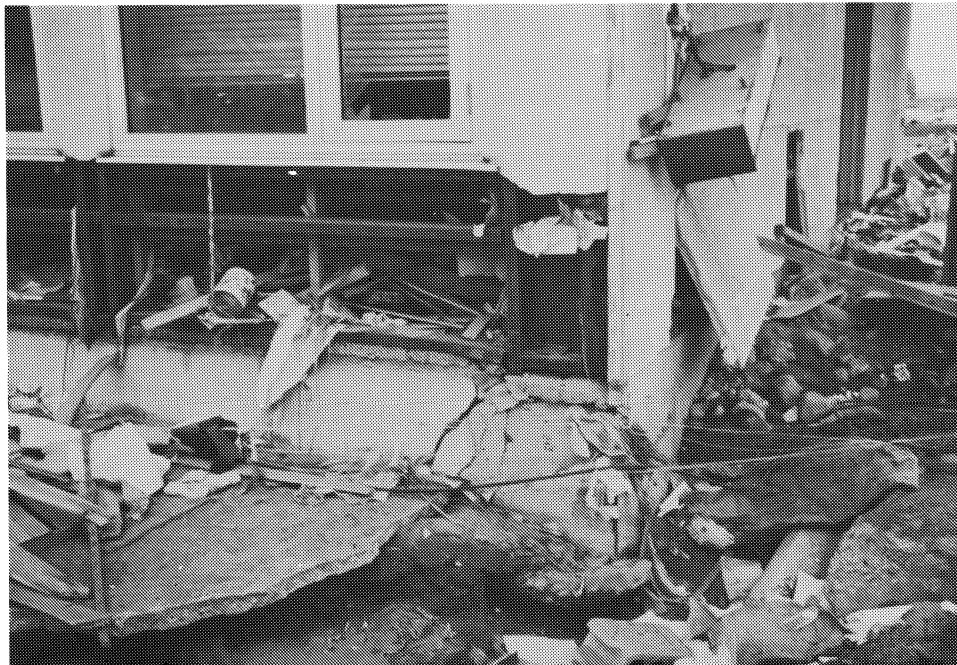
Figure 6-14: The only observed steel-frame building in the tsunami-devastated parts of Aonae. The building suffered some settlement damage (lower photograph), probably due to shaking. Its first-floor interior finishes were damaged extensively, and at least 15 cm of sand was deposited on the ground floor slab. The building is probably repairable, the estimated loss is less than 50% of value. Note the surviving wood-frame building, which was saved by its steel neighbor.
