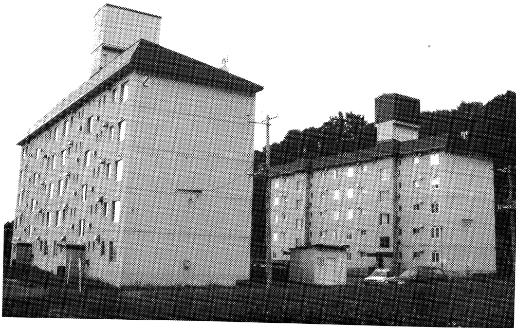
Figure 8-6: Undamaged five-story reinforced concrete shear wall apartment buildings in the outskirts of Okushiri-cho. Minor settlement of fill around the buildings was observed. Several large landslides in steep terrain were visible from the buildings.
