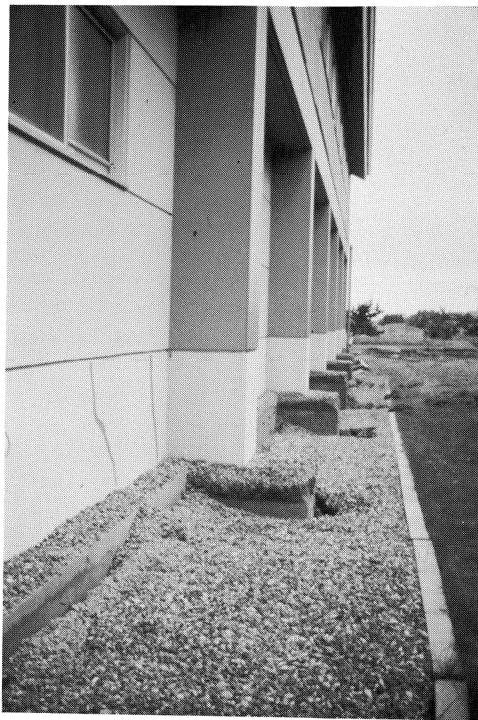
Figure 10-6: Oshamanbe Elementary School--note the minor cracking in spandrels near the column. Other minor cracking of shear walls was observed.
