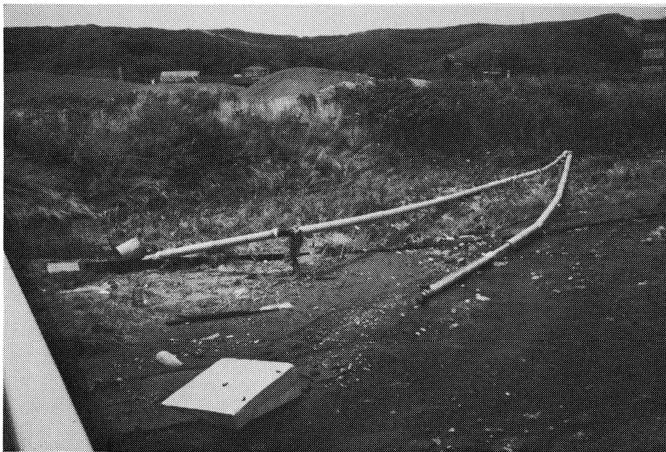
Figure 7-3: The main water line for Aonae was destroyed by the tsunami. This shows views from a bridge of portions of the approximately 20-cm line.
