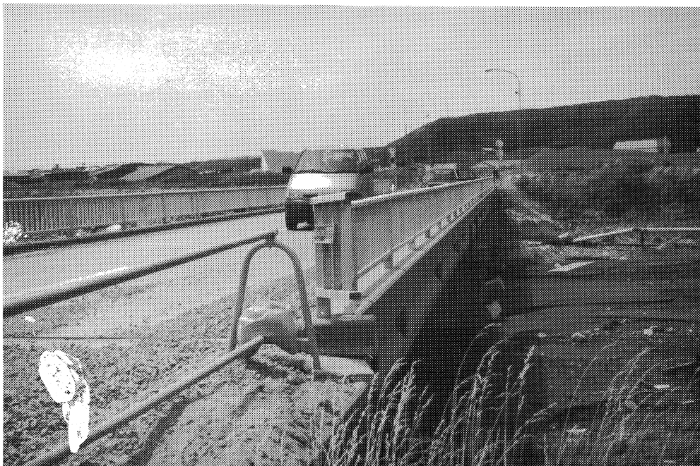
Figure 9-7: A two-lane bridge at Aonae on the coastal road from Okushiri-cho. The bridge was inundated by the tsunami. It suffered minor damage, such as slumping and erosion of abutment fill. One- and two-story wood-frame structures in its vicinity were obliterated by the tsunami.
