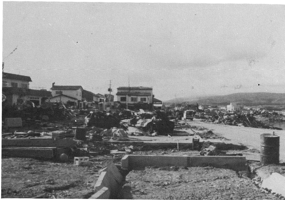
Figure 6-12: Tsunami devastation in the southeastern part of the port area of Aonae. The building foundations in the forefront have been stripped of any wood. Many foundation anchor bolts without any remaining wood-framing were observed throughout the devastated area. The cars (in center) have been rolled over several times. Several people were trapped and killed or drowned in their cars. About 10 days after the earthquake, search teams were still looking for vehicles and trapped victims along the shores of Okushiri Island.
