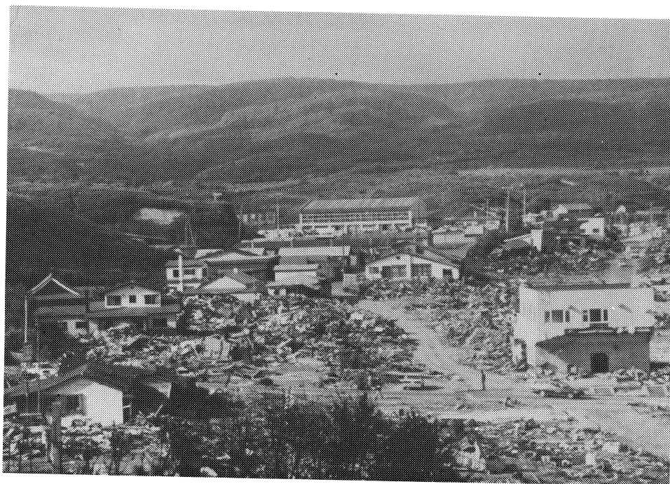
Figure 6-13: A partial view of the central part of Aonae showing tsunami destruction and a surviving steel-frame building on the left. It protected a small wood-frame building (shown in the next photograph)--the only such survivor in this area.
