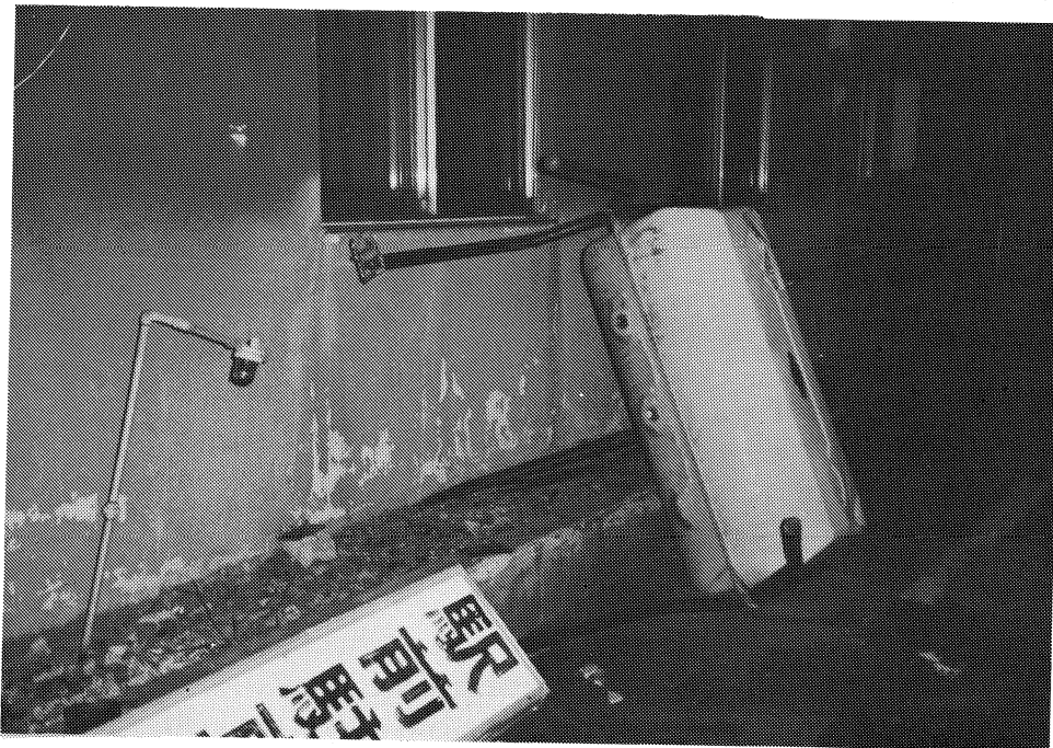
Figure 7-5: An overturned exterior kerosene tank in the town of Kuromatsunai. The highest horizontal acceleration recorded in the main earthquake (0.50g) occurred a few meters away from the tank.
