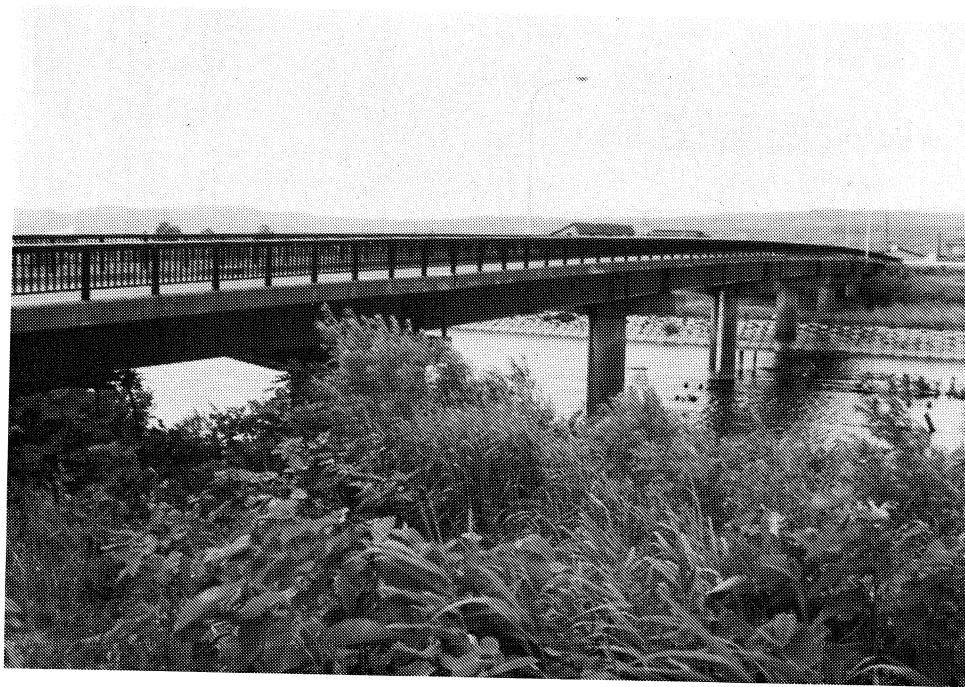
Figure 9-9: A six span, two-lane, 156-m-long, 1970 steel plate girder bridge at Azabu on Highway 277. The bridge suffered severe shear damage to all visible columns, which are about 2 m in diameter. The bridge is located about 70 km from the eastern edge of the aftershock zone. No significant damage to the superstructure was observed. The following figure shows drawings of the bridge.
