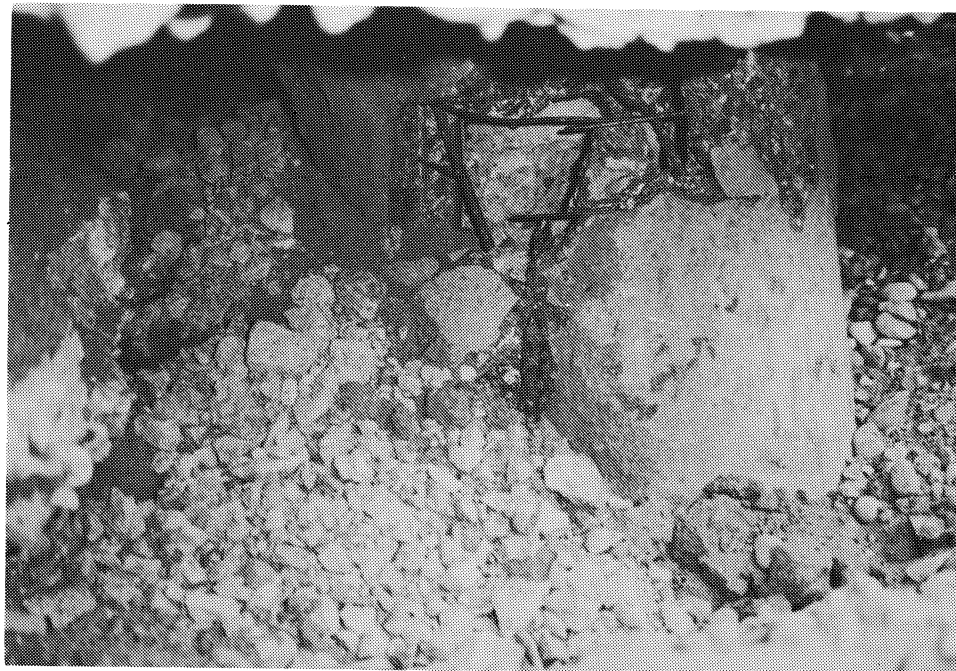
Figure 10-7: Oshamanbe Elementary School--sheared pile just below the cap.
