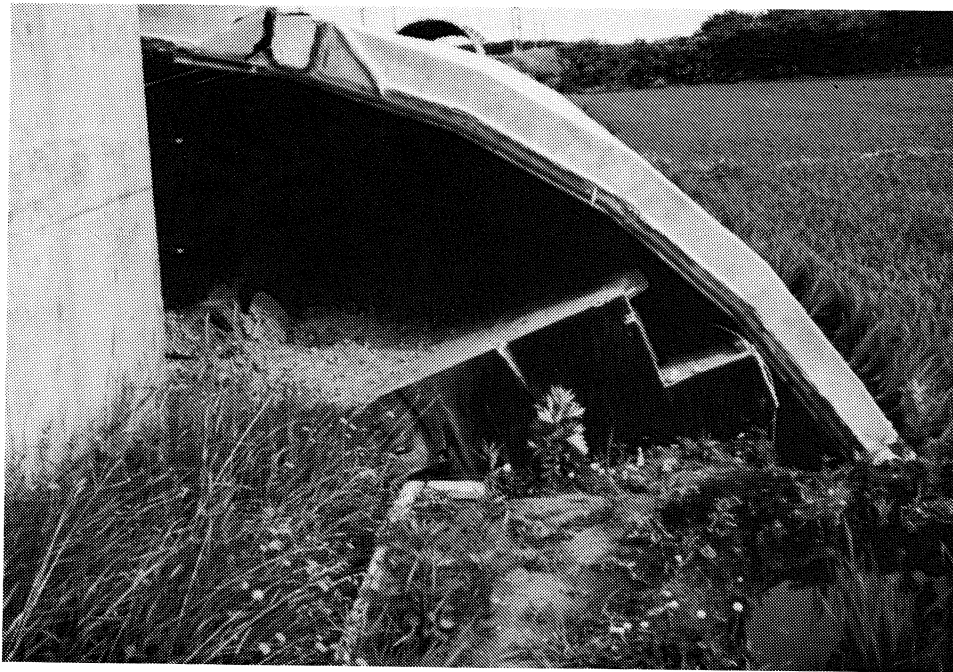
Figure 9-18: Failed east side of the snowshed. Lateral spreading of the fill and/or liquefaction caused spreading of the footings, rotation of the stem wall, and failure of the stem wall.
