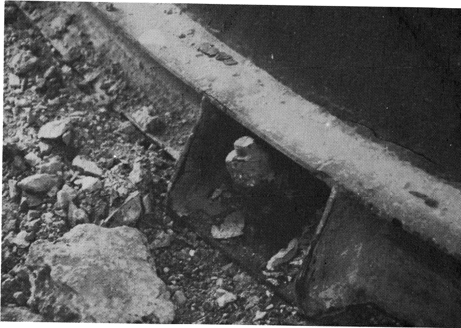
Figure 8-18: OCBP; typical anchorage damage to the two steel silos at the plant. The anchors are somewhat corroded.
