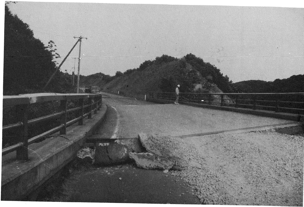
Figure 9-8: Typical road surface damage and abutment fill settlement at a bridge in Okushiri.
