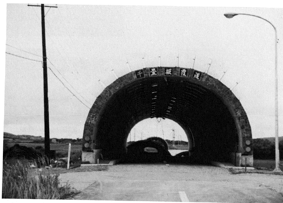
Figure 9-16: A collapsed snowshed (tunnel) north of Aonae. The just-completed structure is on fill in rice paddies. About one-third of the three-hinged arch structure collapsed. The rest is severely damaged. The approximately 2-m-wide quarter-circle panels are precast concrete and are bolted to the footings and to each other at the top.
