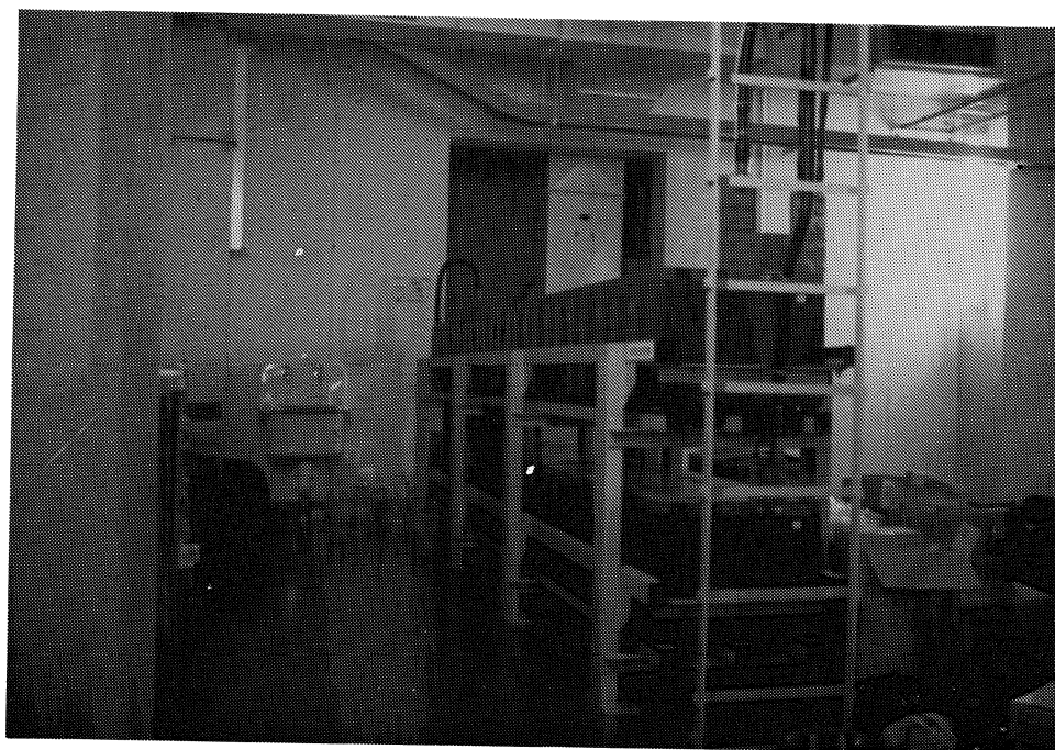
Figure 9-32: Okushiri-cho remote control switch building; the telecommunications equipment in the building was well-braced in both directions, to floor and ceiling. No damage was observed or reported.
