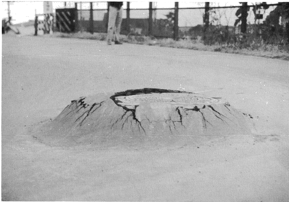
Figure 9-6: Manhole pushed up in Oshamanbe area from settlement. This 30+ cm settlement occurred mostly about 10 to 12 days after the earthquake and was continuing to increase.
