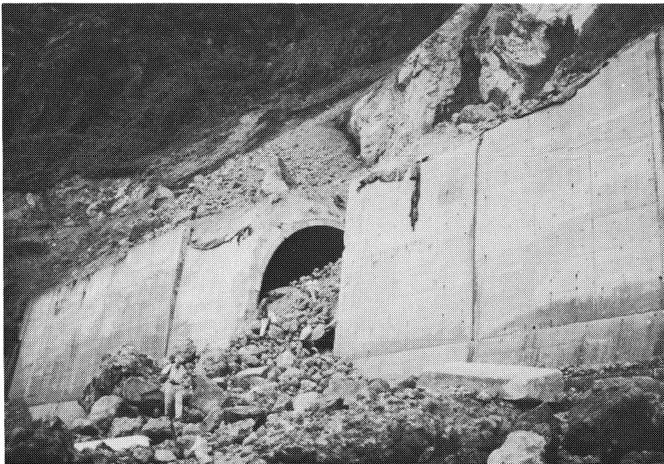
Figure 9-22: Close-up of the failed section of the Shiroito Tunnel.
