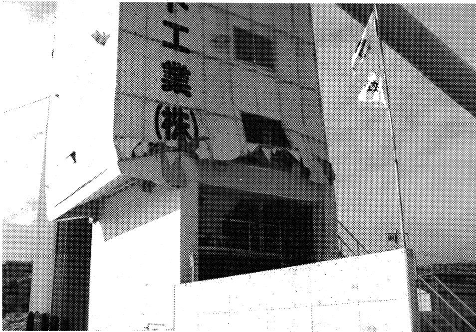
Figure 8-14: OCBP; close-up of the steel-frame hopper superstructure that buckled. The ground-level columns appeared undamaged. Note that the superstructure has dropped about 50 cm.
