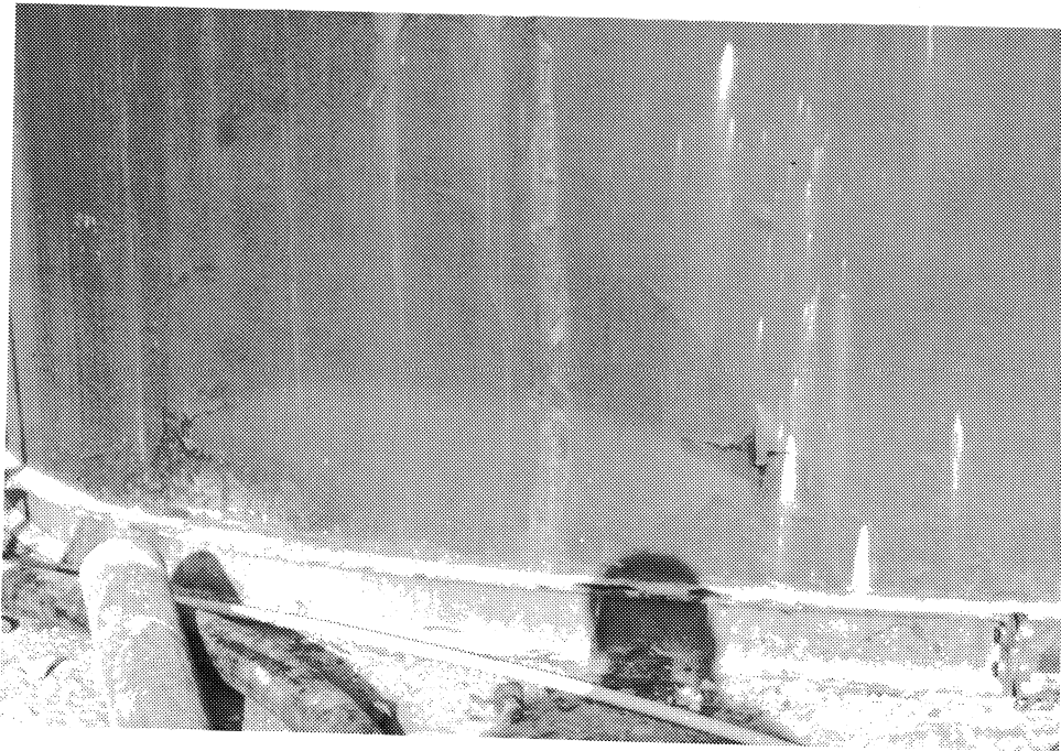
Figure 8-19: OCBP; buckling at the base of one of the two cement silos. Note the damage to the anchorage.
