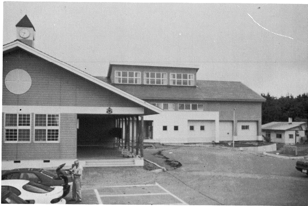
Figure 10-2: Oshamanbe Elementary School; settlement of up to about 1 m and extensive liquefaction occurred. The school is built on top of a 2-m-high fill in a rice paddy area. The school is new. No structural damage other than shearing of piles just below the pile caps was observed. The buildings are a combination of wood frames, concrete frames with shear walls, and steel frames.
