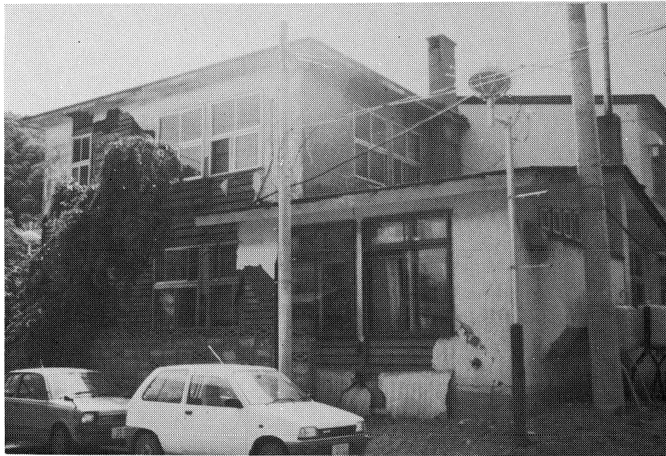
Figure 8-4: The light wood-frame and stucco City Offices Building in Okushiri-cho (upper photograph) and a smaller building (lower photograph) suffered extensive damage to their stucco facades but not major structural damage. These rather flimsily built structures suffered probably as much damage from shaking as any building observed in the town.
