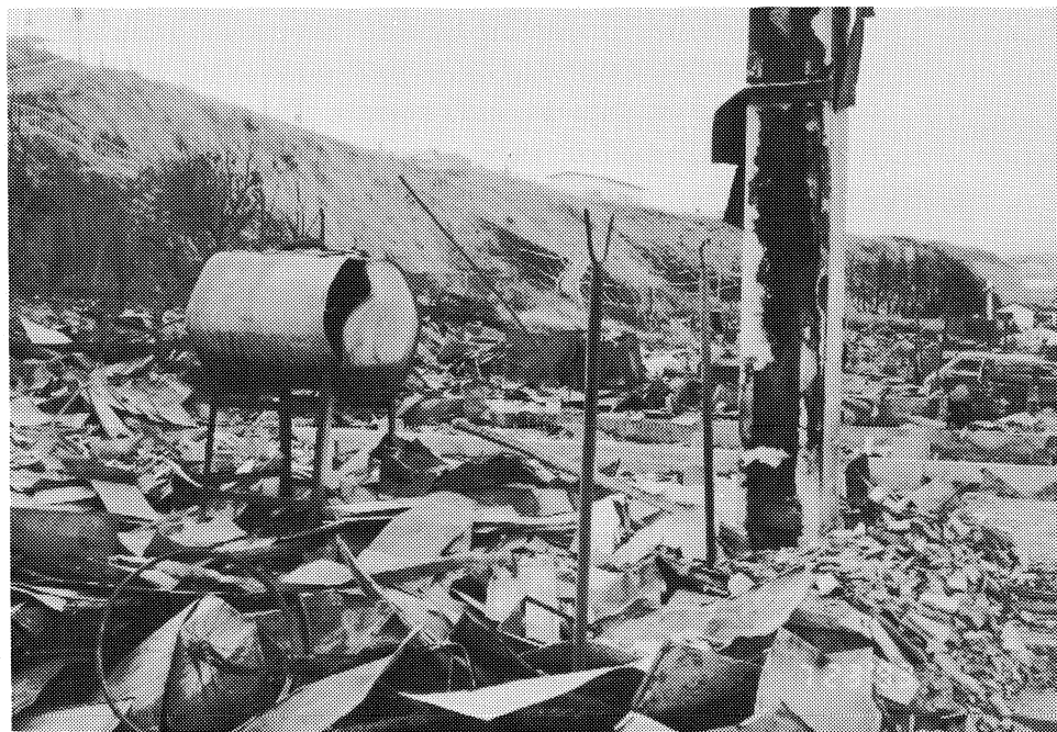
Figure 7-6: A view of a small part of the burned out area of Aonae (top photograph). Note the standing kerosene tank. These and other such tanks, containing fuels, added much fuel to the fire. The vertical columns are chimneys (of wood-frame buildings), which survived the earthquake, tsunami, and fire. Note that the roads have been cleared of debris. The lower photograph shows an exploded kerosene tank.
