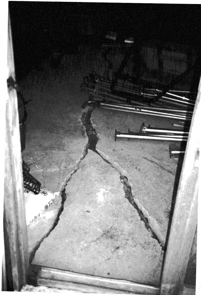
Figure 8-12: Aonae Elementary School. Settlement of fill in the southeast corner of the three-story building (upper photograph) and a cracked floor slab (lower photograph) indicate that the ground failure extended below the structure.
