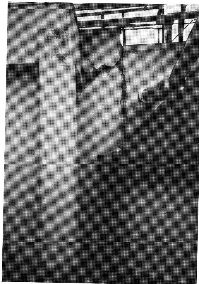
Figure 9-26: ASTP; ground settlement of the main structure of about 30 cm (upper photograph) and damage due to settlement and pounding between a structure and a digester (lower photograph).
