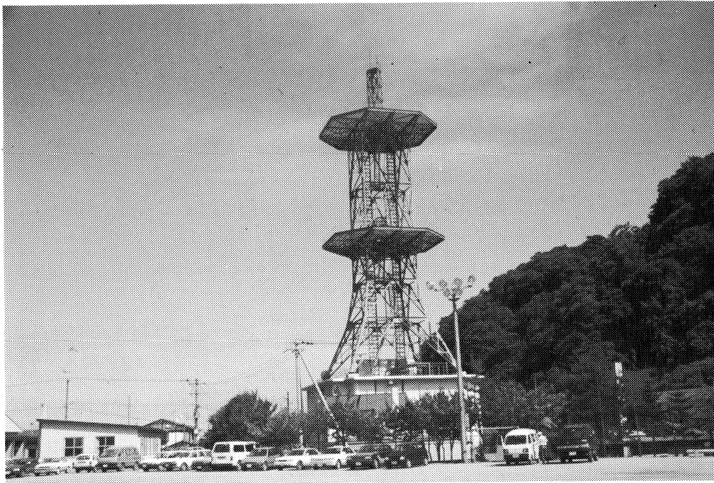
Figure 9-30: Okushiri-cho remote control switch building; this concrete shear wall building supports an approximately 40-m freestanding steel truss microwave tower.
