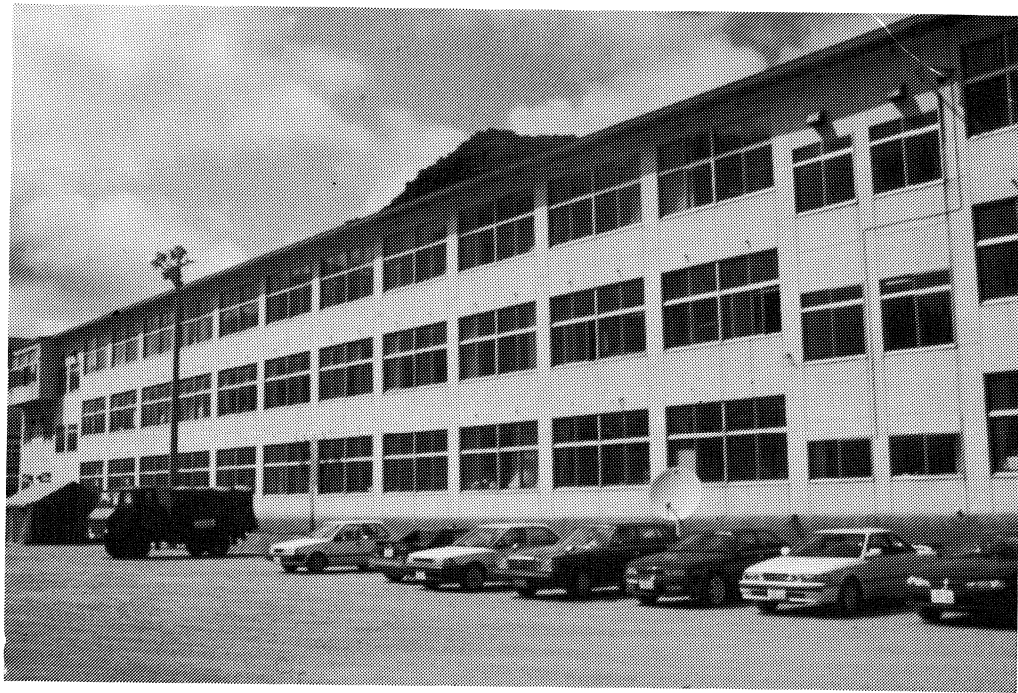
Figure 8-5: The apparently undamaged 1970 reinforced concrete-frame Okushiri-cho elementary school.
