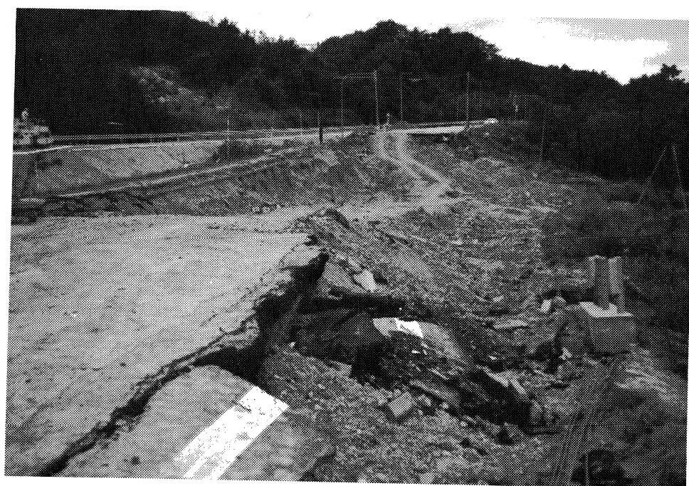
Figure 9-2: The embankment of Highway 5 near Kuromatsunai failed in a flow-slide, taking out both the road and a railroad embankment (which is at the bottom of the upper photograph). Upper photograph by K. Kawashima.
