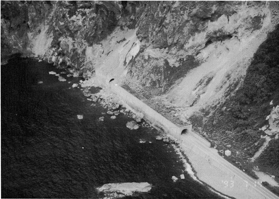
Figure 9-21: Collapsed Shiroito Tunnel north of Setana on Highway 229. Collapse was caused by a large rockfall from above. The tunnel was intended to protect the highway against rockfalls; this rockfall was bigger than designed for. Note that adjacent sections of the collapsed portion of the tunnel have been displaced. Photograph by K. Kawashima.
