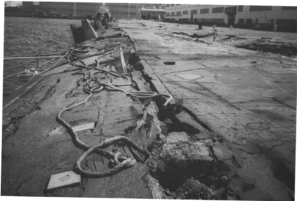
Figure 9-34: Examples of typical damage from the ports of Setana (upper photograph) and Hakodate (lower photograph; photo courtesy of T. Leslie Youd), where quay walls displaced or tilted seaward by as much as 3 m. A peak horizontal ground acceleration of 0.12g was recorded nearby.
