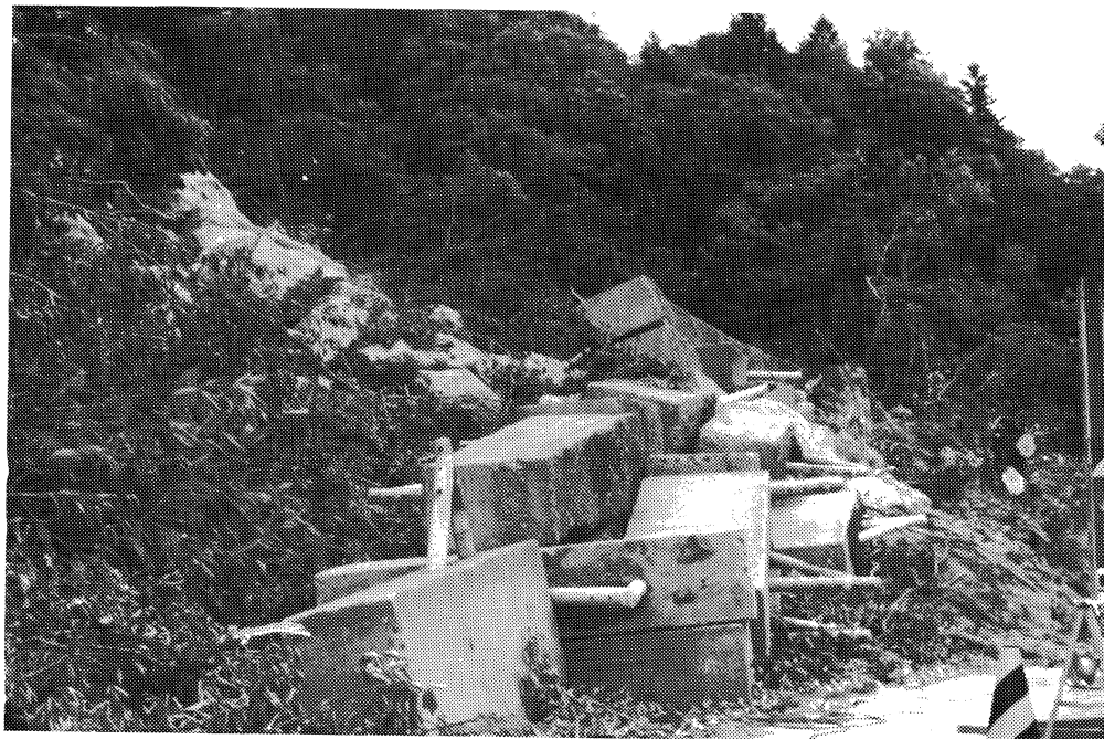
Figure 9-4: Landslide damage to a retaining wall along Highway 230 near Setana.
