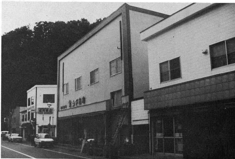
Figure 8-2: Lightly damaged commercial buildings in Okushiri-cho. Typically these buildings are wood-frame with stucco. Note the damaged stucco and brick veneer.
