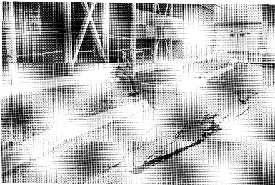
Figure 10-3: Oshamanbe Elementary School; settlement at the entrance of about 1 m.
