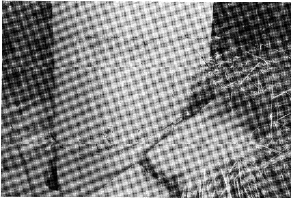
Figure 9-14: Azabu Bridge--settlement of fill (below the paving) away from a bridge pier due to lateral spreading of the fill into the river.
