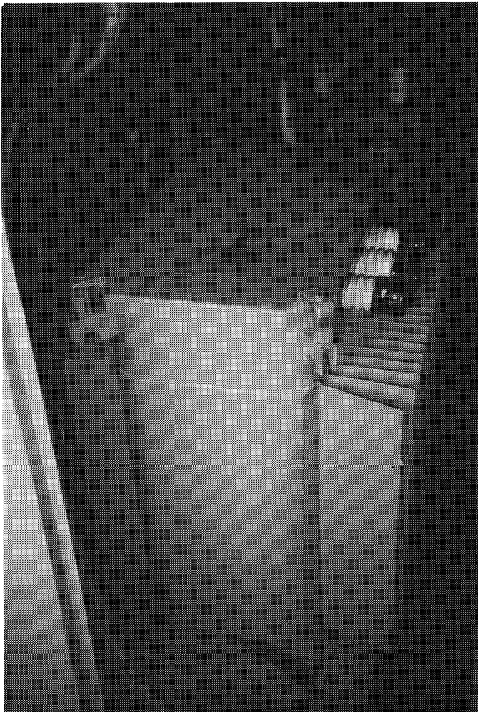
Figure 9-28: ASTP; this transformer overturned. It was housed in the cabinet to the left. It is located on the second floor of the main structure.
