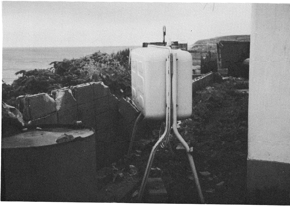
Figure 7-4: A typical kerosene tank for a small building. The fuel is used for heating in Japan (including Tokyo). This tank, in Aonae at the lighthouse, was not anchored and tipped over, severing the small fuel line which is typically about 1/4 inch (0.5 cm) in diameter. Numerous such tanks, many tipped over, were observed on the Island of Okushiri and on Hokkaido (following figure). They are very hazardous and contributed to the fire that destroyed much of the town of Aonae following the earthquake and tsunami. There seemed to be no enforced requirement to anchor such tanks. That practice needs to be changed.
