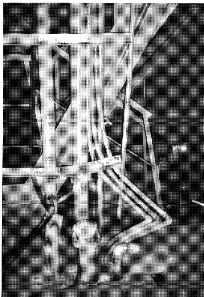
Figure 8-16: OCBP; damage to the large-bore hopper ducting due to differential displacements at its supports—caused by the buckling and shortening of the hopper structure.
