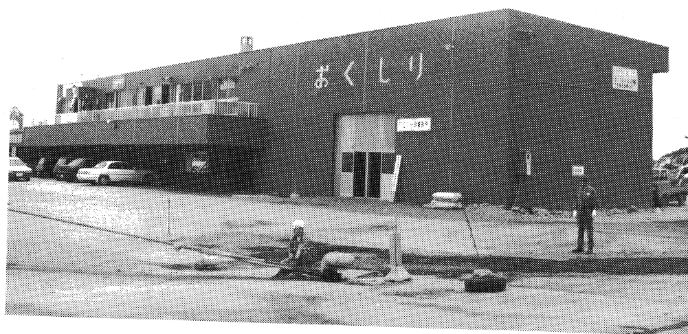
Figure 8-3: The reinforced concrete-frame Ferry Building in Okushiri. The ground-floor finishes were extensively damaged by the tsunami. The building had some damage due to local settlement in one corner.
