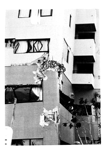
Figure 5-2: A partial collapse occurred in the seaward wing of the Royal Palms Condominiums. A discontinuity in masonry in-fill at the second floor concentrated shear on the corner columns.
