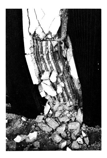
inches relative to the foundation, shattering concrete in the ground floor columns. Some of the columns lost their ability to resist gravity loads, leaving portions of the building supported by the in-fill masonry walls. The building was subsequently slated for demolition.
