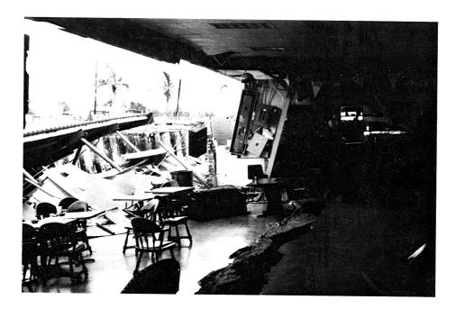
Figure 4-2: Liquefaction in the soft alluvium and fill beneath the Navy port area created fissures running several hundred meters (top photo). The enlisted personnel's shoreline club partially collapsed due to liquefaction-induced spreading beneath the structure (bottom photo).
