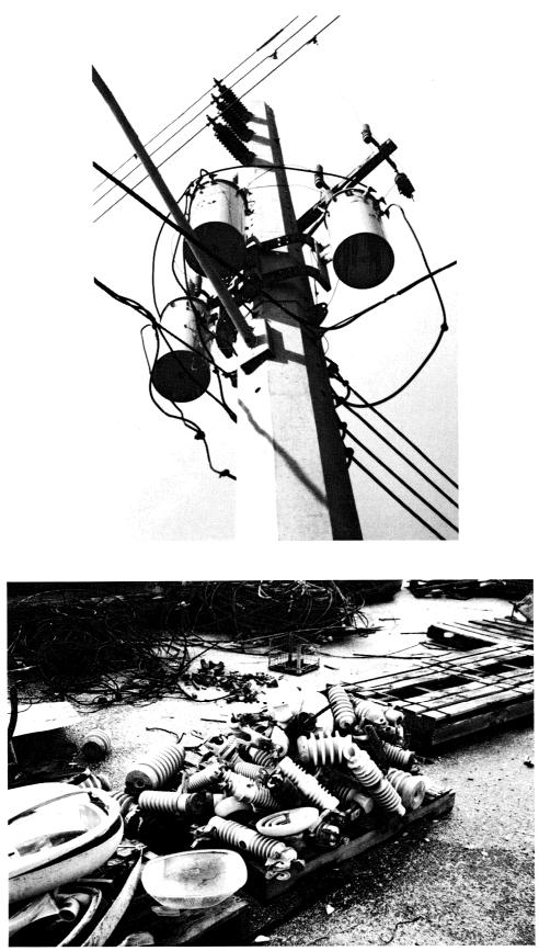
Figure 6-1: Wind loads on Guam result in power and transmission poles of heavy reinforced concrete (top photo). A small portion of poles suffered broken ceramic insulators. Broken insulators are collected on pallets in the Power Authority's service yard (bottom photo).
