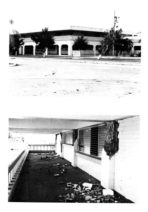
Figure 5-1: One wing of Inarajan High School suffered shattered concrete due to the short column effect, where shear loads from half-height masonry in-fill were transferred into the columns.
