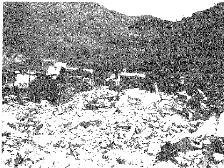
Figure 3-2 Widespread collapse of unreinforced masonry buildings.
