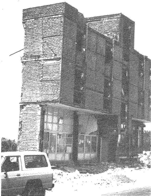
Figure 3-9 Masonry infill constructed with light steel reinforcement
