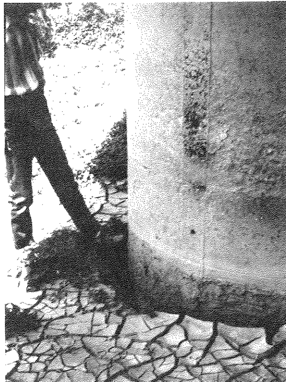
Figure 3-21 Concrete bridge with large lateral pier displacement appears to be undamaged
