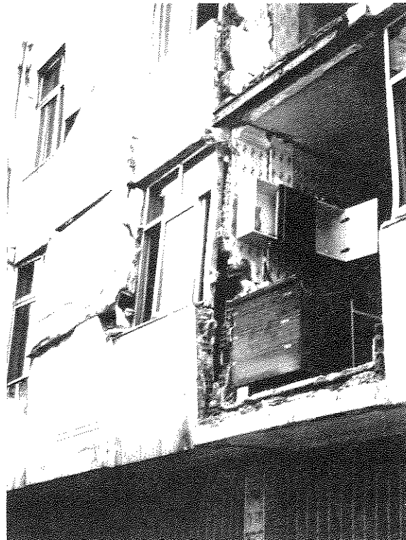
Figure 3-8 Typical damage to hollow clay unreinforced masonry infill walls
