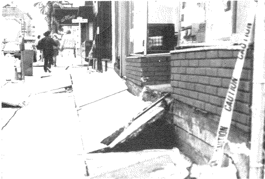
FIGURE 2-6. Differential Settlement of 0.1 to 0.3 m Adjacent to Building at Corner of 7th St. and Natoma St. (photograph by T. D. O'Rourke)
