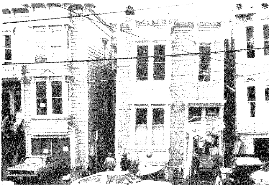
FIGURE 2-3. Racking and Settlement of Houses on Shotwell St. Between 17th and 18th Sts. in 1989. These Houses are Directly Behind the Location of Houses in Figure 2-2 (photograph by T. D. O'Rourke)
