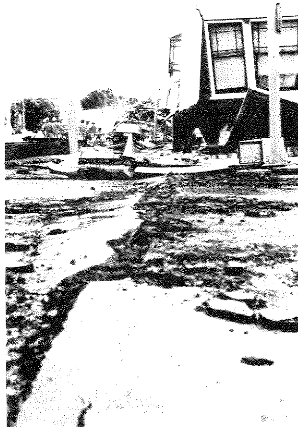
FIGURE 2-12. Sand Ejected from Garage of Building on Scott St. (photograph by H. E. Stewart)
