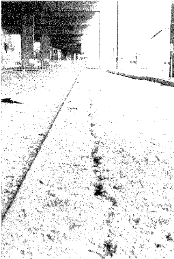
FIGURE 2-10. Open 25-mm Crack Beneath the Embarcadero Skyway Between Howard and Mission Sts. Showing Movement Toward the Bay (photograph by T. D. O'Rourke)
