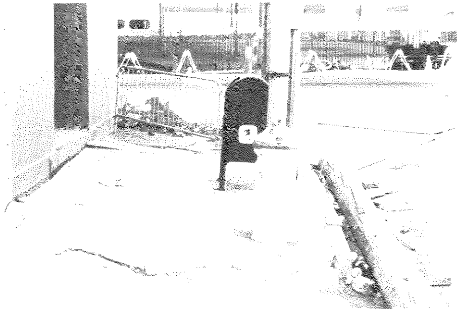
FIGURE 2-7. Differential Settlement at Corner of 6th St. and Townsend St. (photograph by T. D. O'Rourke)
