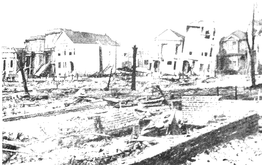
FIGURE 2-2. Racking and Settlement of Houses on South Van Ness Between 17th and 18th Sts. in 1906 [after Lawson, et al., 1908]
