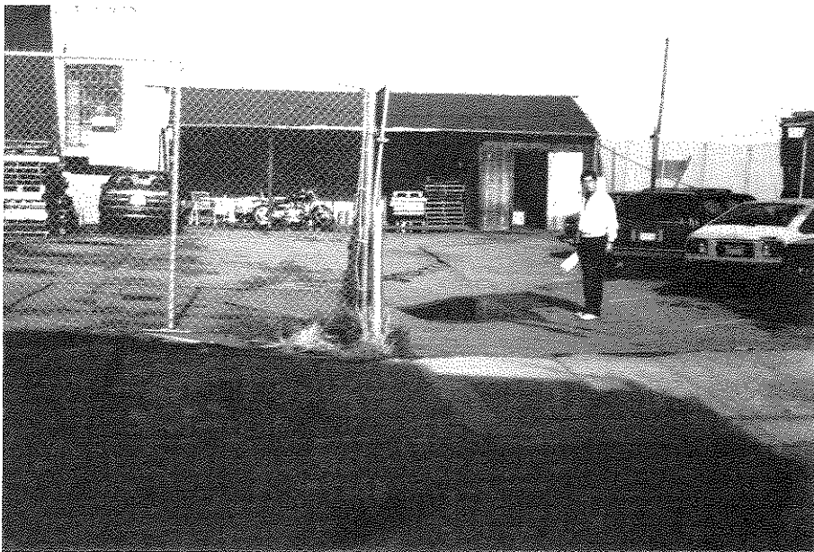
FIGURE 2-5. Differential Settlement Along Dore St. Just North of Bryant St. in 1989 (photograph by T. D. O'Rourke)
