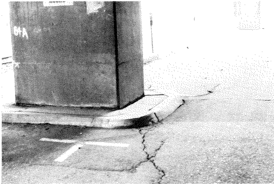
FIGURE 2-11. Differential Settlement Adjacent to Pile-Supported Column of Embarcadero Skyway Near Mission St. (photograph by T. D. O'Rourke)
