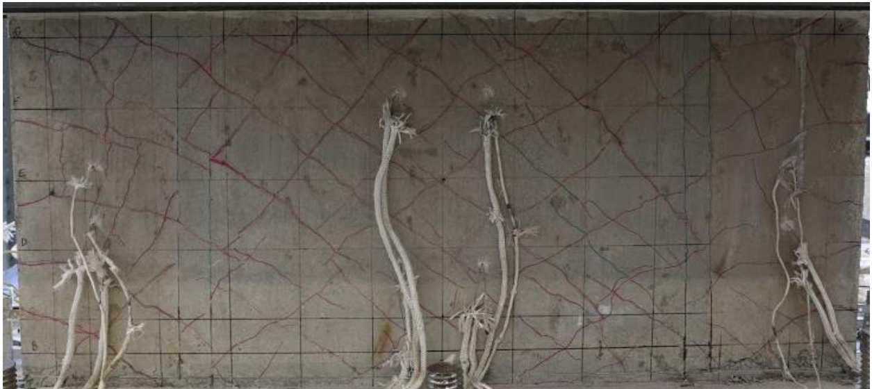
Figure 4-14. Crack pattern on West face of Wall 2 after LC16
