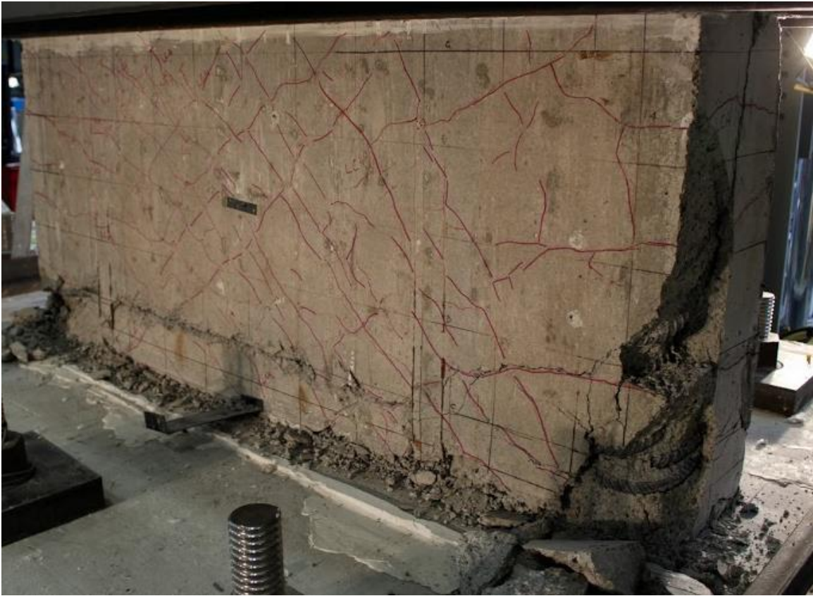
Figure 4-22. Damage to Wall 3 at the end of testing
