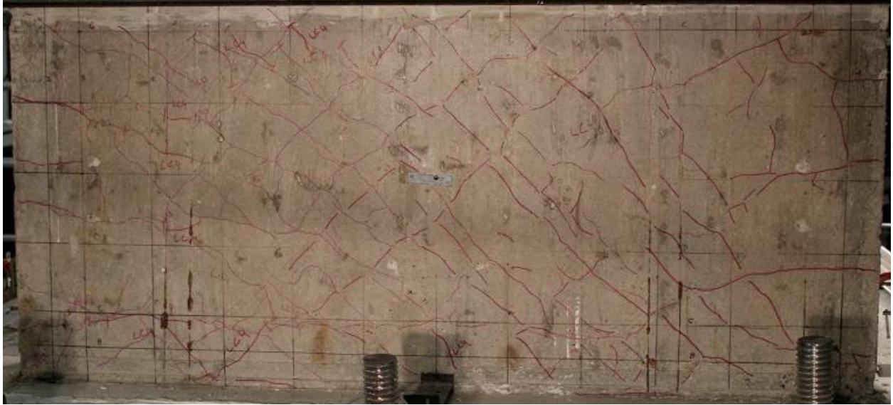
Figure 4-21. Crack pattern on West face of Wall 3 after LC15
