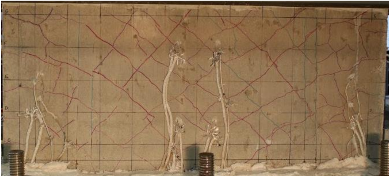
Figure 4-12. Crack pattern on West face of Wall 2 after LC8
