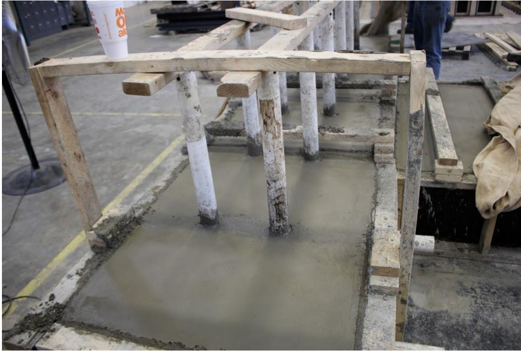
Figure 3-9. Finished concrete surface of a wall and its foundation
