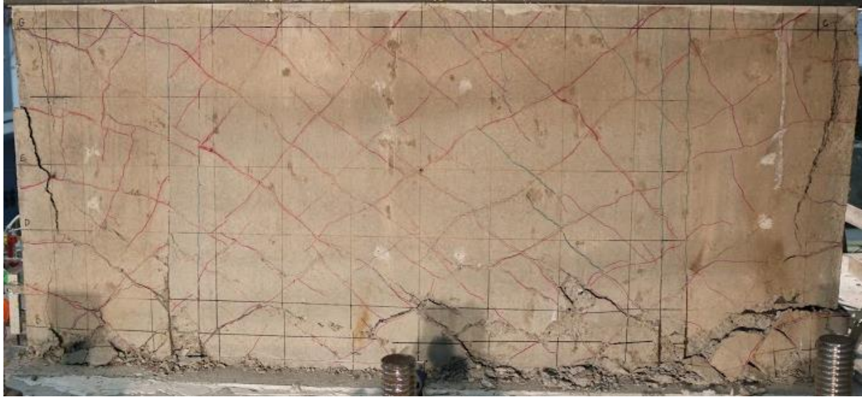
Figure 4-15. Damage to Wall 2 at the end of testing
