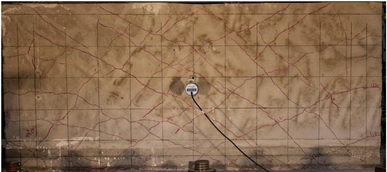
Figure 4-6. Crack pattern on East face of Wall 1 after LC15
