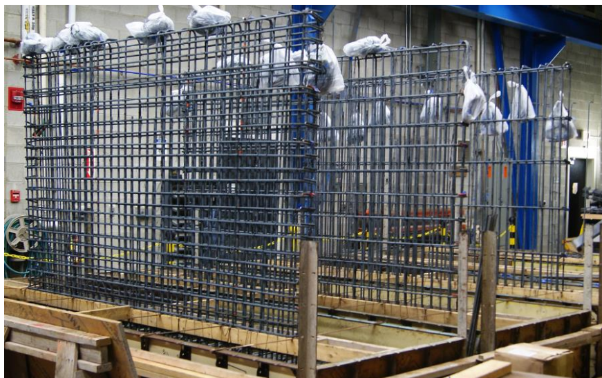
Figure 2-26. SW8 through SW10 rebar cages
