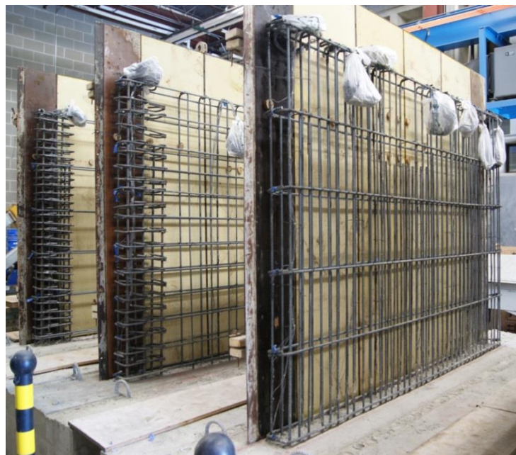
Figure 2-27. Wall formwork for specimens SW10 through SW12
