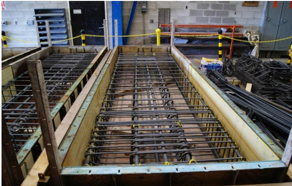
Figure 2-24. SW12 foundation rebar cage
