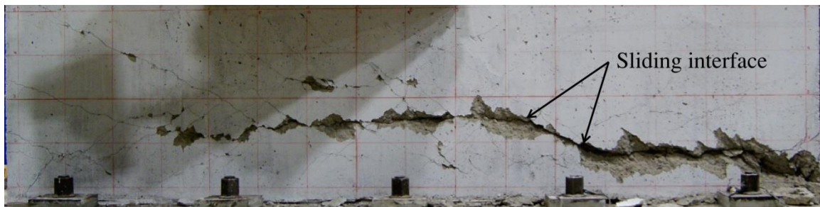
Figure 5-1. Crack in wall SW5 after LS8 (peak transient drift ratio of 0.89%)
