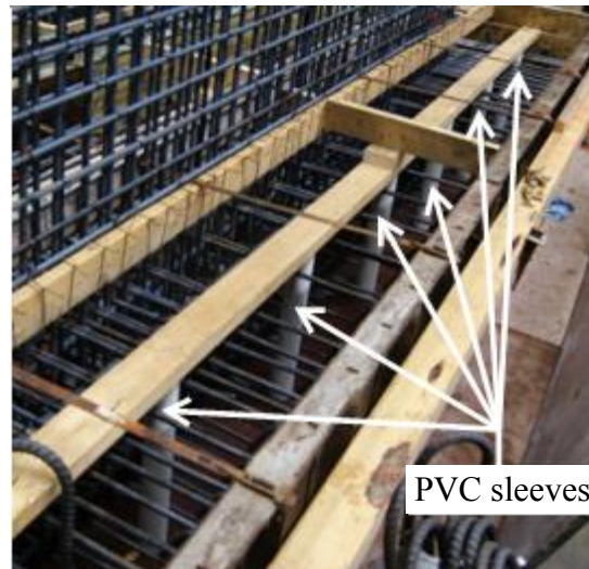
Figure 2-25. Vertical PVC sleeves in the foundation
