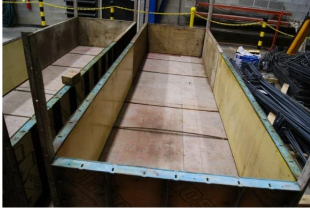
Figure 2-23. Typical foundation formwork
