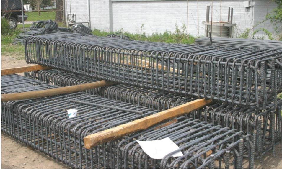
Figure 3.2. Pre-fabricated reinforcement cages for the Phase I foundations
