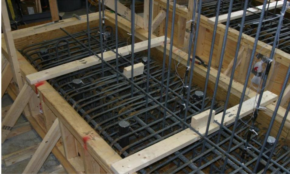
Figure 3.4. Rebar cage positioned inside formwork, Phase I foundation
