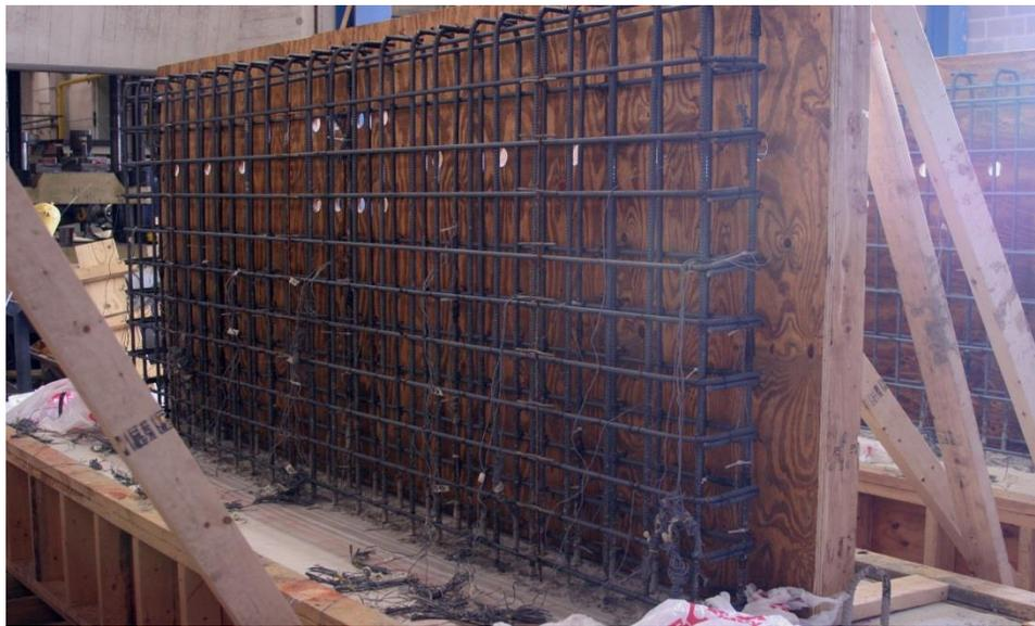
Figure 3.7. SW5 prior to finishing of wall formwork
