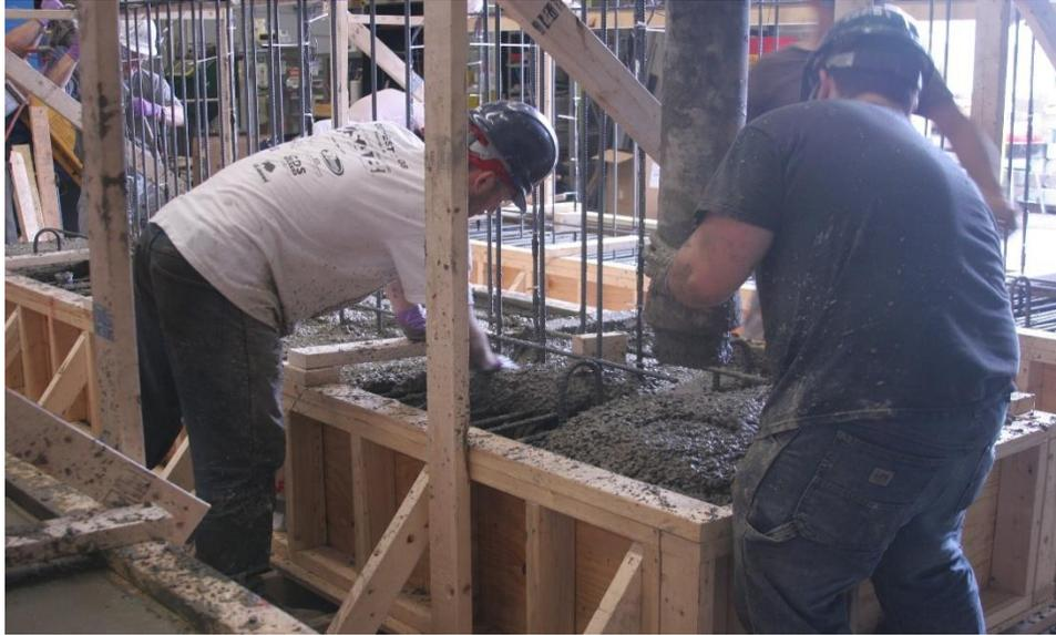
Figure 3.6. Pouring of Phase I foundation concrete
