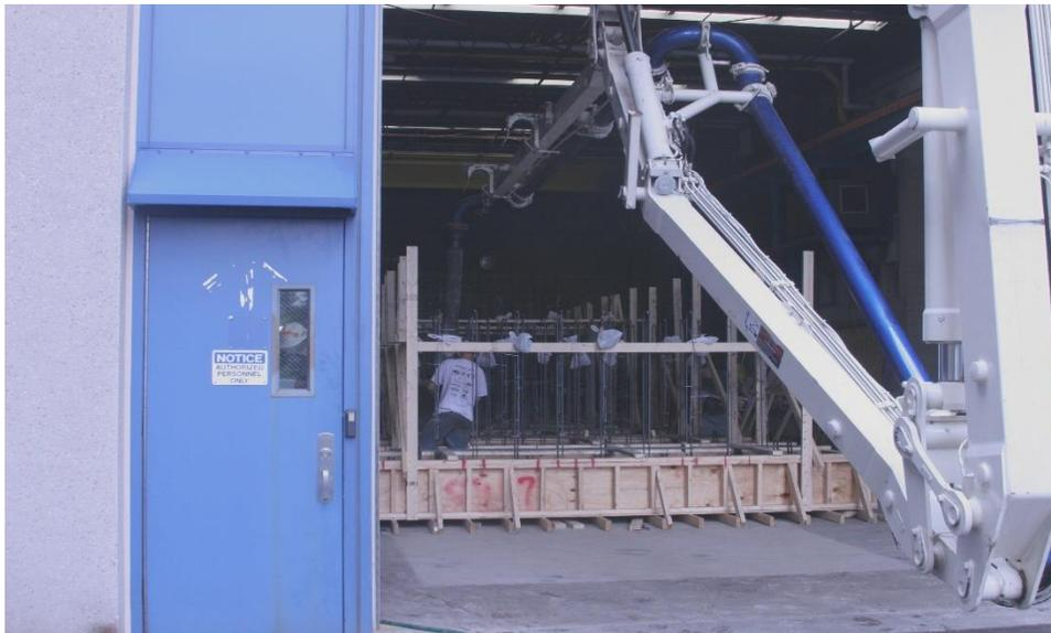
Figure 3.5. Pumping of concrete for Phase I foundations
