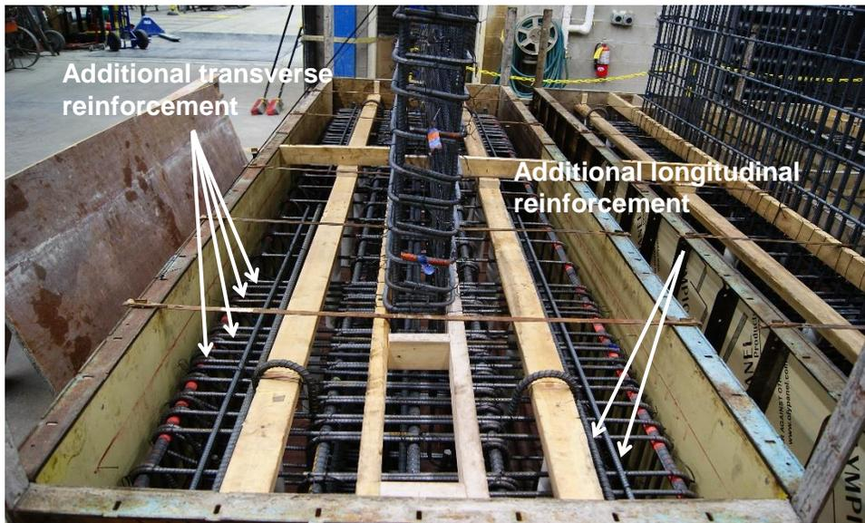
Figure 3.10. Supplemental reinforcement in the foundation of SW8
