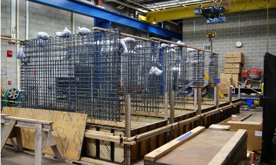
Figure 3.12. Phase II walls prior to foundation concrete casting
