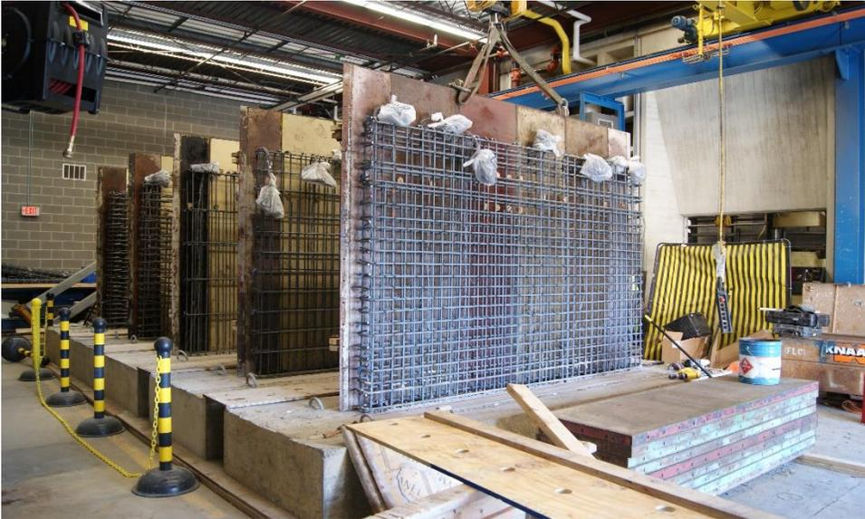
Figure 3.13. Installation of Phase II wall formwork
