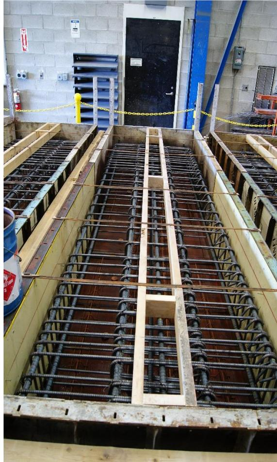
Figure 3.8 Foundation formwork and rebar cage for a Phase II wall
