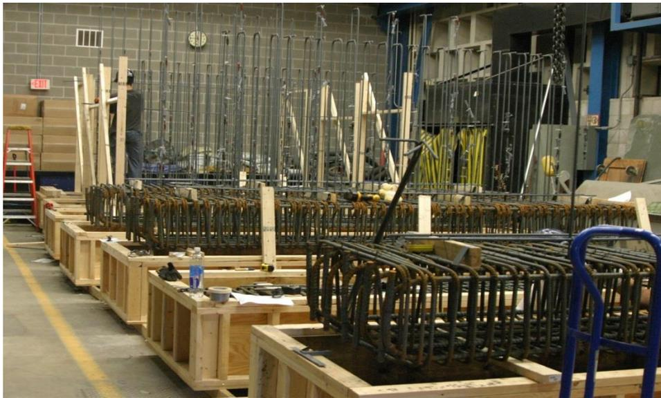
Figure 3.3. Phase I rebar cages prior to placement in formwork
