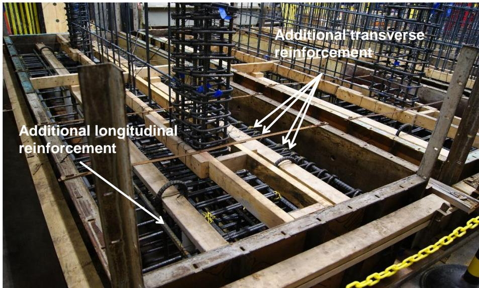
Figure 3.11. Supplemental reinforcement in the foundation of SW12
