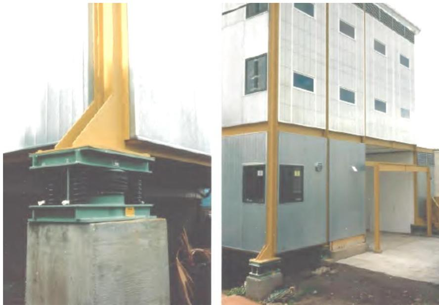
**Figure 1-8 3D Seismic Isolation System for a House in California (Makris and Constantinou, 1992)**
