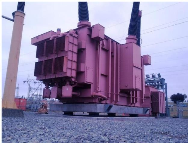
**Figure 2-1 Seismically Isolated Transformer in Vancouver, WA (courtesy L. Kempner, BPA)**
