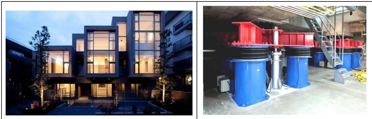
**Figure 1-7 Seismic Isolation System of Chisuikan Building (Tomizawa et al, 2011; Mori et al, 2012)**
