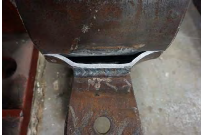
Figure 6-72 Failure section of the CHS for specimen D9.625L6-1
