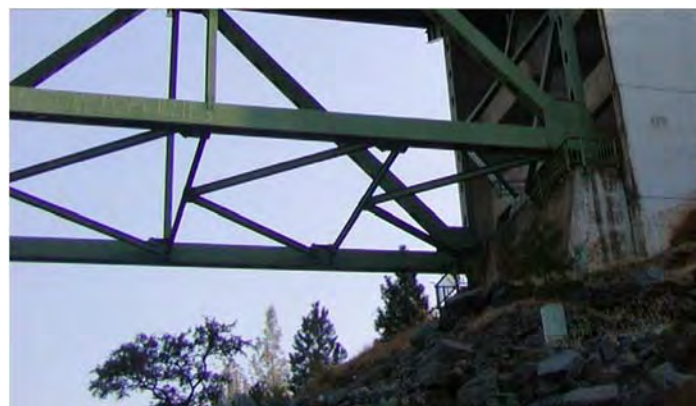
Figure 2-29 Lower Horizontal Bracing Near Abutment
