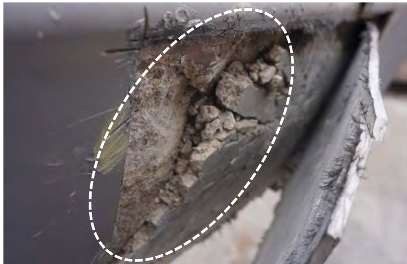
Figure 9-3 Concrete fractured around the broken core plate of BRB-2-4
