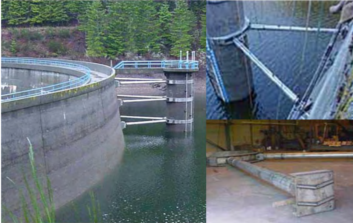
Figure 2-37 BRBs Installed in Casad Dam (Star Seismic, 2016b)
