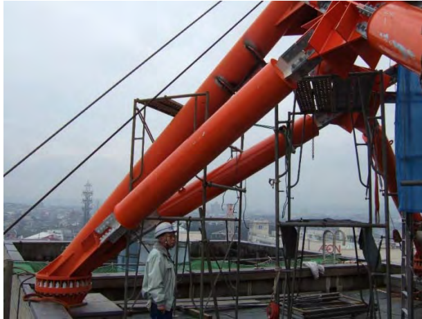
Figure 2-35 Close Look of BRBs Installed in the Communication Tower (Courtesy of Ian Aiken, Seismic Isolation Engineering, Emeryville, California)
