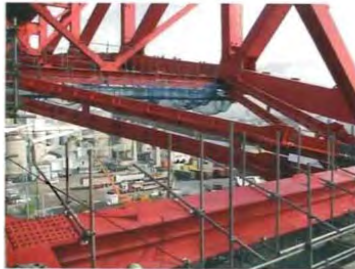
Figure 2-25 BRB Installed in the Bridge (Hamada et al., 2007)
