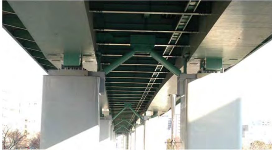
Figure 2-33 BRB application in transverse ductile diaphragm (Courtesy of H.B.Ge, Meijo University, Japan)
