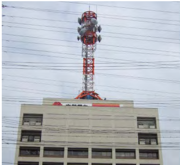
Figure 2-34 A Telecommunication Tower in Japan (Courtesy of Ian Aiken, Seismic Isolation Engineering, Emeryville, California)
