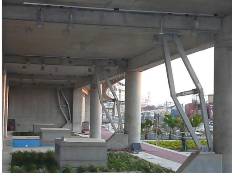
**Figure 1-2 Installation of Scissor-Jack-Damper System with Open Space and Large Angle of Inclination (image by Michael C. Constantinou)**
