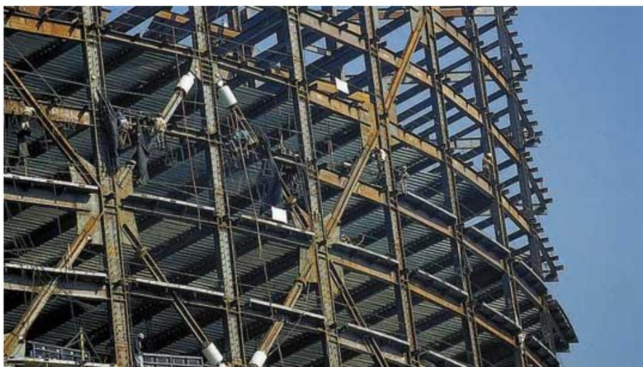
**Figure 1-3 Coupled Truss and Damping Mechanism in Torre Mayor building in Mexico**
