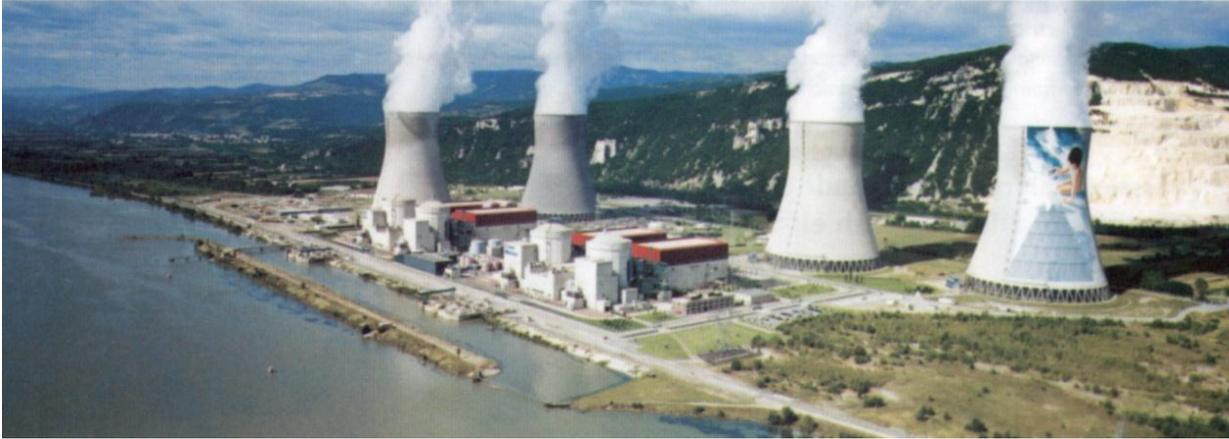
**Figure 2.3: Four units of seismically isolated NPP at Cruas, France (Forni and Poggianti, 2011)**
