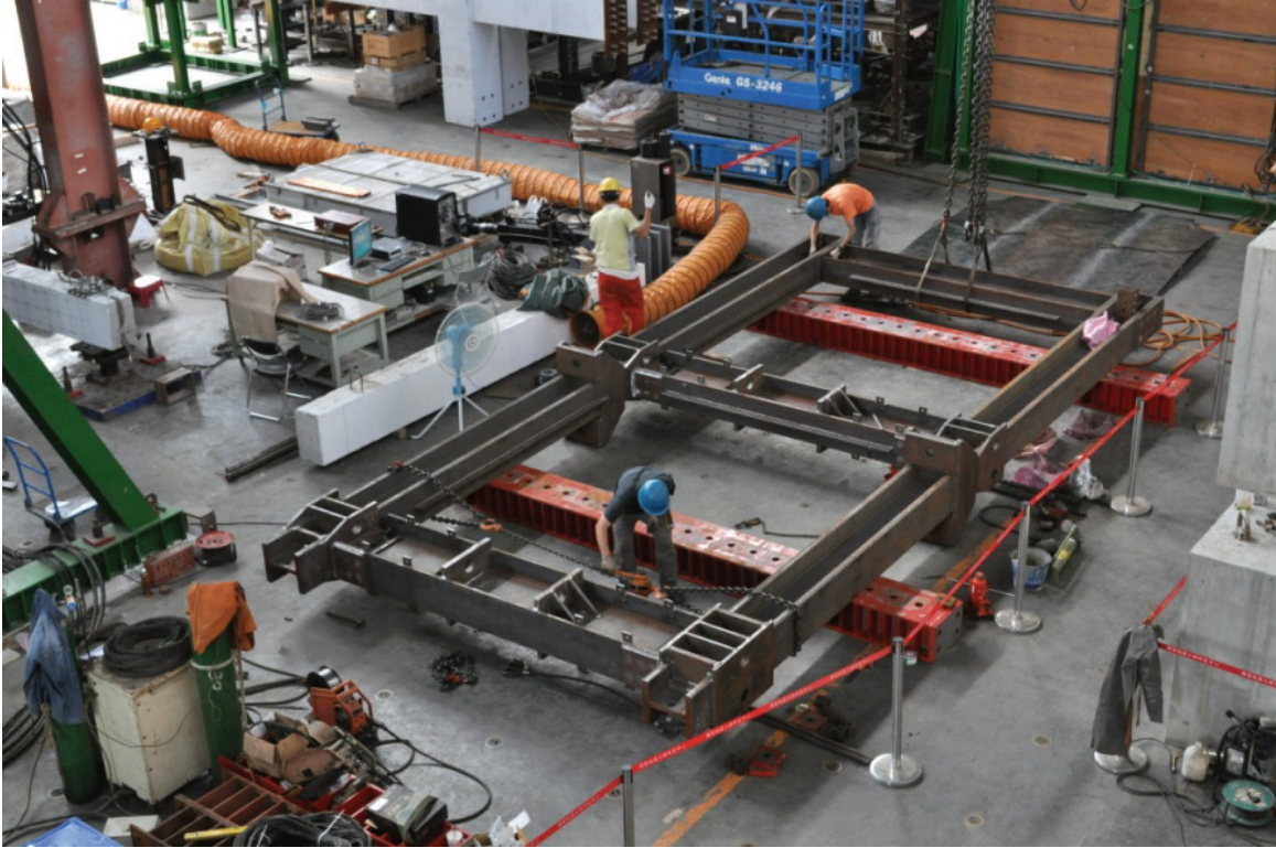
FIGURE 9-1a Specimen NZ construction: Step 1 – assemble boundary frame
