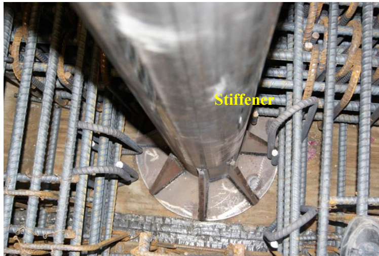
Figure 4-24 Stiffened Annular Ring and CFSSP-Wall Positioning
