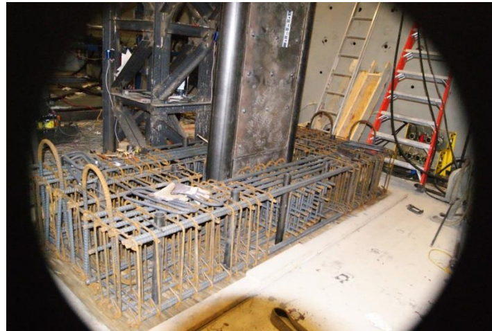
Figure 4-26 Final Assembly for the Foundation Re-bars
