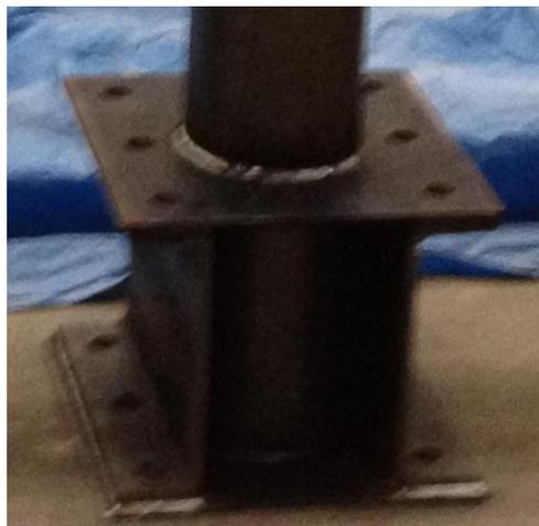
**Figure 4- 13 Circular Welding of the Additional Elements to the Column's Base**
