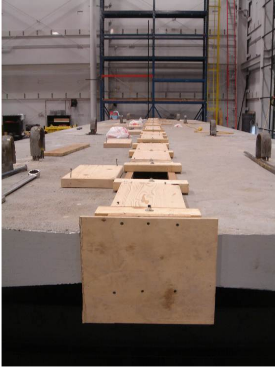
(a) Preparation of wood form
