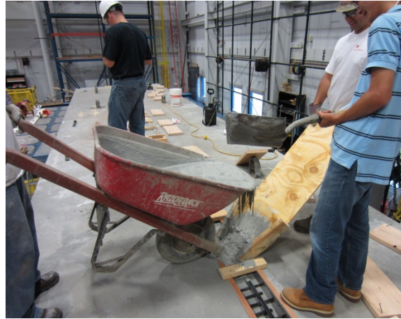
(b) Casting UHPC
