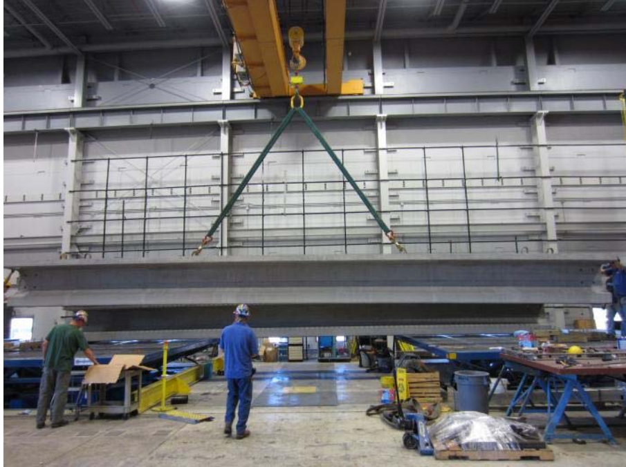
(b) Lifting of the DBT girder 2
