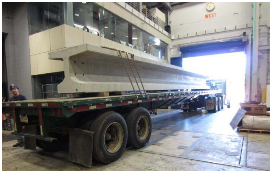
(a) Delivery of the DBT girder 1
