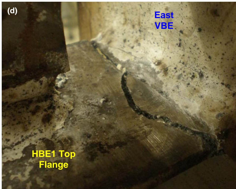
Figure 4-32 Boundary Frame Final Condition – Cont'd: (c) Fracture at HBE1 Top Flange (North View); (d) Fracture at HBE1 Top Flange (South View)
