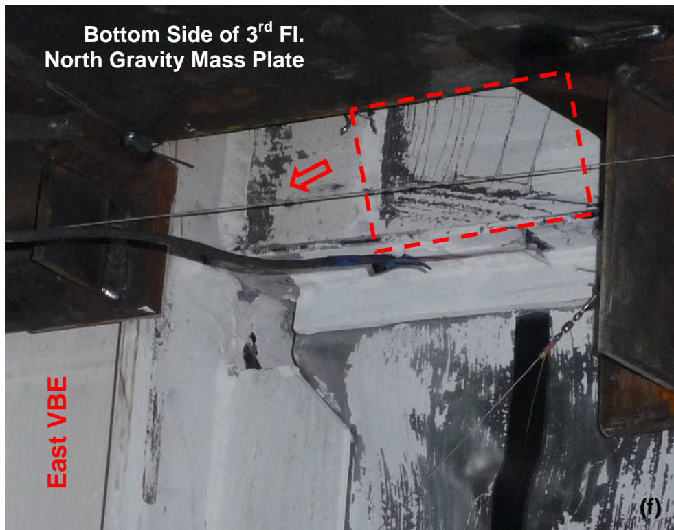
Figure 4-15 Specimen Condition at the End of Displacement Step 7b ( \Delta_3 = 4\delta_y = 1.88\% Drift) – Cont'd: (e) & (f) Yielding on HBE-to-VBE Connections
