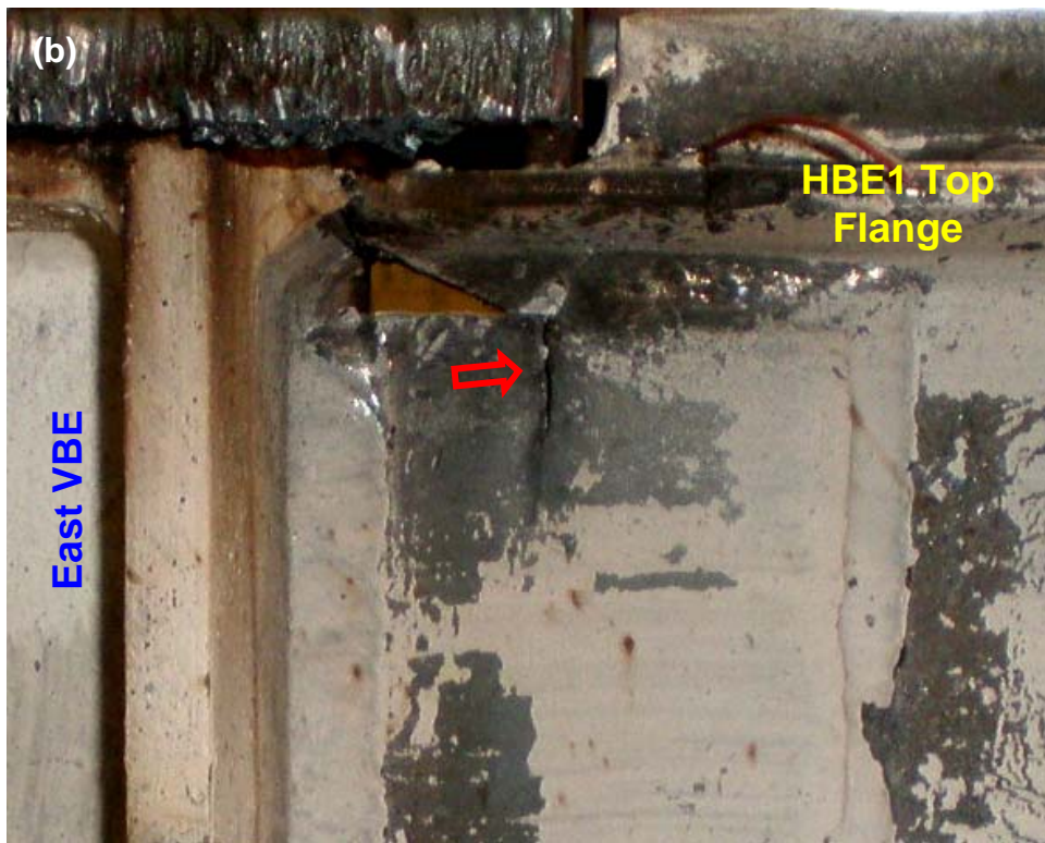
Figure 4-32 Boundary Frame Final Condition (Step 10d: \Delta_3 = 3.33\% Drift = 7.09\delta_y ): (a) Fracture at HBE2 Bottom Flange; (b) Shear Tab Fracture at HBE1
