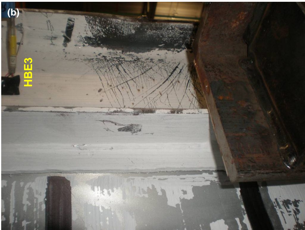
Figure 4-17 Yielding beneath HBE3 Connecting Angles in Displacement Step 8a ( \Delta_3 = 2.5\% Drift = 5.32\delta_y ): (a) Detail of West Side; (b) Detail of East Side
