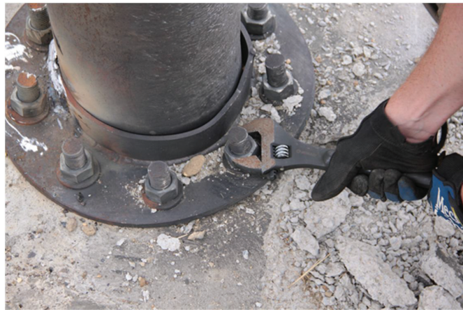
Figure 8-89: Loose Bolt Being Retightened on Specimen MSJC3
