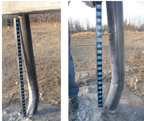
Figure 8-29: View of the Global Deformation of Specimen B1
