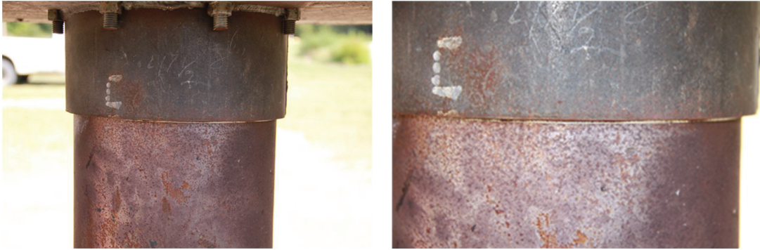
Figure 8-81: Evidence of Contact Between on Specimen MSJC2 and its Collar
