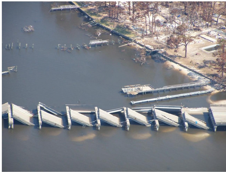
Figure 2-3: Span Unseating for Simple Span Bridge (MCEER, 2008)
