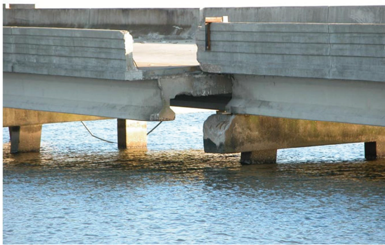
Figure 2-2: Shifting of Bridge Superstructure After Hurricane Katrina (MCEER, 2008)
