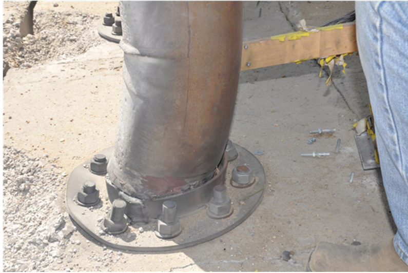
Figure 8-86: Damage to the Rulon Tape and Slip of Specimen MSJC1 over the Collar
