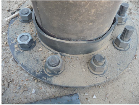
Figure 8-63: Deformation of Collar after Test 1 on Specimen MSJC1
