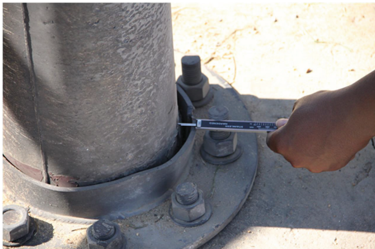
Figure 8-72: Collar Deformations Measured Using the Depth Probe of a Vernier Caliper
