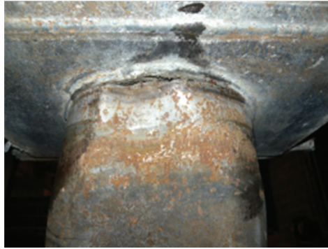
Figure 8-25: Crack in the Outside Tube at the Specimen to Foundation Beam Connection
