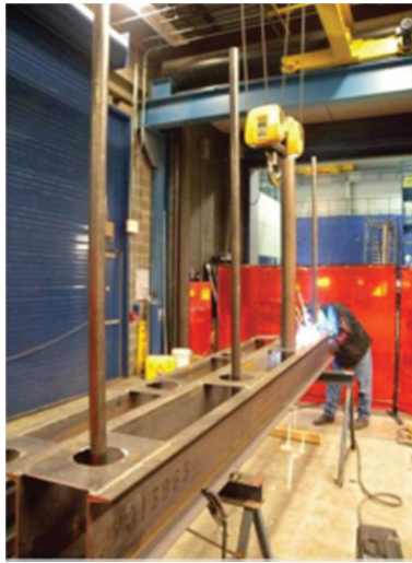
Figure 8-10: Outer Tube to Cap Beam Plates Connection
