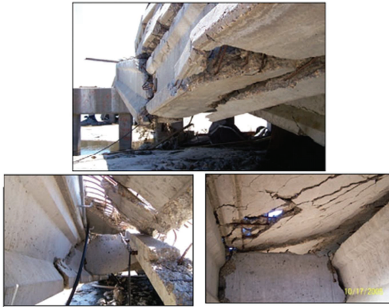
Figure 2-4: Failure of Prestressed Concrete Girder (Top) Accompanied by Diaphragm Failure (Bottom Left) and Deck Failure (Bottom Right) (MCEER, 2008)
