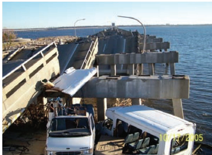
Figure 2-5: Debris Lodged Against a Bridge Bent (MCEER, 2008)
