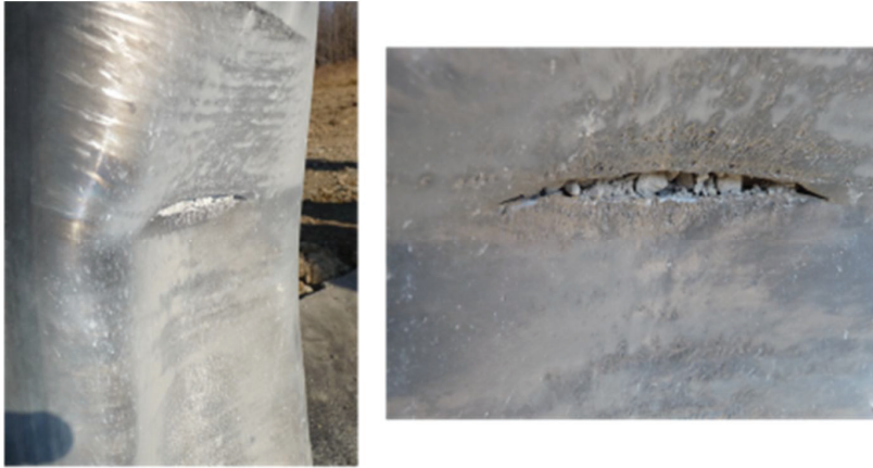
Figure 8-23: Crack in Specimen B7
