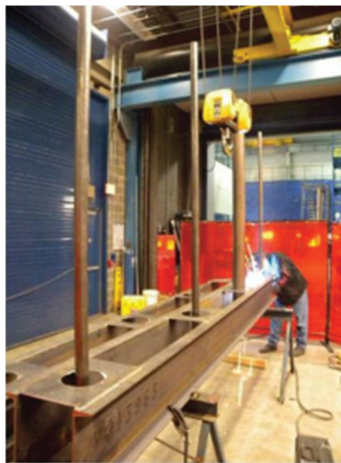
Figure 8-9: Inner Tube to Cap Beam Top Plate Welding
