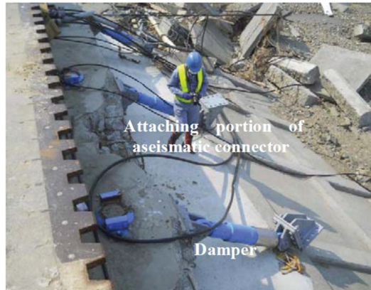
Figure 2-7: Damper Failure (J_BEC, 2011)
