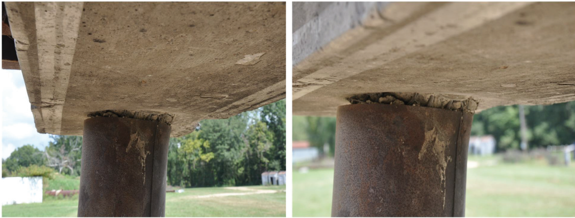
Figure 8-87: Widening of the Crack at the Top of Specimen MSJC1
