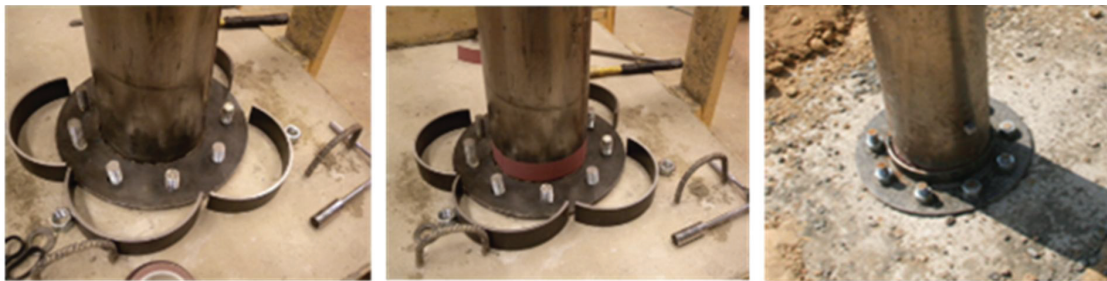
Figure 8-49: Steel Collar: Components (Left and Middle) and Construction (Right)
