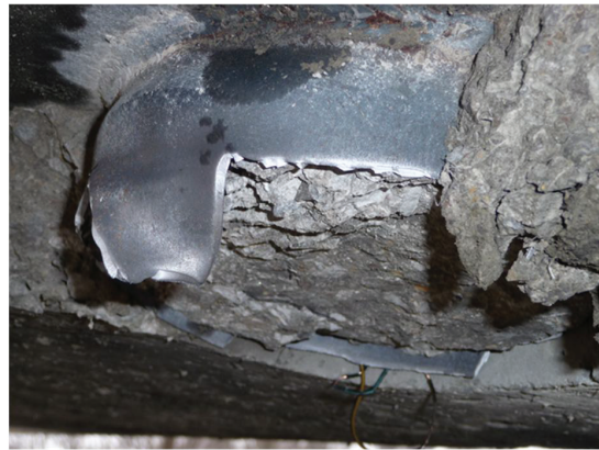
Figure 8-37: Tear of Specimen B8 from the Cap Beam
