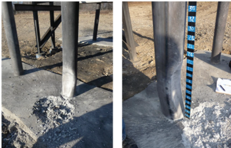
Figure 8-24: Overview of the Deformations of Specimen B7
