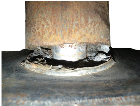
Figure 8-39: Fracture at the Base of Specimen B2
