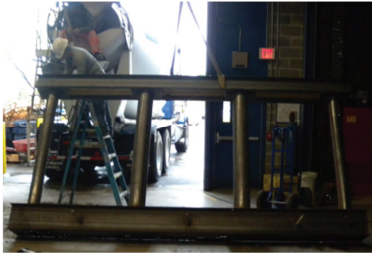
Figure 8-13: Concreting of the CFDST Columns
