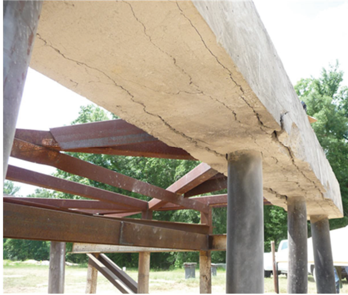
Figure 8-58: Longitudinal Crack Underneath the Cap Beam
