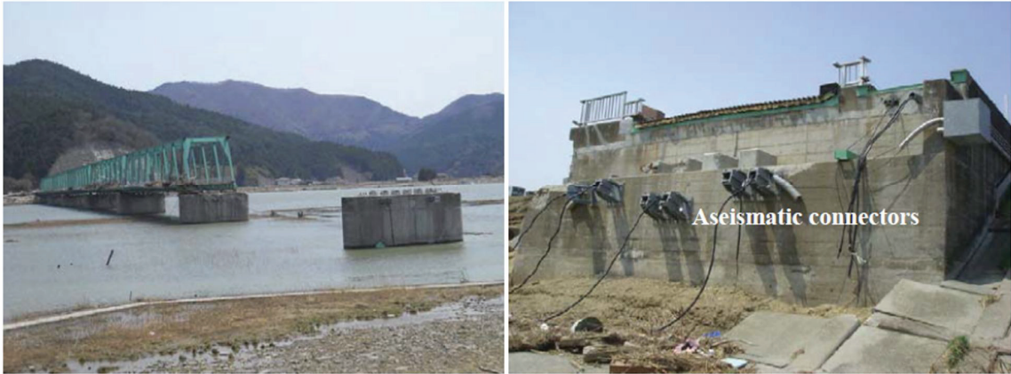
Figure 2-8: Washed Away Truss Bridge Span (J_BEC, 2011)
