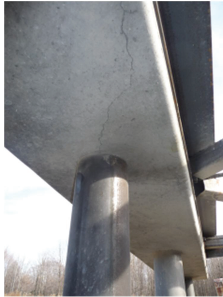
Figure 8-21: Crack in the Cap Beam in the Vicinity of B4
