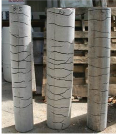
Figure 8-95: Crack Pattern in the Upper Part Specimens B5 (Left), B6 (Middle) and B1 (Right)
