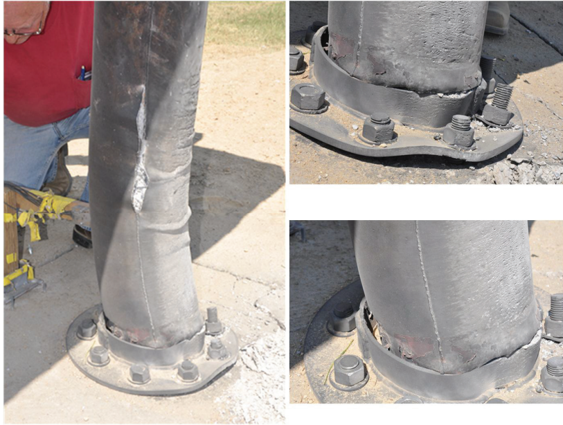
Figure 8-85: Seam Failure of Specimen MSJC1 and Base Deformation
