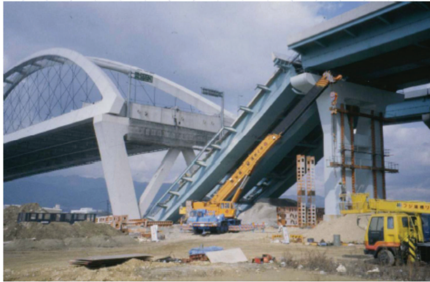
Figure 2-1: Example of Bridge Unseating (Priestley, et al., 1996)
