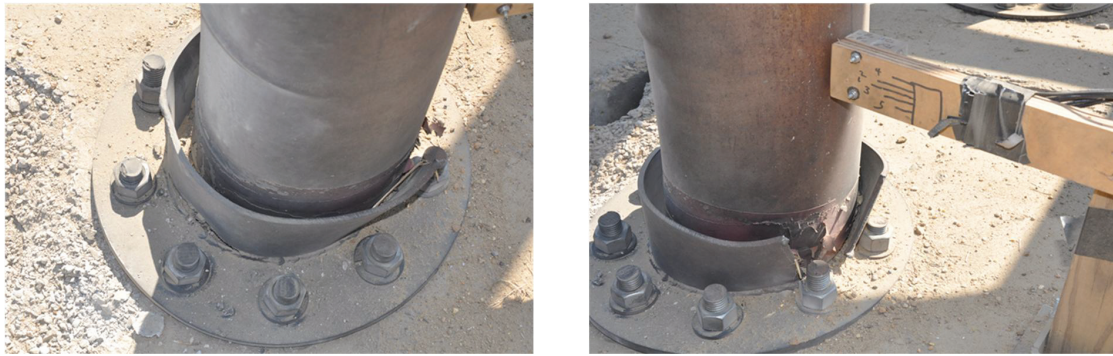
Figure 8-79: Post-shot Failure of the Collar on Specimen MSJC2
