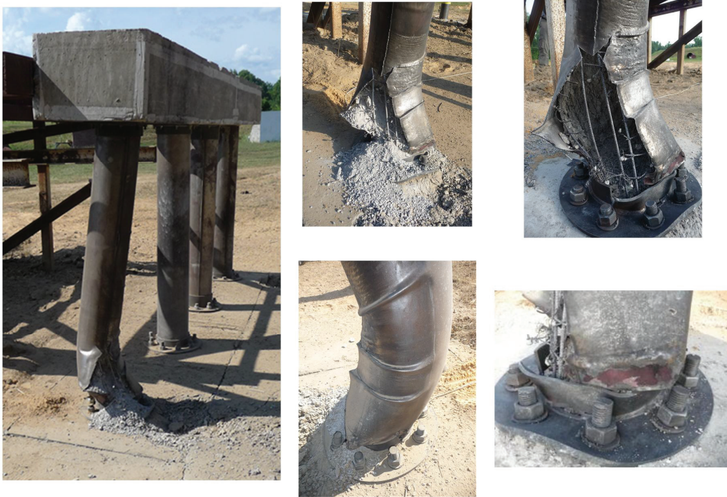
Figure 8-67: Global View and Close-up of the Base of MSJC4 After the Test
