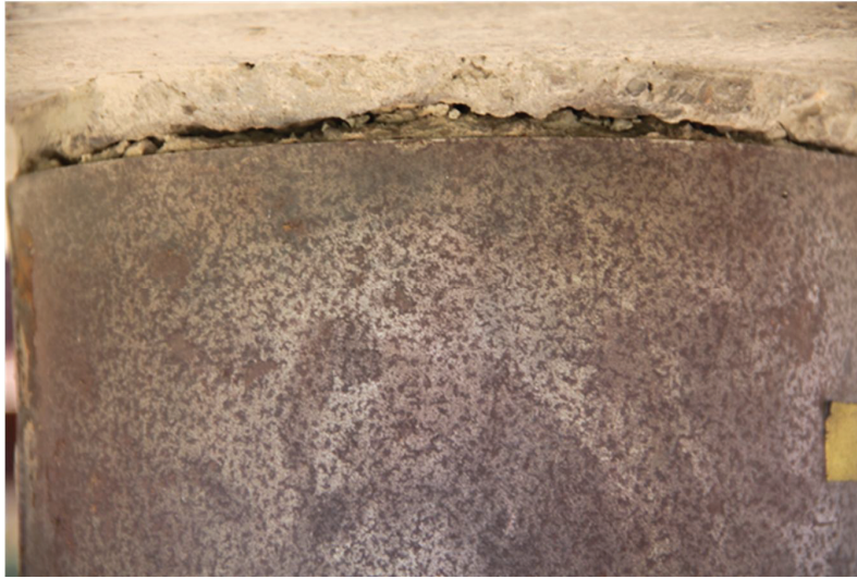
Figure 8-73: Widening of the Pre-existing Crack at the Top of Specimen MSJC1
