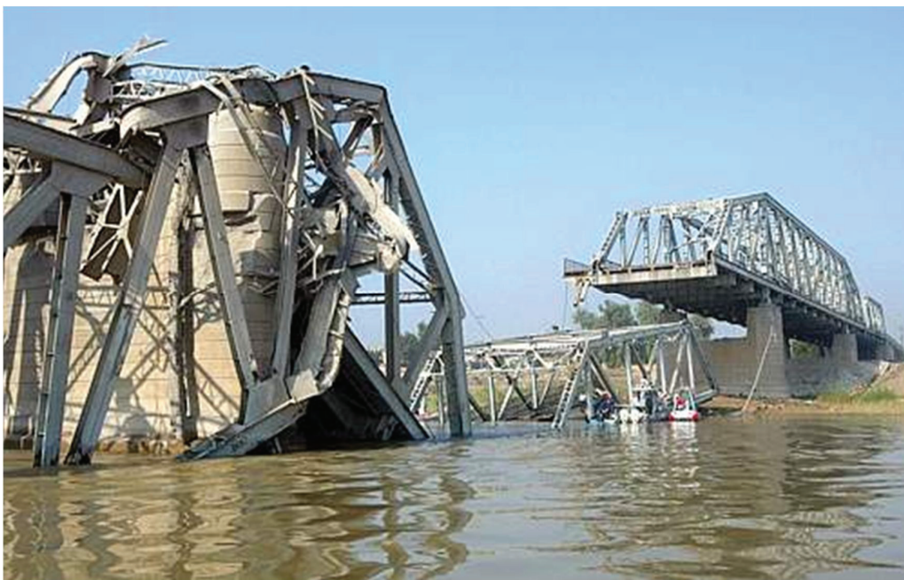
Figure 2-23: Structural damage to Truss Bridge Due to Explosion at the Deck Level (Bridge on the Tigris River, Iraq, AFP, 2007)
