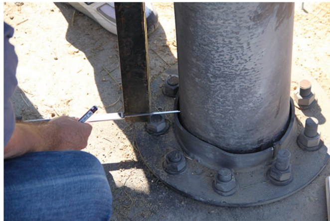
Figure 8-70: Inward Deformation of the Collar in the Front of Specimen MSJC1
