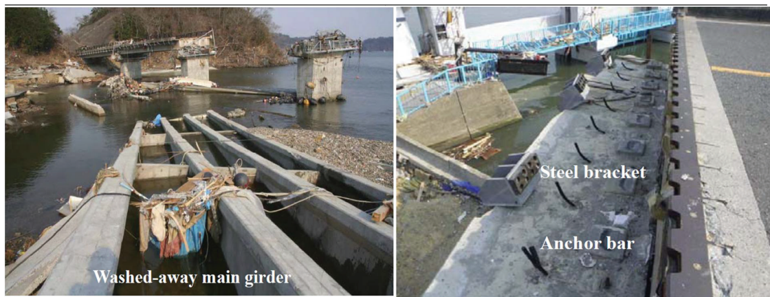
Figure 2-6: Deck and Brackets Failure (J_BEC, 2011)
