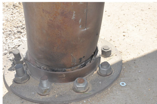
Figure 8-84: Mark on the Steel Jacket Resulting From Bearing on the Collar
