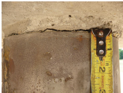
Figure 8-62: Crack at the Top of Specimen MSJC1
