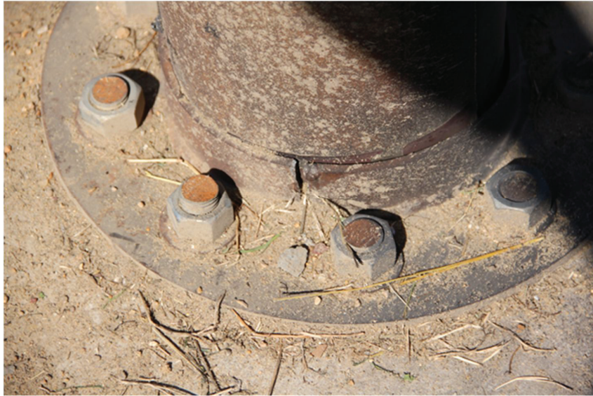
Figure 8-71: Crack in the Collar of MSJC1 at Weld Connection
