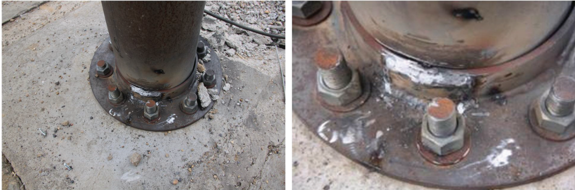
Figure 8-88: Repair of the Bottom Collar Fracture of Specimen MSJC3
