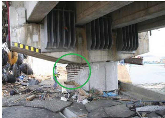
Figure 2-9: Crushing of Concrete at the Column to Cap Beam Connection (J_BEC, 2011)
