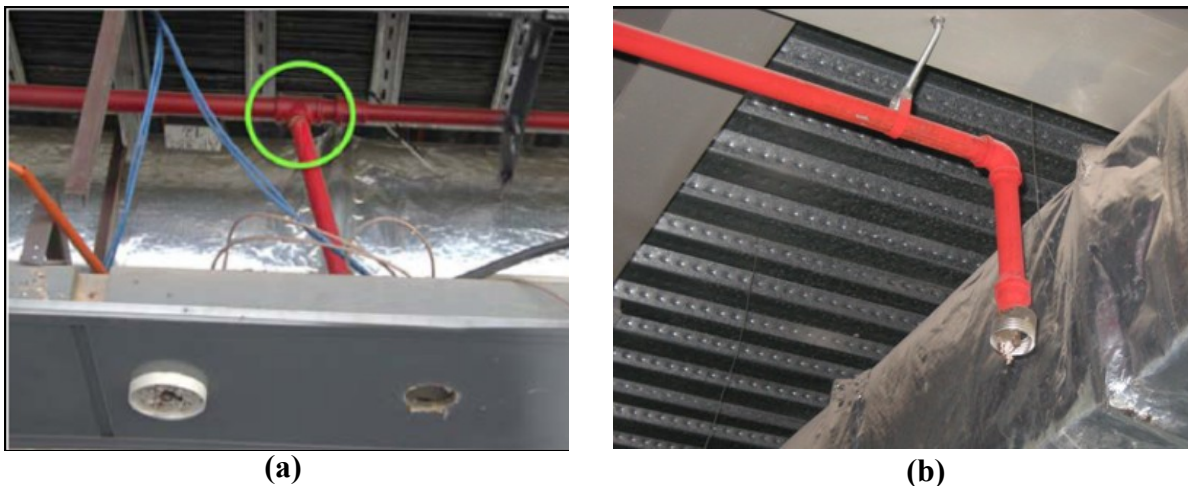
Figure 1-5 (a) Failures of Water Sprinkler Piping Near Joints (Miranda et al. 2012). and (b) Permanent Offset of Pipe Hanger (Photo: P. Correa)
