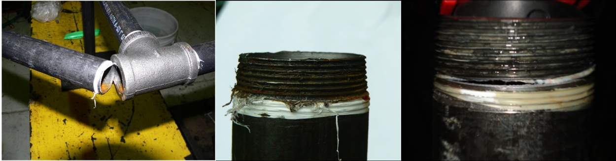
Figure 2-3 Observed Damage in Threaded Tee Joints (Tian et al., 2012)
