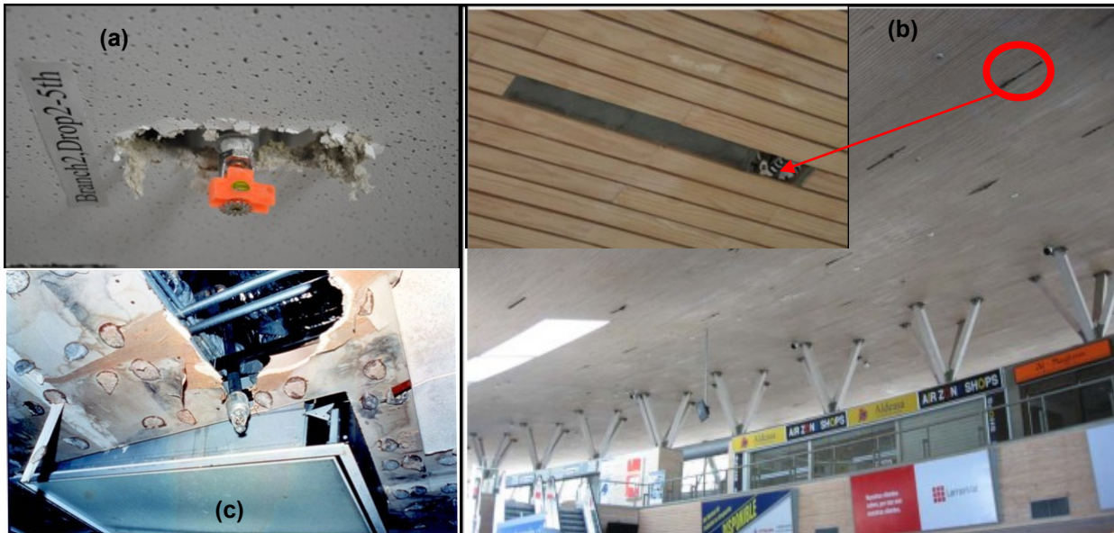
Figure 7-2 Damage Caused by Sprinkler Head-Ceiling Interaction, Photo courtesy of; (b) Rodrigo Retamales, Rubn Boroschek & Associates (c) Robert Reitherman
