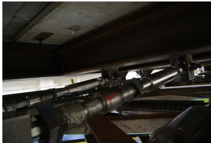
Figure 3.11. Two viscous dampers installed as part of isolation system
