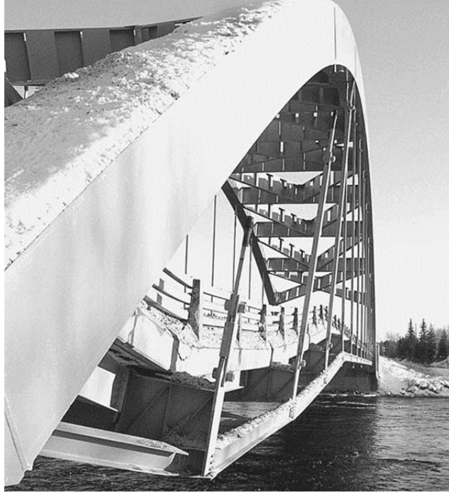
Figure 3-12: Distress of Sgt. Aubrey Cosens V.C. Memorial Bridge
