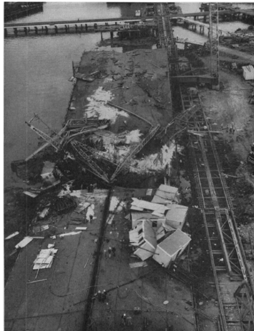
Figure 3-10: Collapse of the West Gate Bridge during Construction
