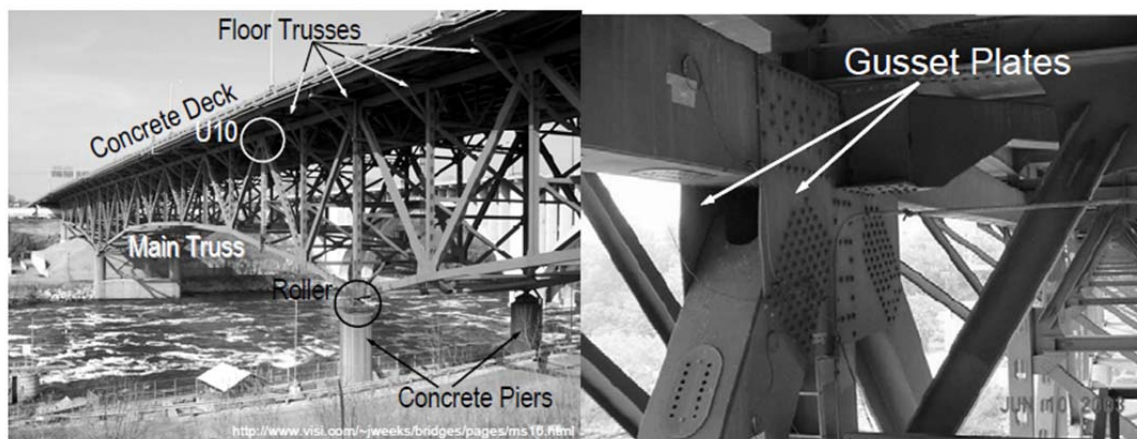
Figure 3-6: Structure of the I-35W Bridge over the Mississippi River in Minneapolis
