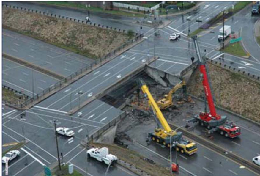
Figure 3-8: Concorde Overpass Partial Collapse
