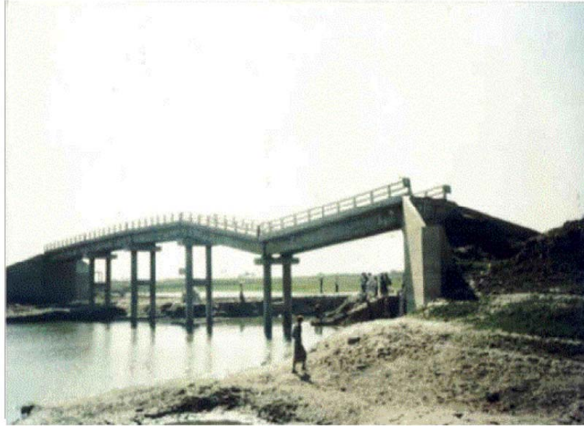
Figure 3-20: Failure of Turag-Bhakturta Bridge
