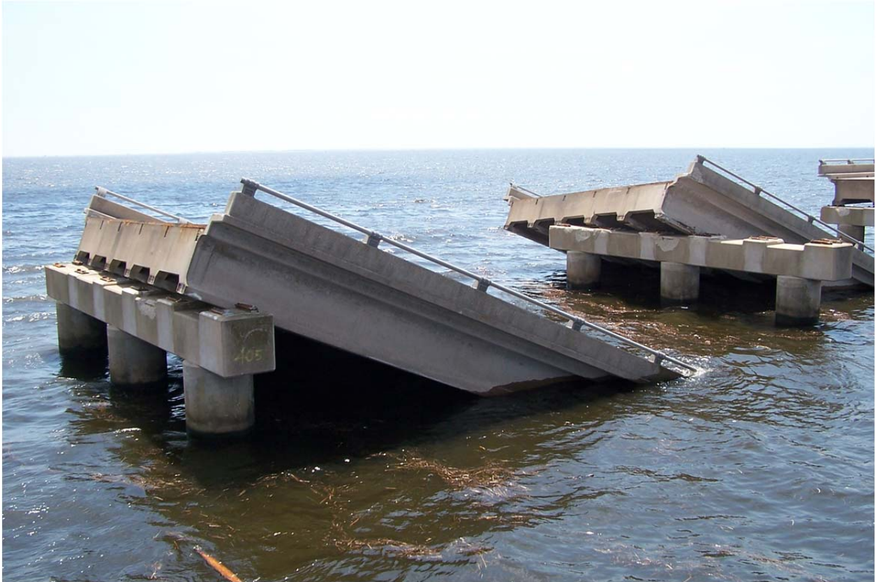
Figure 3-26: Spans of the Interstate 10 Twin Bridge were dropped off by Hurricane Katrina
