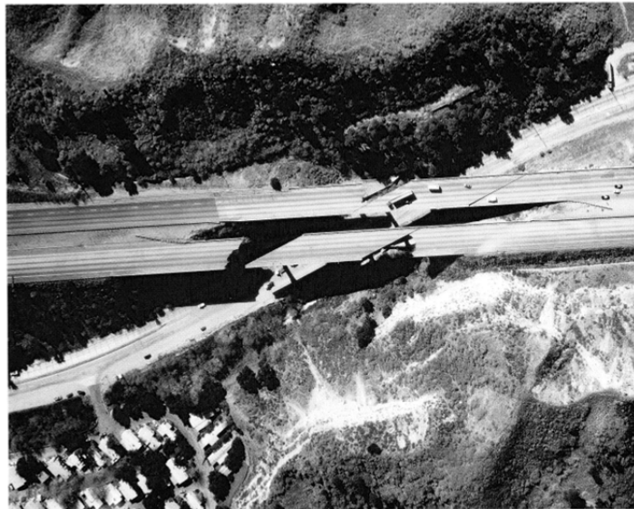
Figure 3-16: Collapsed Gavin Canyon Undercrossing (Source: Buckle 1994) [223]
