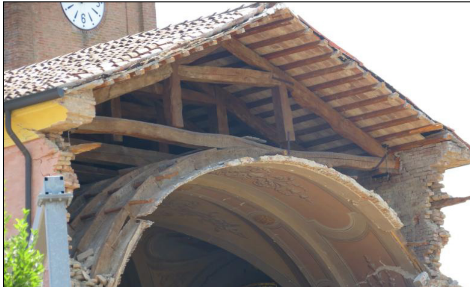
Figure 7-18 Example of roof structure made of timber trusses
