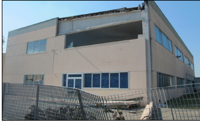
Figure 6-46 Detachment of horizontal panels (Mirandola)
