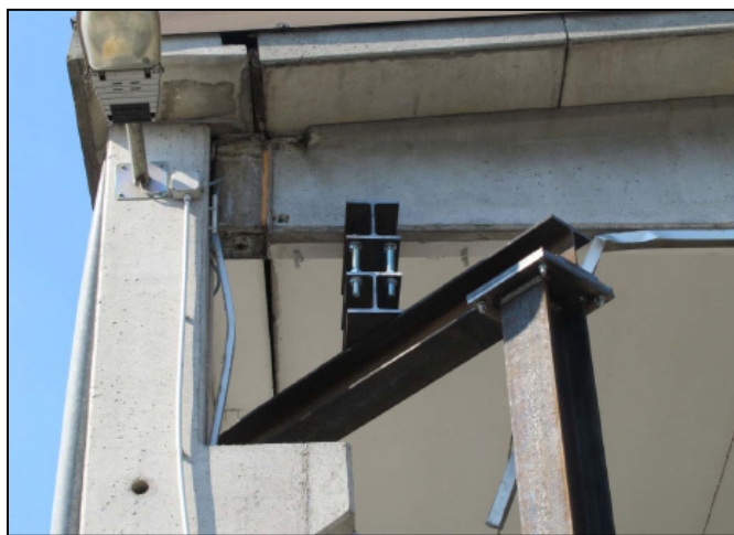
Figure 6-26 Emergency intervention to avoid collapse of the industrial shed due to beam slippage
