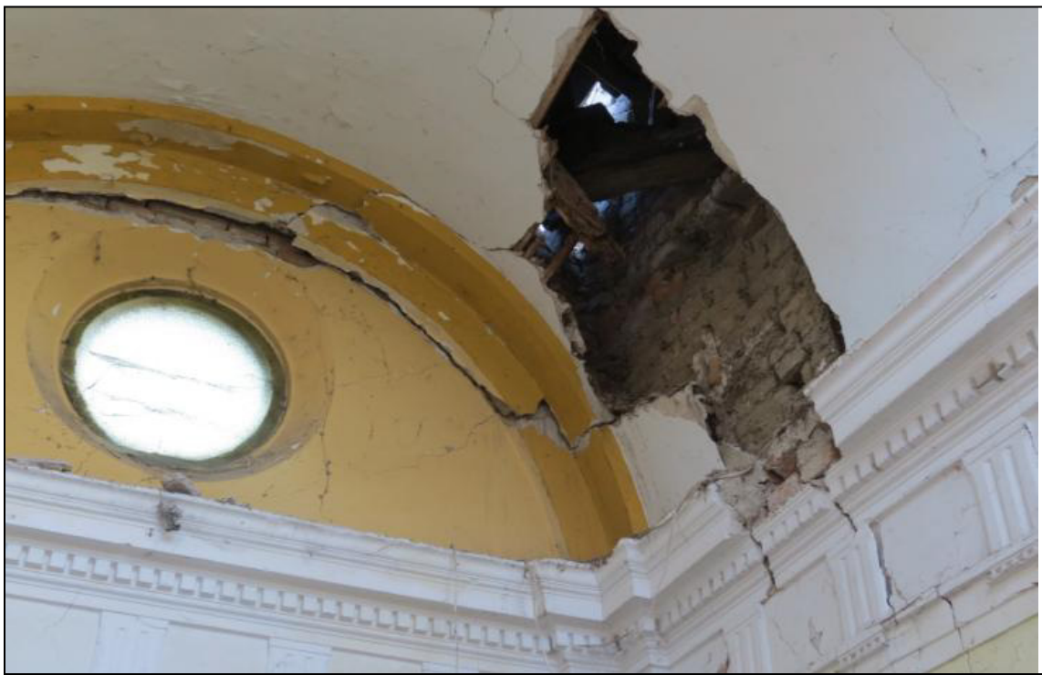
Figure 7-22 Example of vault made of timber elements imbedded in mortar/plaster
