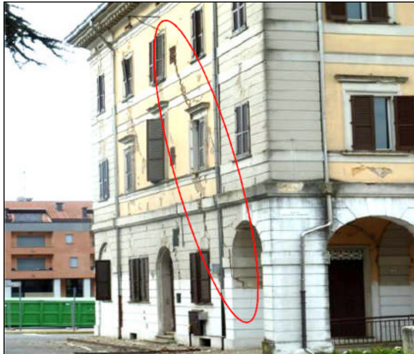
Figure 7-67 Large and extensive crack in a side wall
