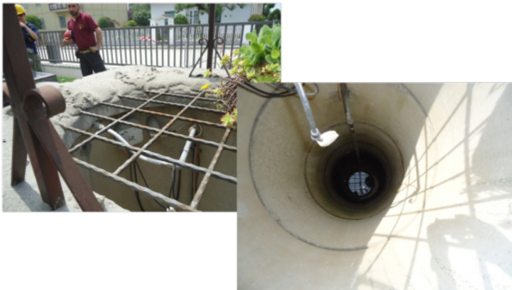
Figure 5-6 Aquifer level in the wells in San Carlo (Sant'Agostino)
