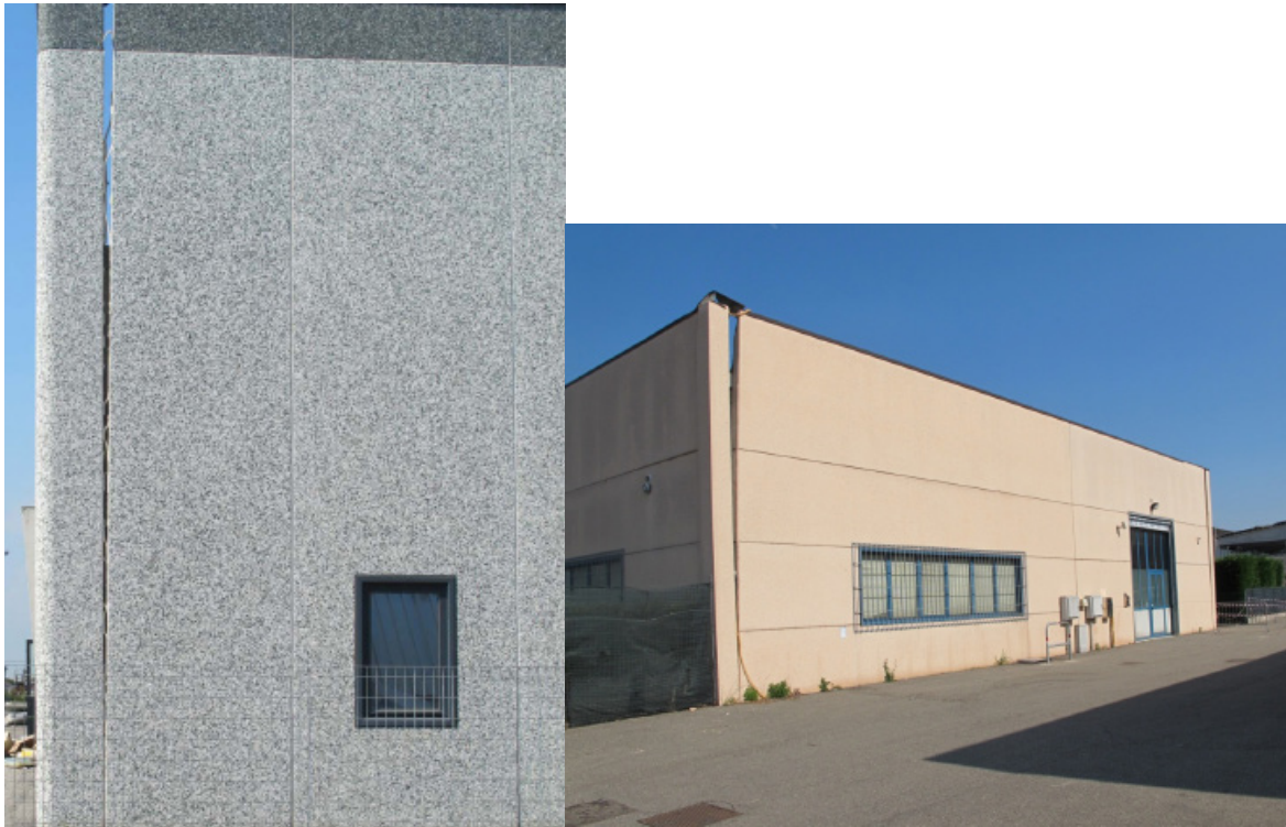
Figure 6-40 Vertical panels behave properly when connected at the base
