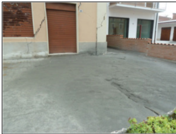
Figure 4-3 Damage to a residential building in San Carlo due to soil liquefaction
