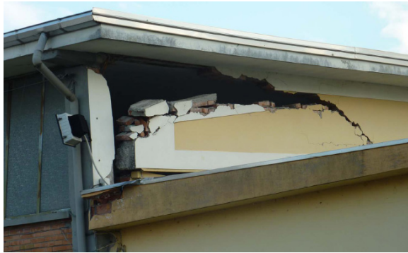
Figure 6-28 (a) Overview (b) Failure of out of plane claddings in Sant'Agostino
