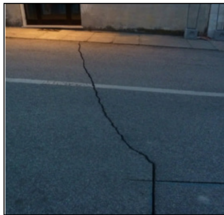
Figure 9-4 Cracking phenomena in a road in Mirabello
