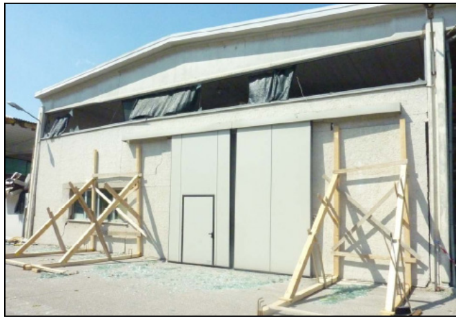
Figure 6-13 Panels without connection with the main structural frame CF
