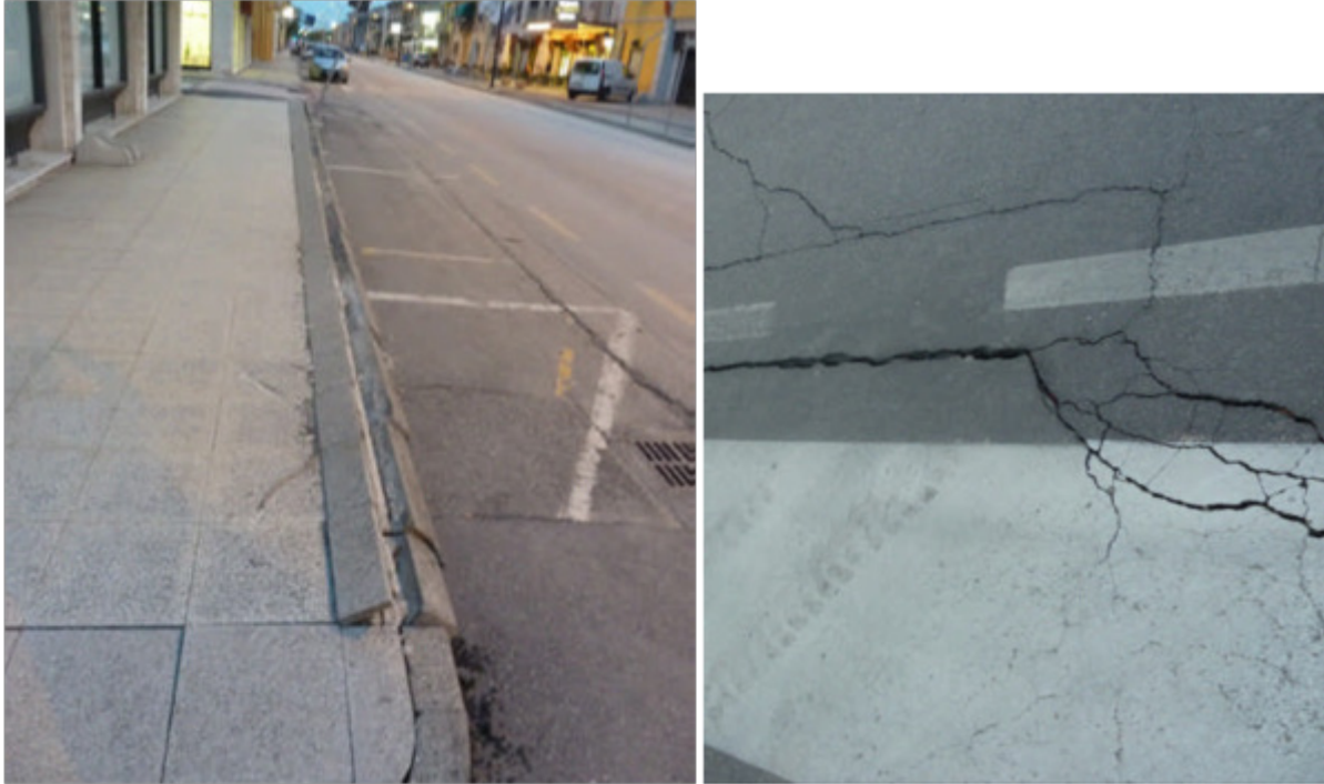
Figure 4-2 Evidence of lateral spreading in the street in Mirabello
