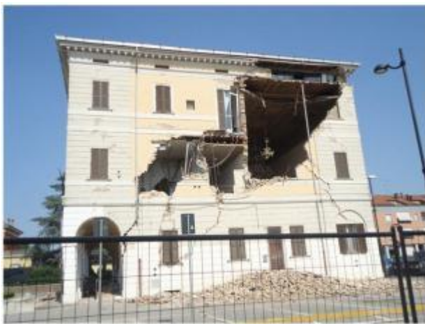
Figure 7-65 Partial collapse of the side wall and loss of the connection to the external wall in the front
