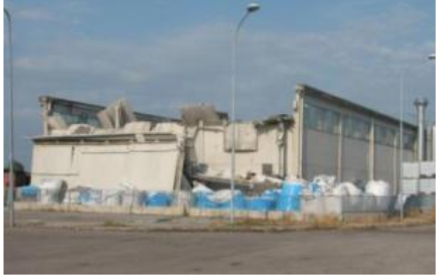
Figure 6-32 Recent industrial sheds with internal collapse
