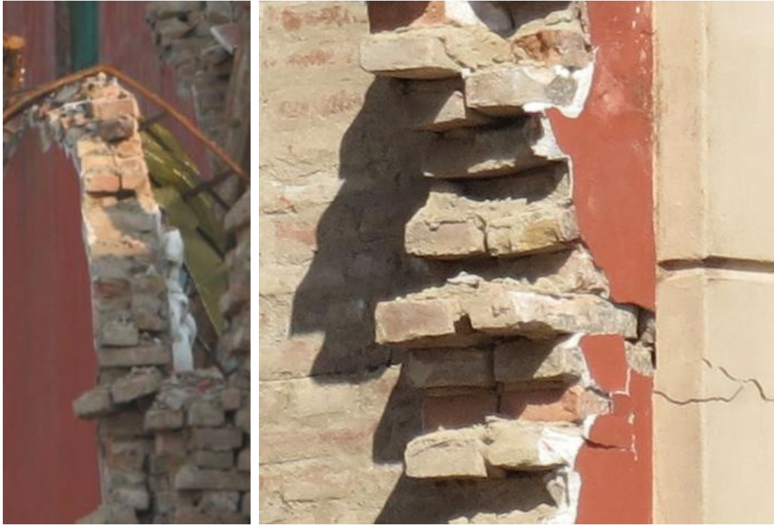
Figure 7-10 Double header brick masonry bond
