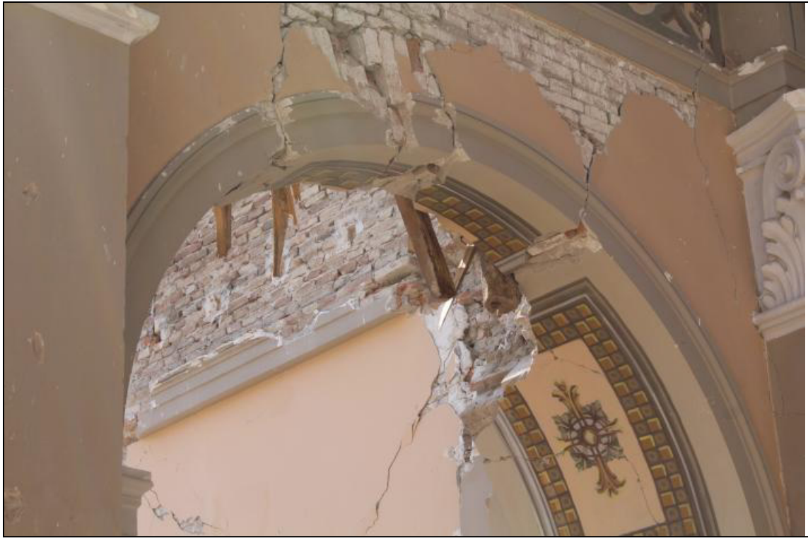
Figure 7-23 Example of arches made of vertically stacked brick masonry
