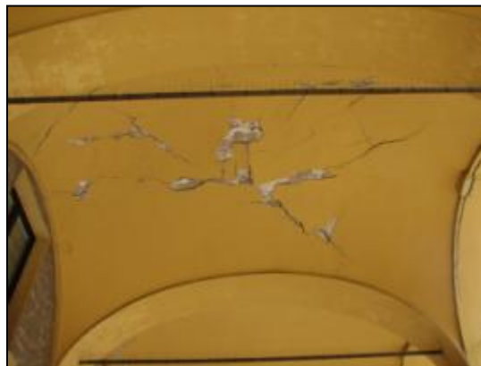
Figure 7-72 Vault damaged by floor failure
