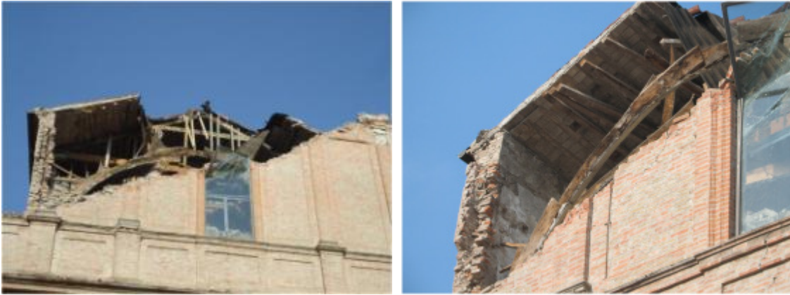
Figure 7-54 Collapsed roof
