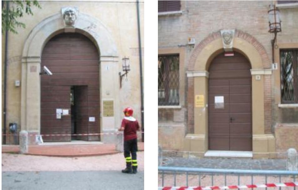
Figure 7-84 Entrance to the library (left), and archive entry (right)
