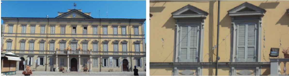
Figure 8-3 Façade of Corbelli Palace and cracked walls
