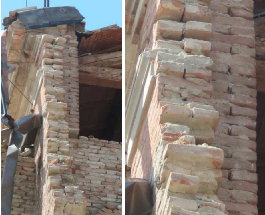
Figure 7-12 Double wall made of double header brick masonry bond
