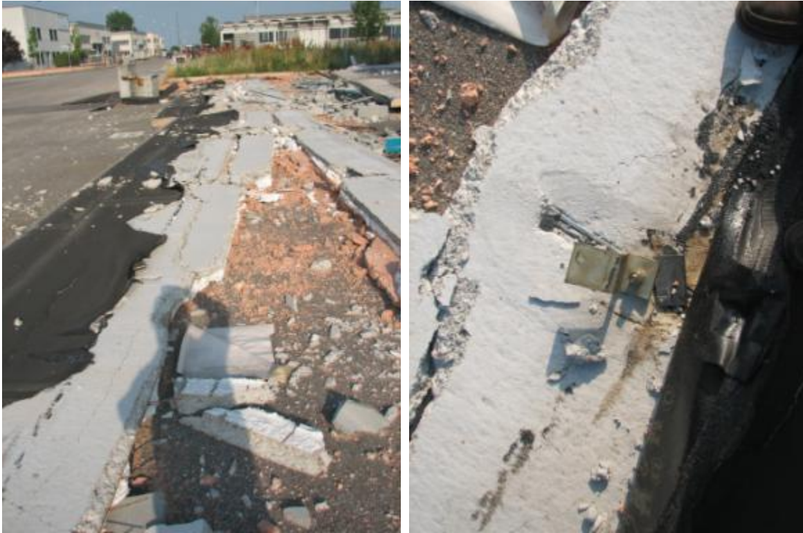
Figure 6-44 Collapse of horizontal panels due to insufficient connections to the beams
