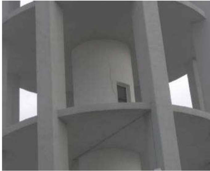
Figure 9-1 Water tank in San Carlo and localized crack in the interior reinforced concrete core
