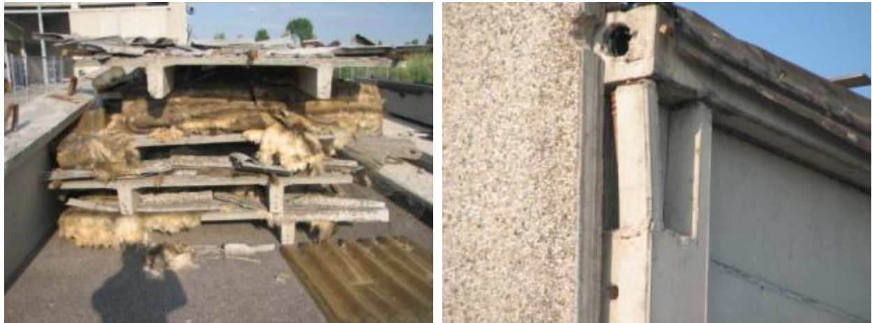
Figure 6-38 (a) Remains of the collapsed roof; (b) failure of shear key due to lack of reinforcement
