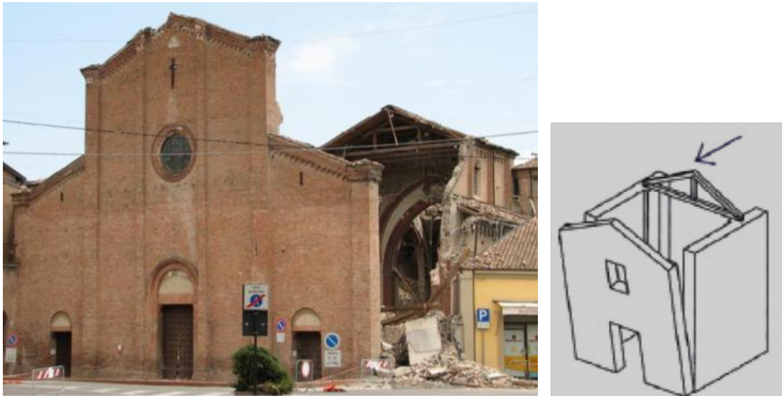
Figure 7-36 San Francis Church in Mirandola after the earthquake and critical mechanism
