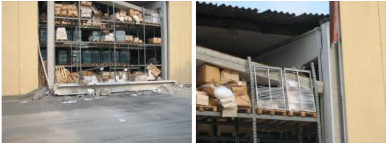
Figure 6-8 Roof collapse due to the movement of the vertical panels hung from the roof cover (Mirandola)
