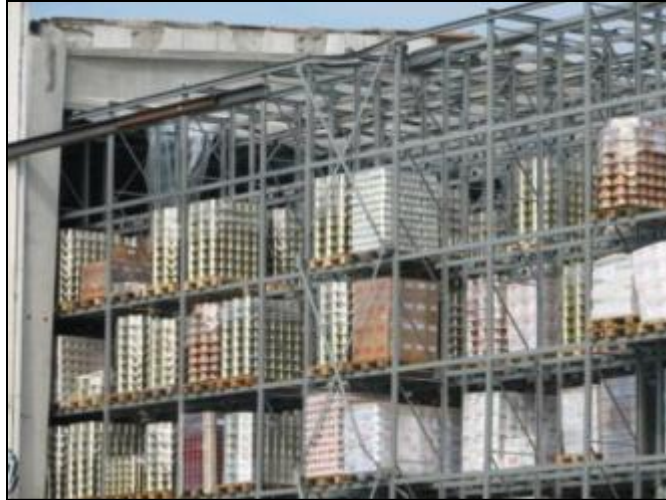
Figure 6-62 Detail of the internal scaffolds
