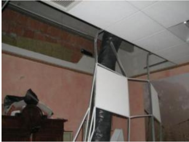
Figure 6-64 Broken suspended ceiling tile
