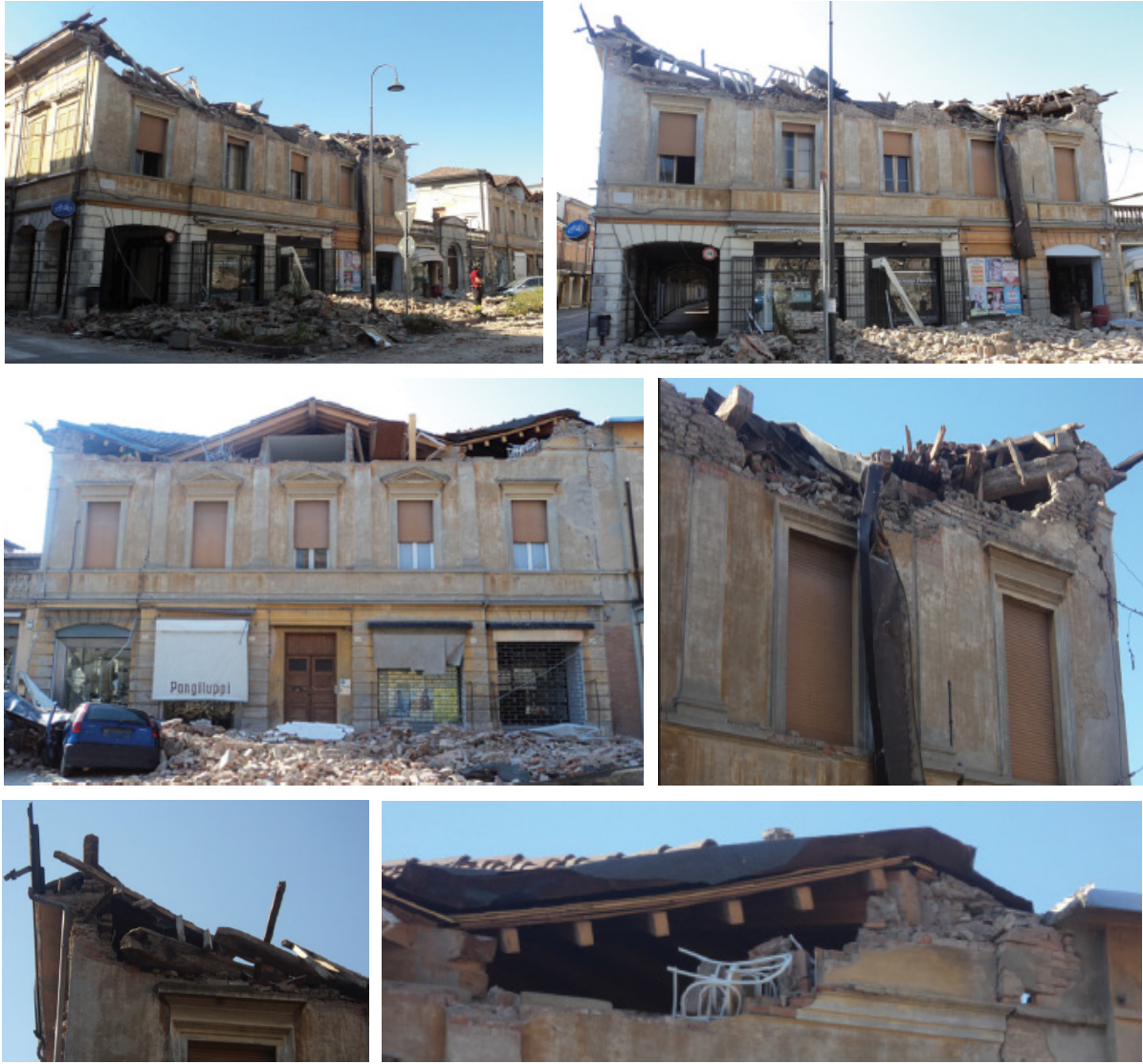
Figure 8-5 Damage to the post office building
