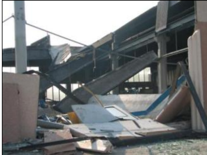
Figure 6-35 Longitudinal toppling of beams for displacement limit
