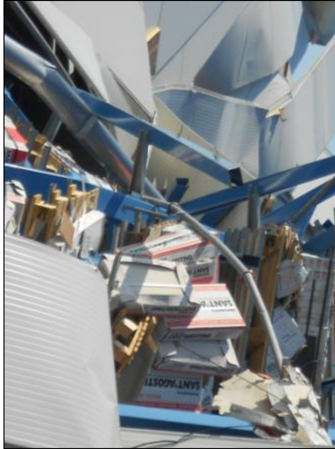
Figure 6-60 Warping failure effects of U-shaped sections
