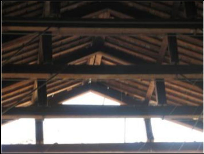
Figure 7-17 Example of roof structure made of timber trusses
