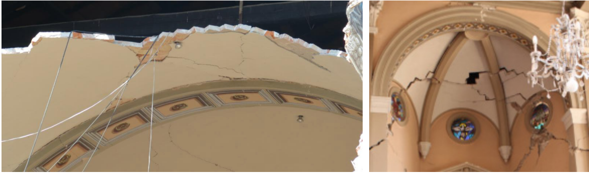
Figure 7-20 Example of vault structure made of brick masonry laid flatwise
