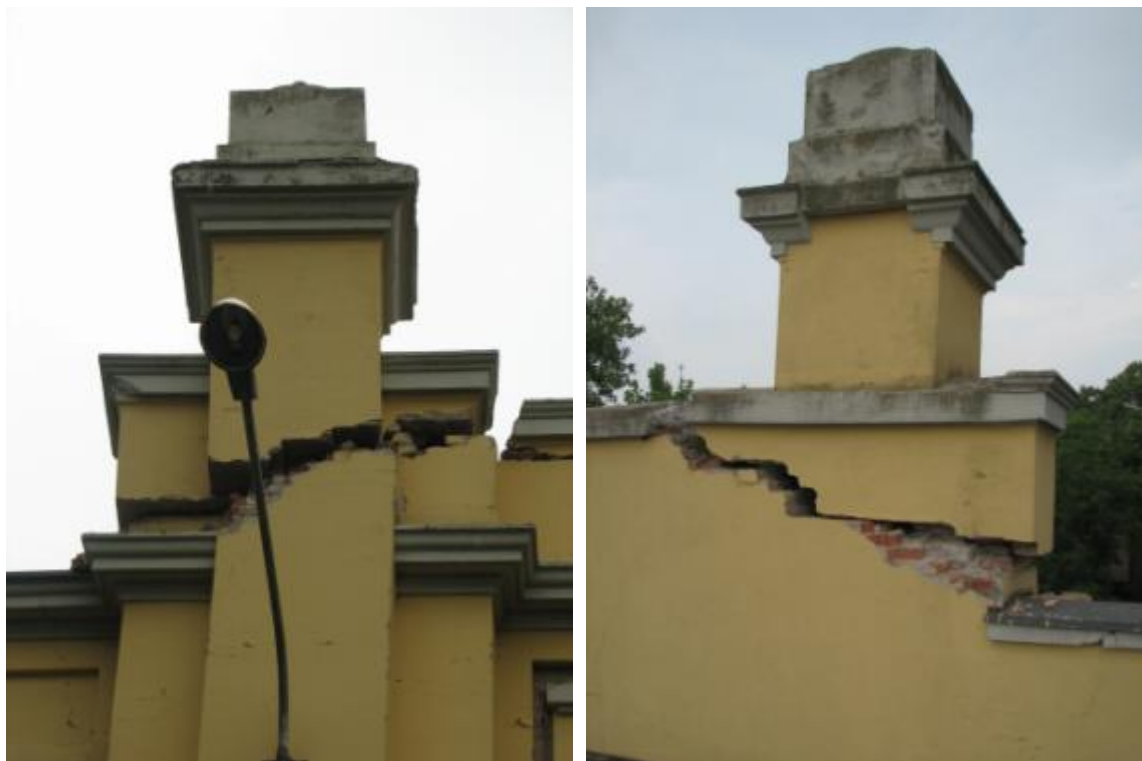
Figure 7-93 Unsafe architectural elements
