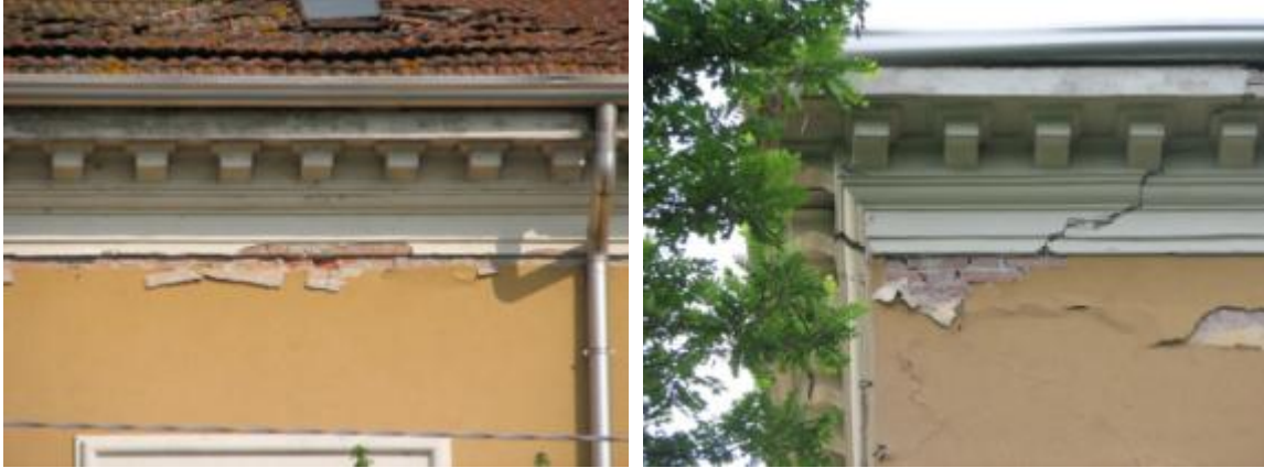
Figure 7-95 Crack on external walls
