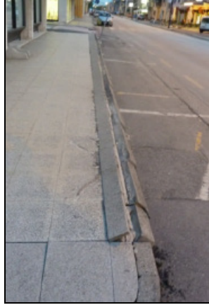
Figure 9-3 Damage to the footpath in Mirabello due to lateral spreading
