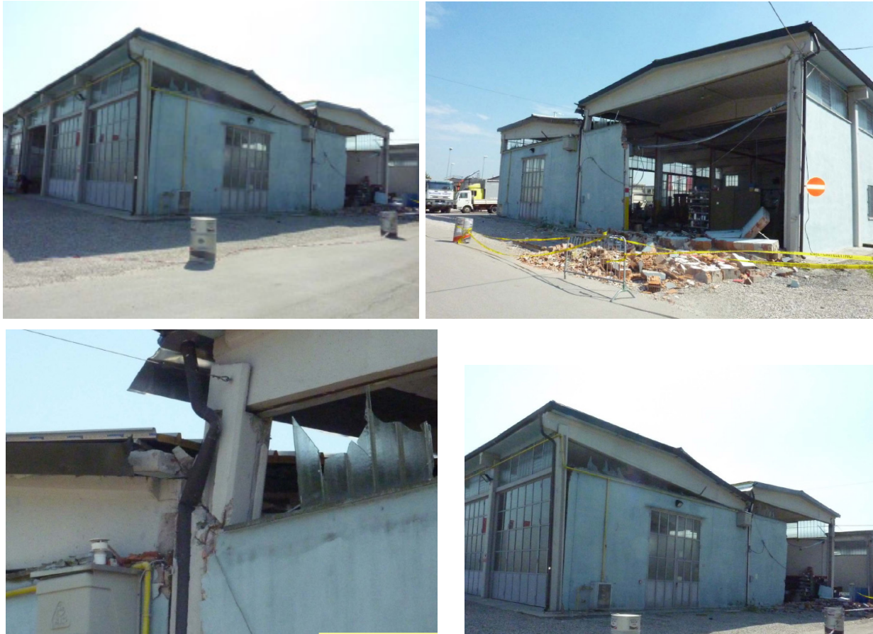
Figure 6-16 Negative effect of irregular cladding (San Felice sul Panaro)
