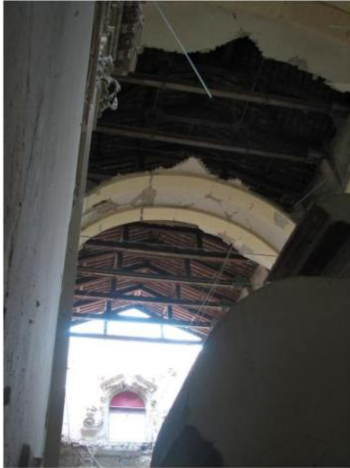
Figure 7-30 Collapsed roof
