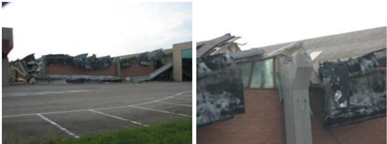
Figure 6-11 (a) Lateral overturning of the beam (b) structural detail
