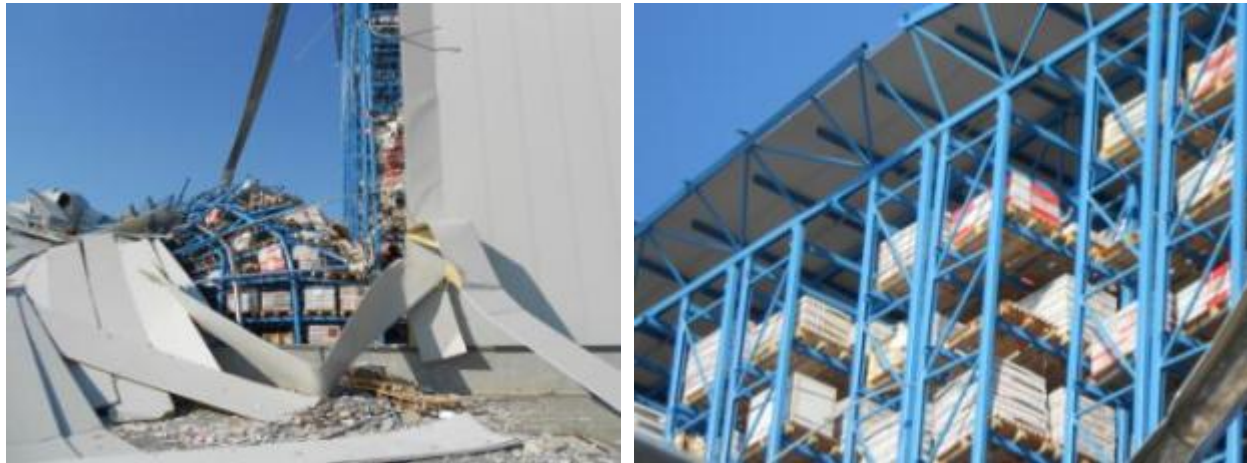
Figure 6-59 (a) Damage to the sandwich insulation panels; (b) roof detail
