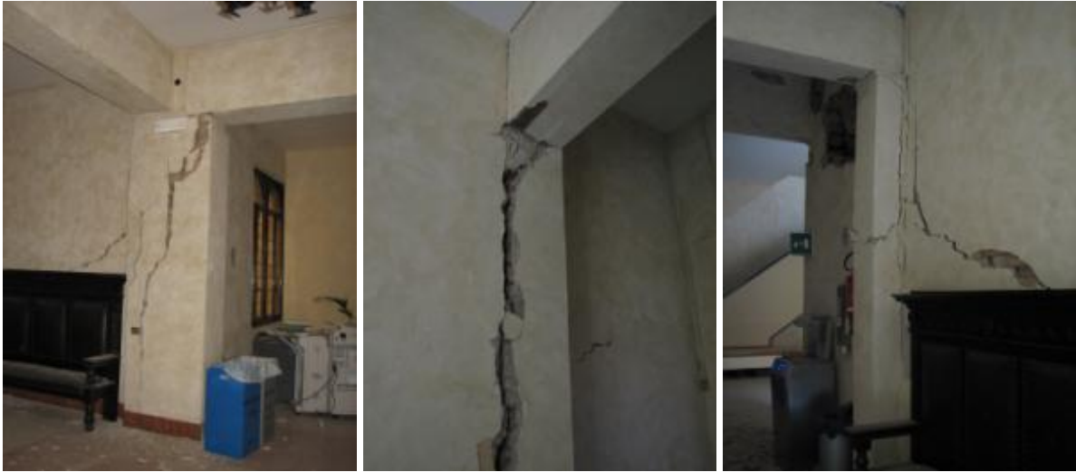
Figure 7-73 Cracks on internal walls
