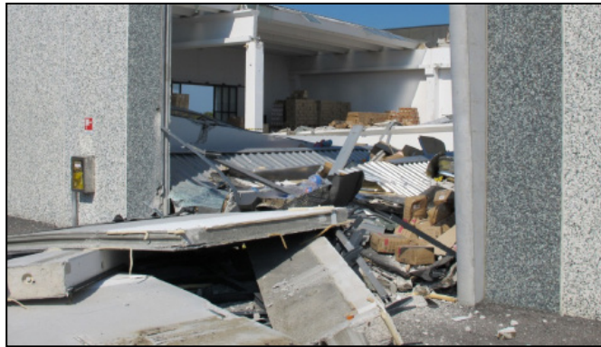
Figure 6-33 Probable collapse of internal pillar
