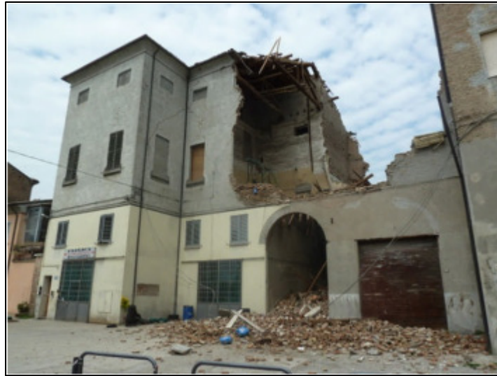
Figure 4-6 Collapse of a masonry house in Finale Emilia
