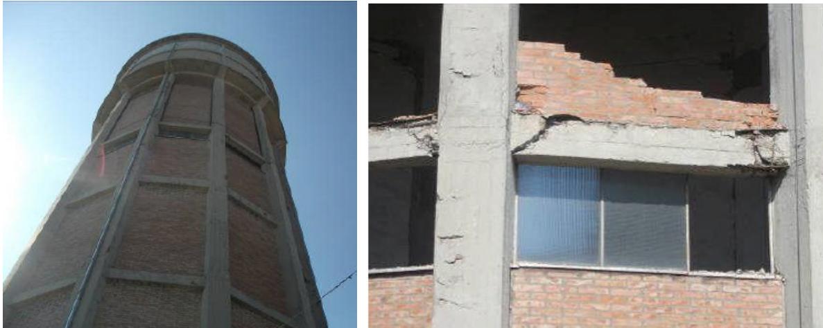
Figure 9-2 Water tank in San Felice sul Panaro and plastic hinges in the beam
