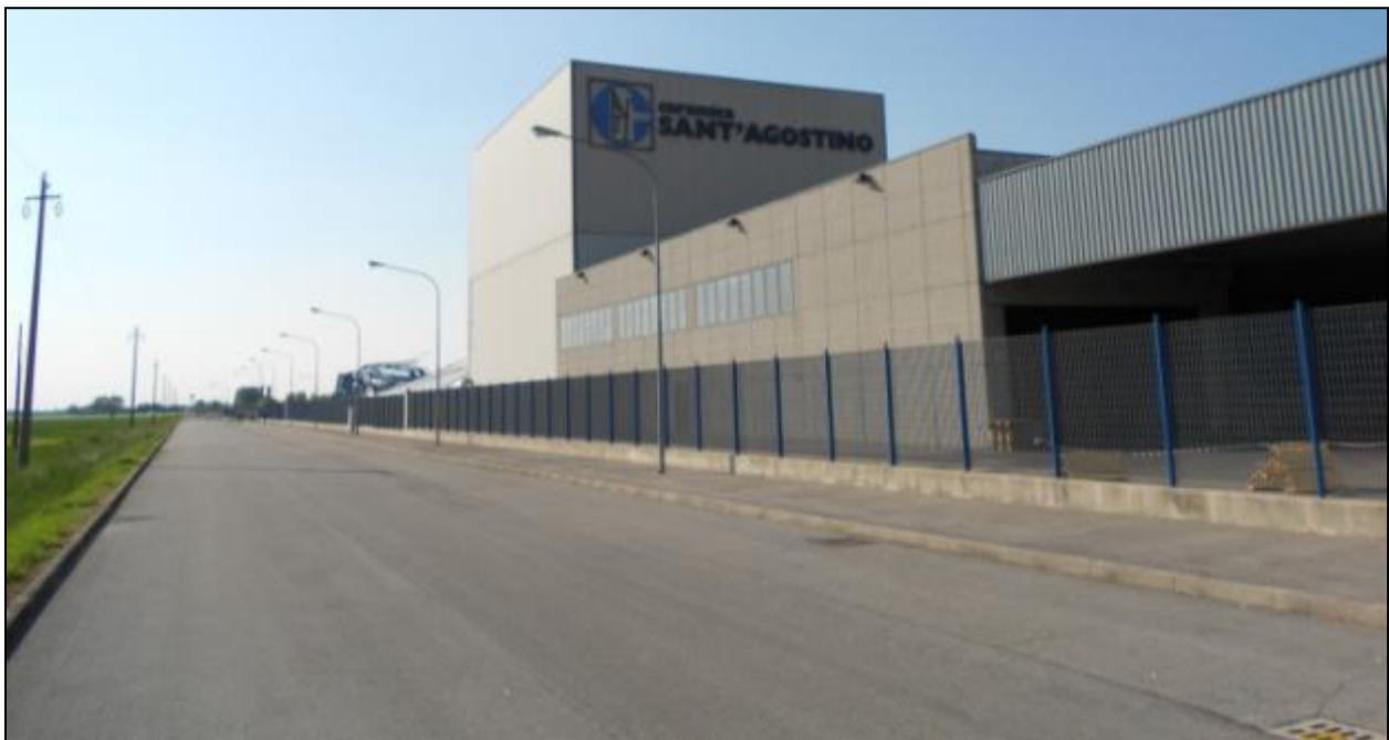
Figure 6-56 Automated storage warehouse of Sant'Agostino ceramics factory: overview
