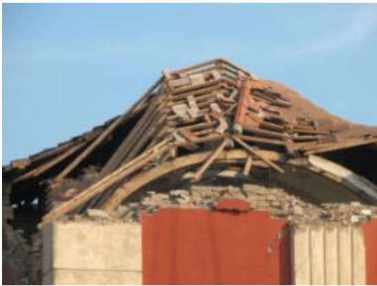
Figure 7-47 Collapsed roof
