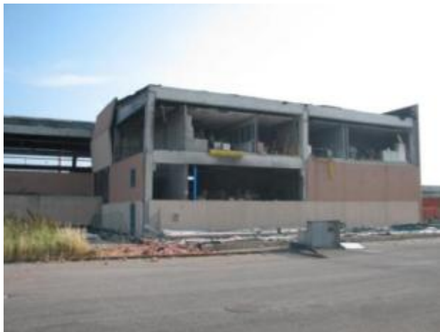
Figure 6-43 Detachment of horizontal panels that were not well-connected to the pillar
