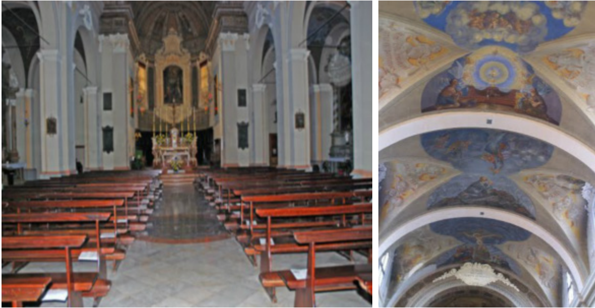
Figure 7-52 Internal view of the church before the earthquake
