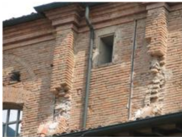
Figure 7-29 External damage and collapsed buttresses
