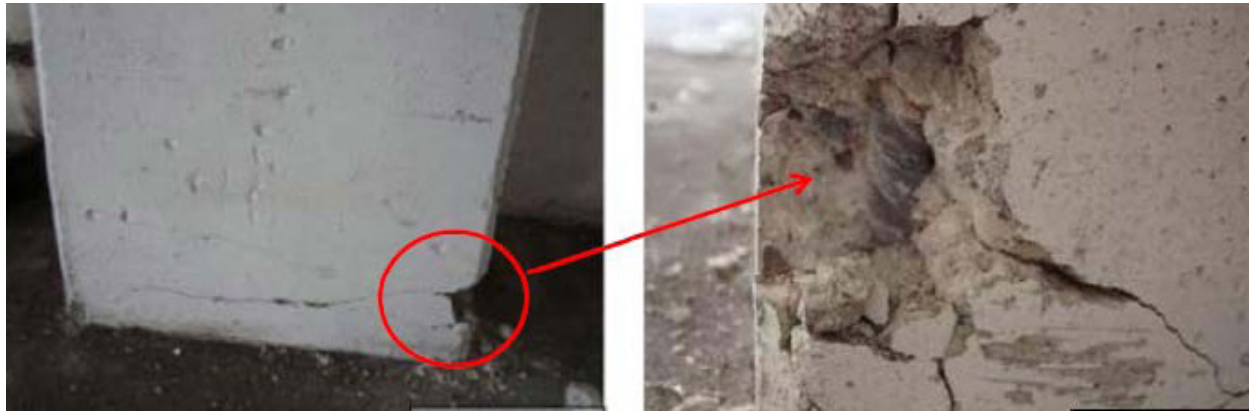
Figure 6-55 Plastic hinge at the base of the pillar
