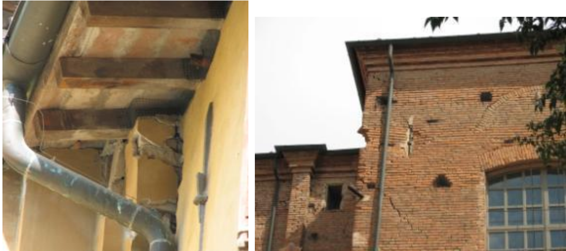
Figure 7-89 Masonry crushing at the tie rod anchorage
