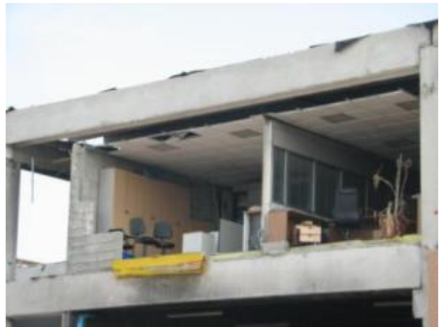
Figure 6-42 Horizontal panels only added mass and did not add stiffness to the structure
