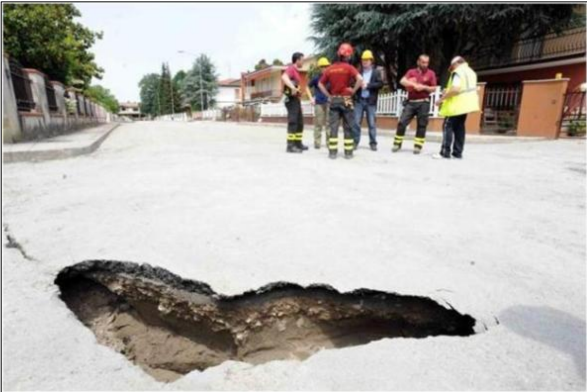
Figure 5-1 Liquefaction in San Carlo
