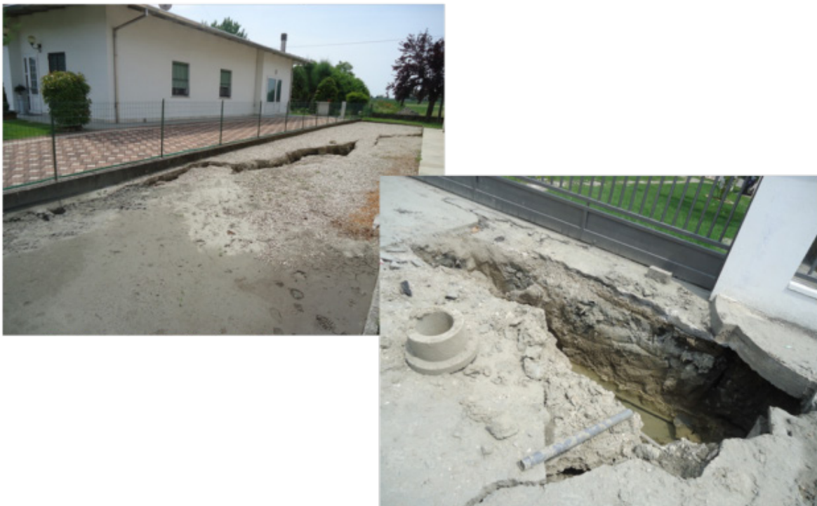
Figure 5-9 Structural damage due to liquefaction in San Carlo (Sant'Agostino)
