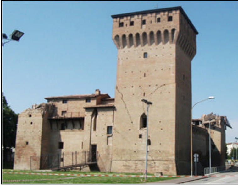
Figure 7-82 Partial collapse of the two towers and severe damage to third tower
