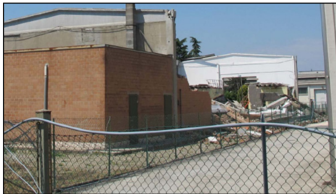
Figure 6-23 Collapse of the intermediate span due to the presence of cladding
