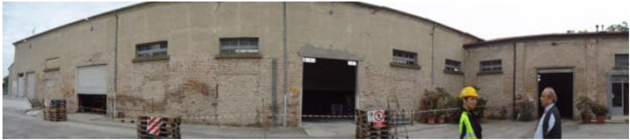
Figure 6-68 Masonry industrial structure in Reno Centese
