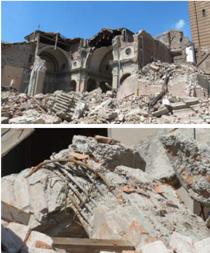
Figure 7-62 Collapse of reinforced concrete element
