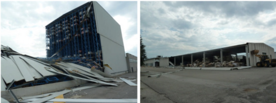
Figure 4-5 Collapse of a ceramic tile warehouse in S. Agostino
