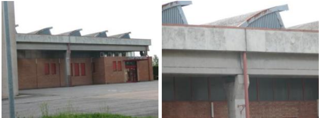
Figure 6-10 Overview of the gymnasium before the earthquake (Mirandola)
