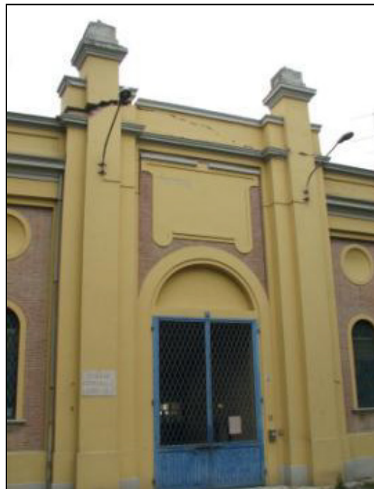
Figure 7-92 Façade of the stadium
