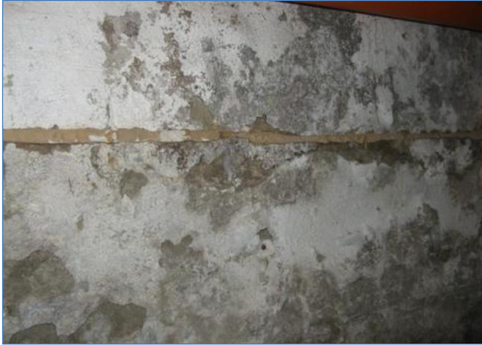
Figure 7-5 Physical cut at level of foundation
