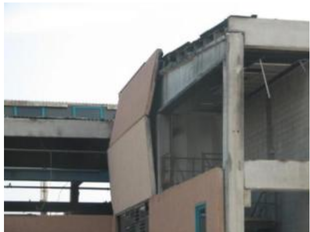
Figure 6-43 Detachment of horizontal panels that were not well-connected to the pillar
