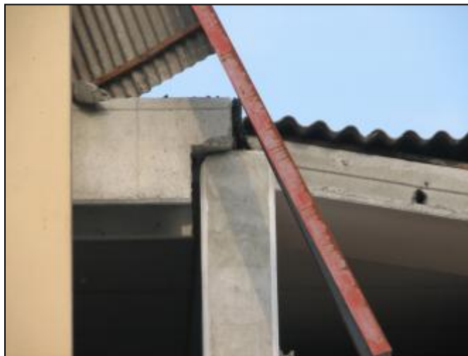
Figure 6-9 Insufficient beam-column support without restraints (Mirandola)
