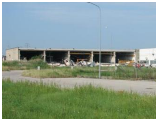
Figure 6-29 Collapse of vertical panels
