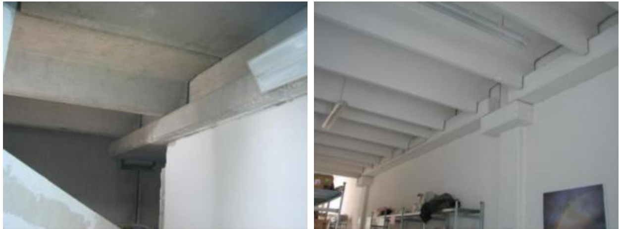
Figure 6-66 Absence of seismic connections
