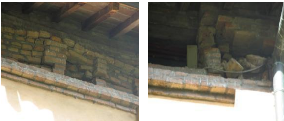
Figure 7-85 Walls under the roof
