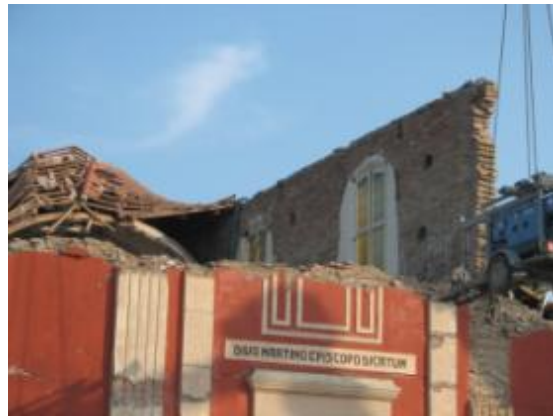
Figure 7-47 Collapsed roof
