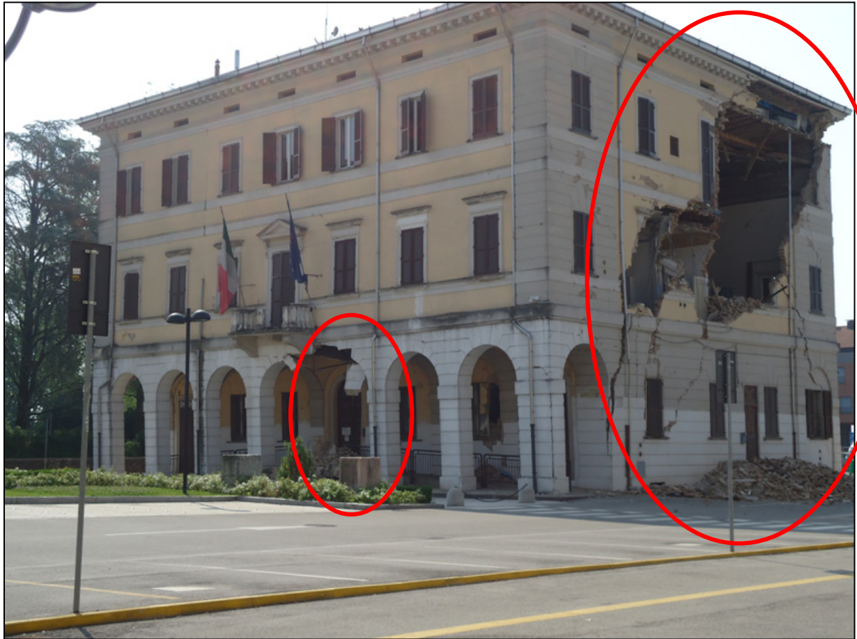
Figure 7-63 City hall of Sant'Agostino – Fallen column and collapse of external wall
