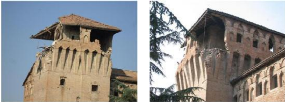
Figure 7-80 Collapse of the tower of the castle in Finale Emilia
