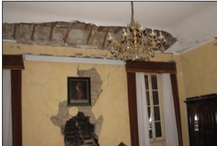
Figure 7-74 Partial collapse of the floor
