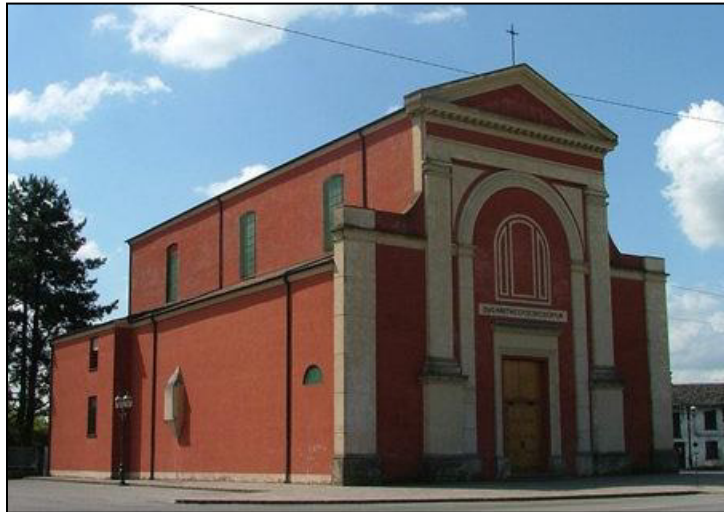
Figure 7-44 San Martino Church before the earthquake
