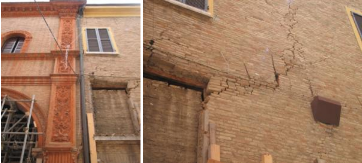
Figure 7-70 Shear crack on the external walls
