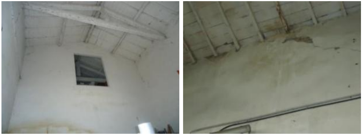
Figure 6-69 Overview of the internal wooden roof
