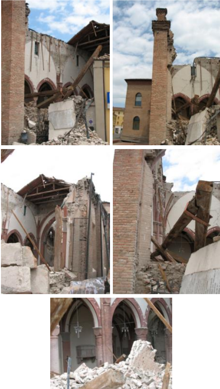
Figure 7-38 Internal view of the church after the earthquake
