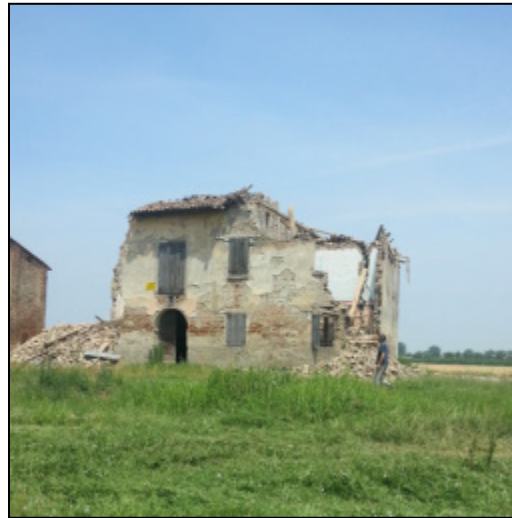
Figure 10-6 Building investigated with the Danni application
