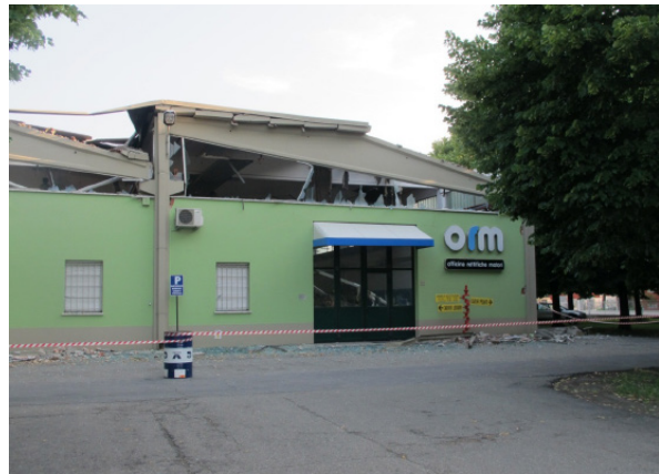
Figure 6-19 Collapse of industrial shed due to seismic behavior of irregular cladding
