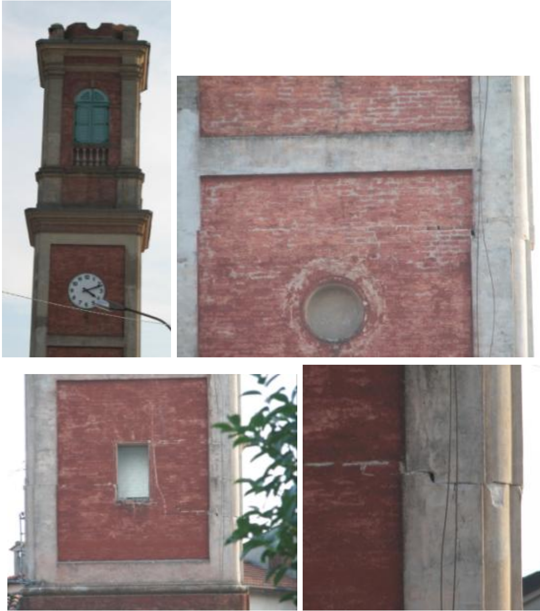
Figure 7-51 Shear fracture was the reason for the demolition
