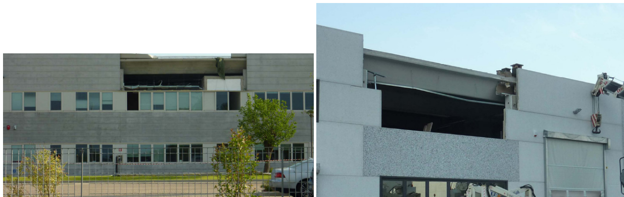
Figure 6-45 Detachment of horizontal panels that were not well connected to the pillar in Sant'Agostino
