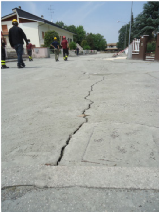
Figure 5-12 Damage due to liquefaction
