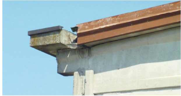
Figure 6-12 Dangerous heavy nonstructural elements
