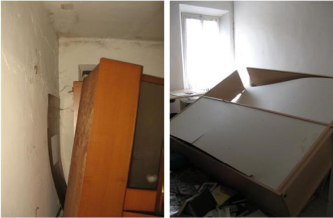
Figure 7-7 Overturning effects: This building has been classified as non-accessible
