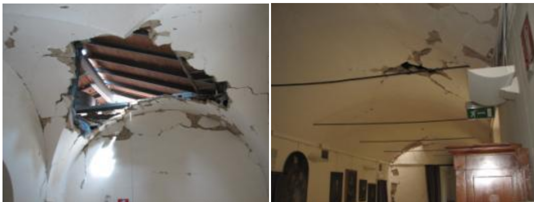
Figure 7-88 Partial collapse of the roof
