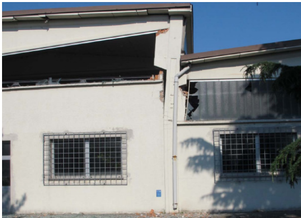
Figure 6-19 Collapse of industrial shed due to seismic behavior of irregular cladding
