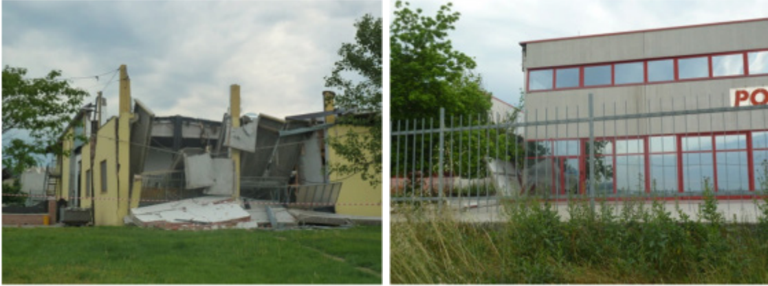
Figure 4-4 Damage to industrial facilities in San Carlo
