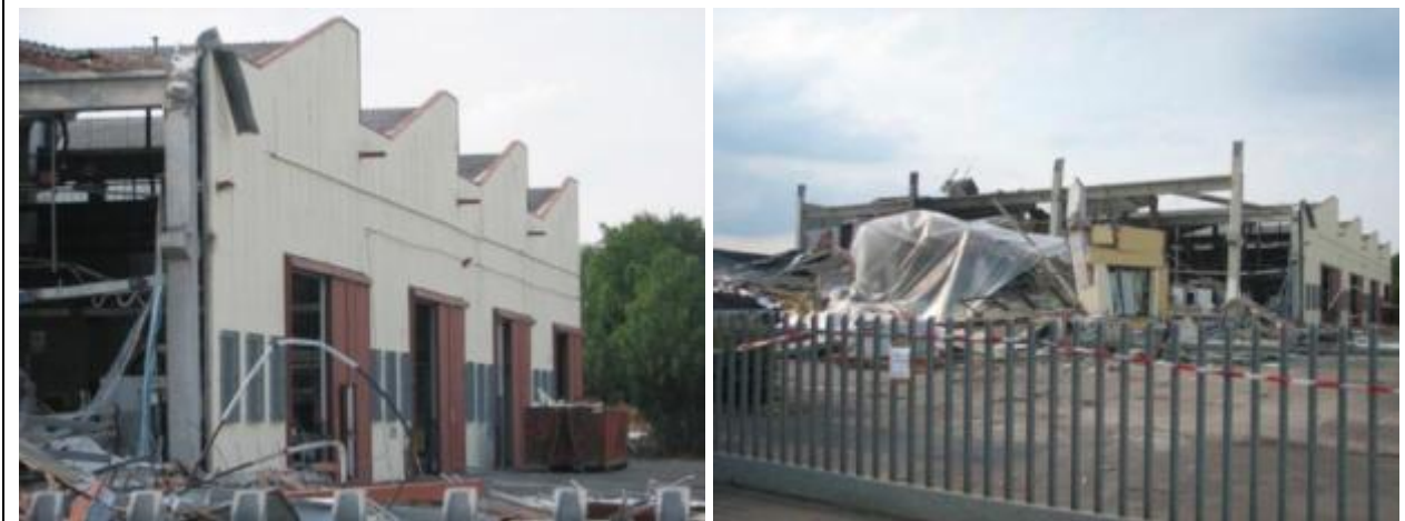
Figure 6-4 Overview of industrial shed of BBG.srl
