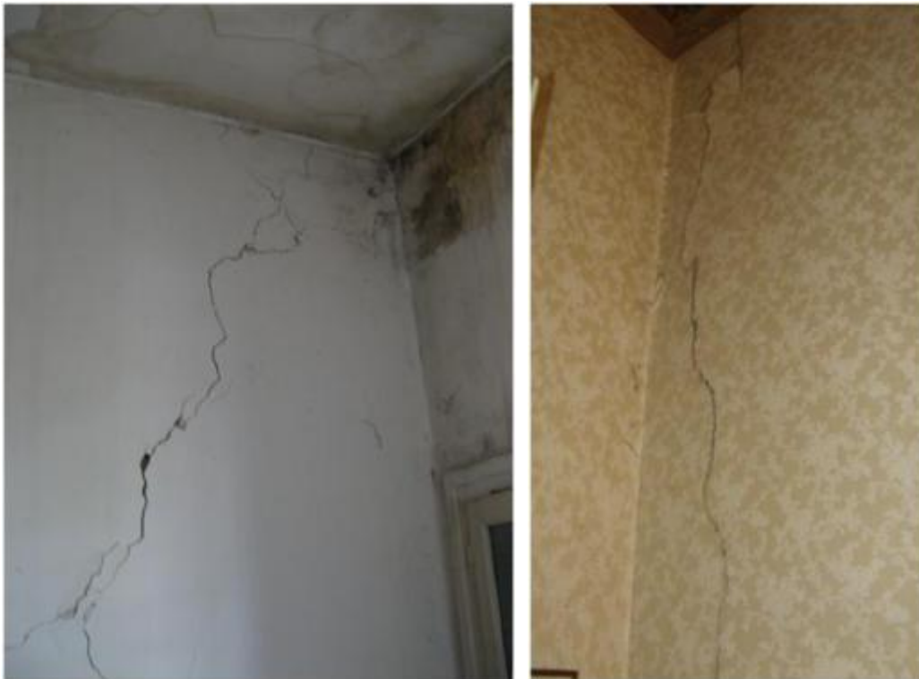
Figure 7-6 Lesions on load-bearing walls
