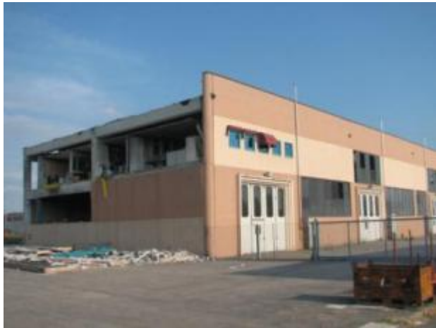
Figure 6-42 Horizontal panels only added mass and did not add stiffness to the structure
