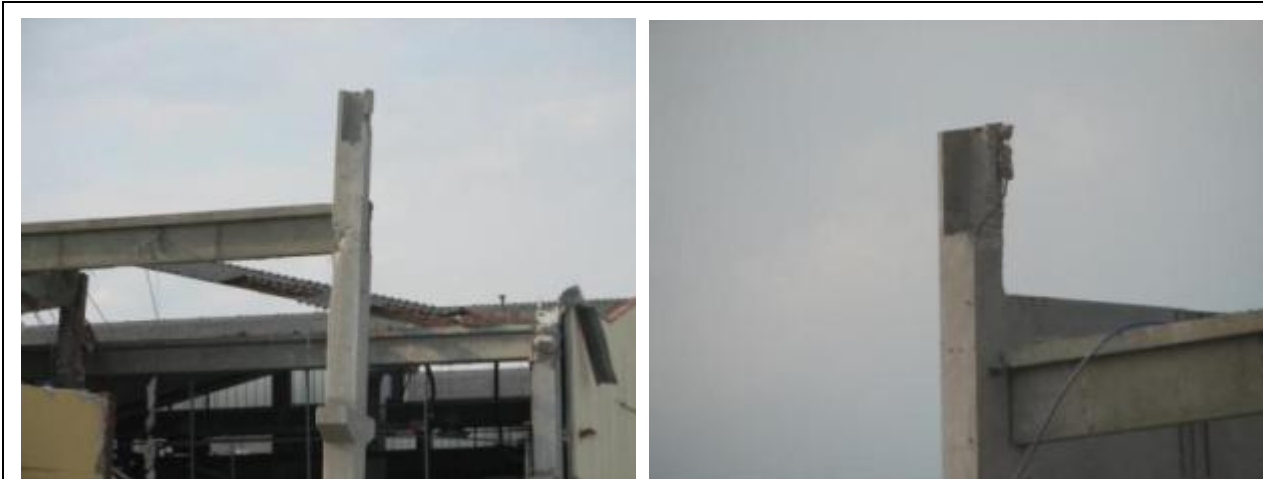
Figure 6-5 Shear keys with no reinforcement of BBG.srl
