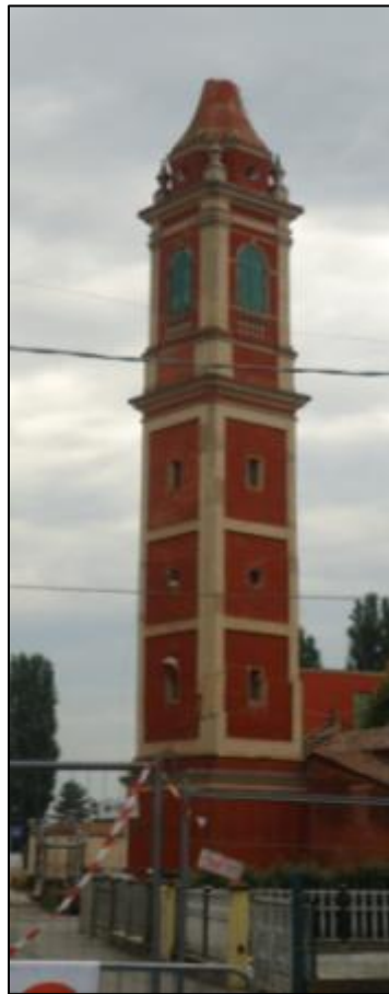
Figure 7-49 San Martino bell tower after the earthquake and before the demolition
