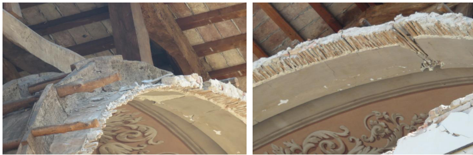
Figure 7-21 Example of reed mat false vaults
