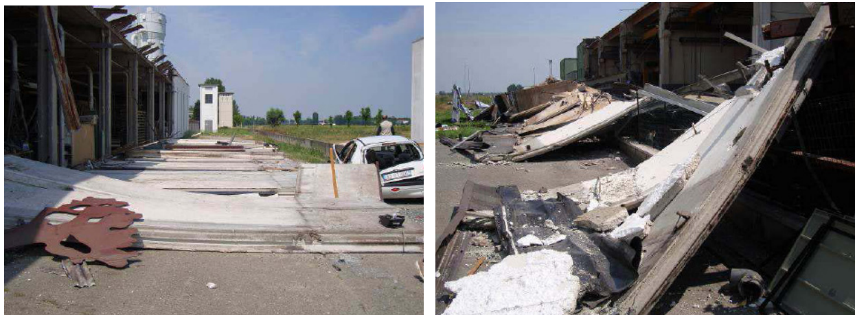
Figure 6-41 Collapse of vertical panels not attached to the foundation curb
