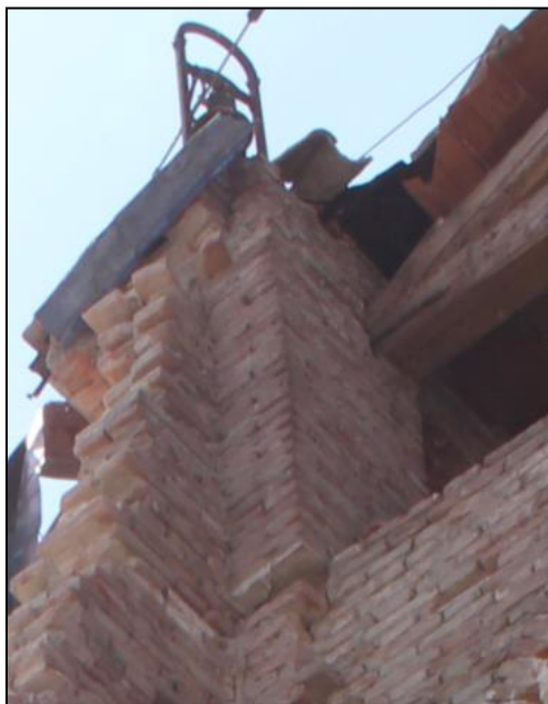
Figure 7-13 Double wall supports a timber truss
