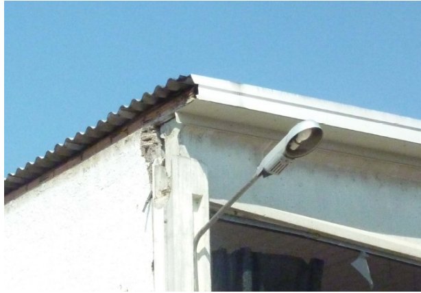
Figure 6-12 Dangerous heavy nonstructural elements
