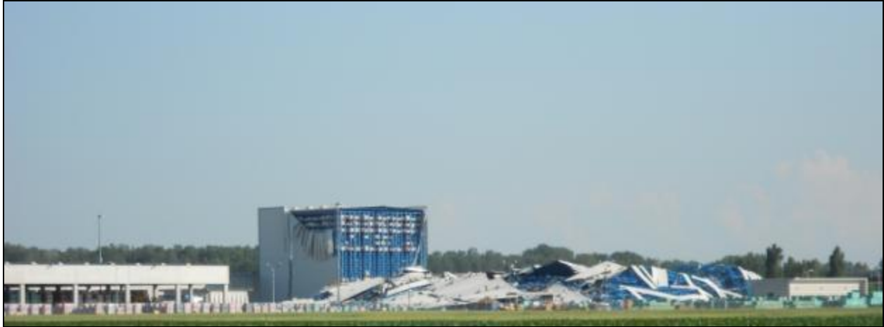
Figure 6-57 Damage overview of automated storage warehouse of Sant'Agostino ceramics factory
