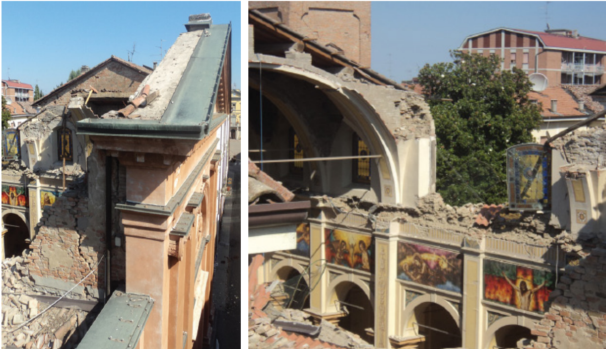
Figure 8-4 Church of St. Paul and its damage
