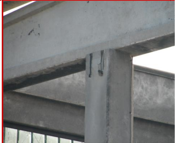
Figure 6-34 Beam-column connection without sufficient reinforcement in the beam head
