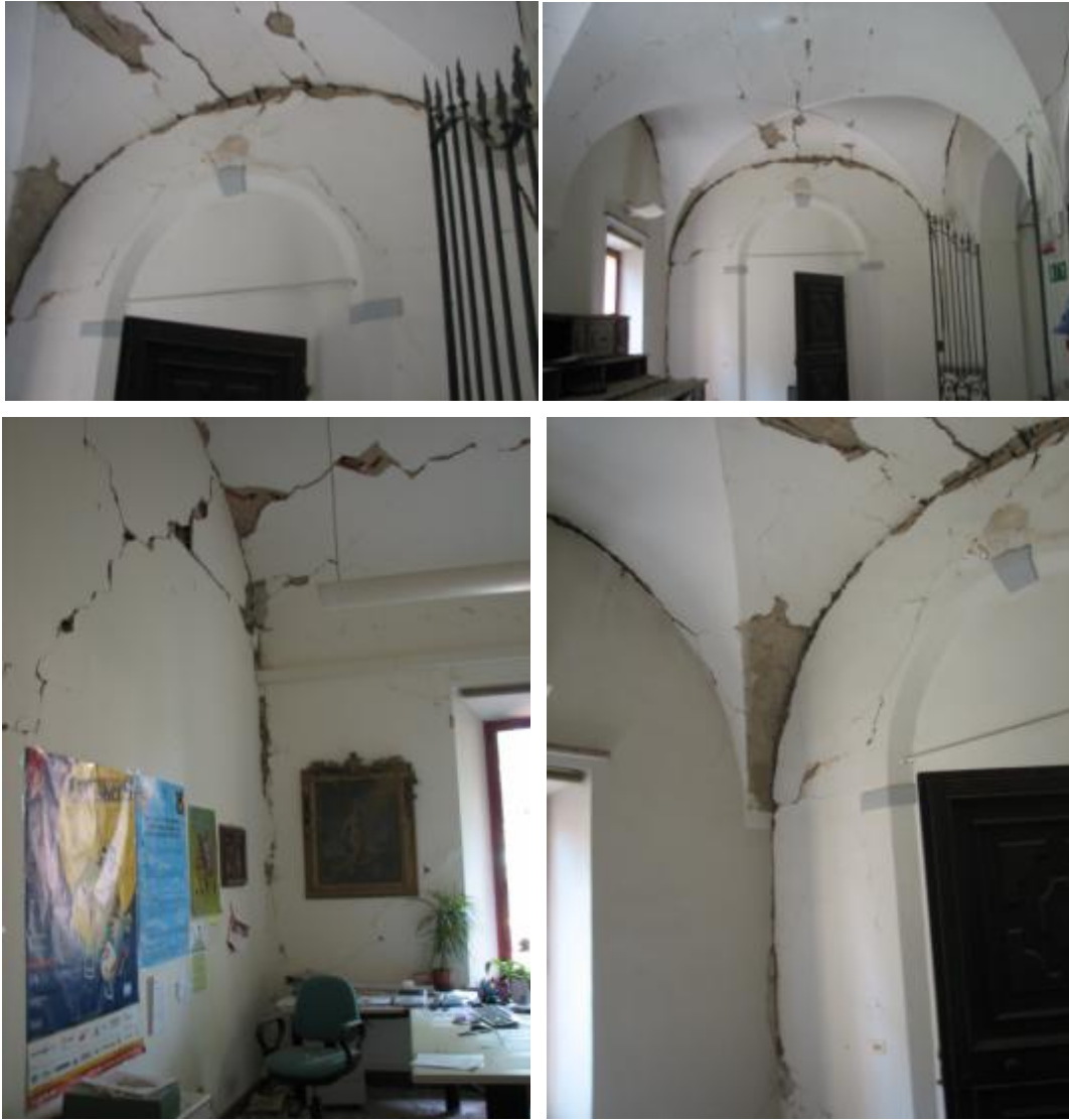
Figure 7-87 Damage to the vaults
