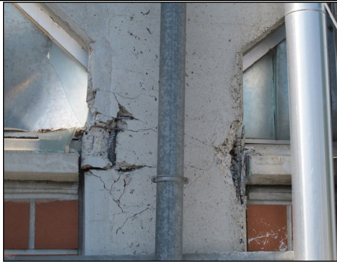
Figure 6-22 Plastic hinge in the column due to the presence of irregular cladding
