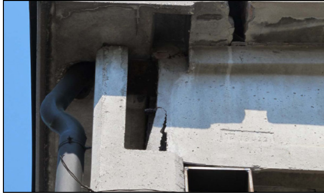
Figure 6-24 Beam-column connection without sufficient reinforcement in the beam head
