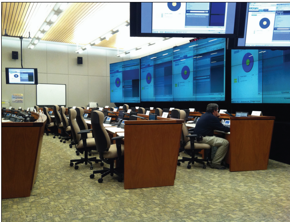
Figure 3-1. Emergency Operations Center, New Jersey Office of Emergency Management
