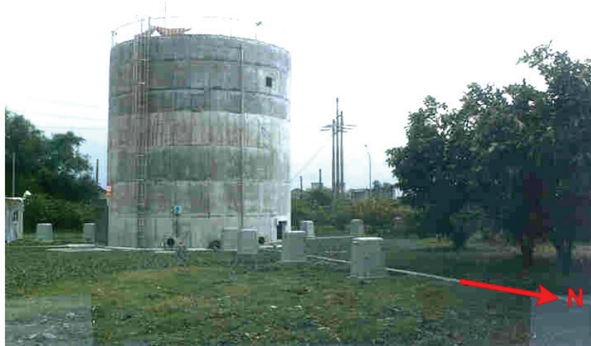
Figure 2-5: Lotung model containment structure ( www.earth.sinica.edu.tw/~smdmc/llsst/llsst.htm )
