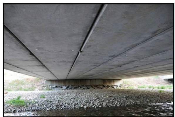
Figure 6-7. Adjacent Prestressed Concrete Box Beams (O'Connor)
