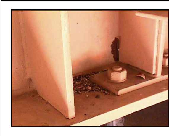
Figure 5-16. Moderate Damage: Crack in Web of Steel Girder. Note that this may be a red flag condition if it is in the primary member. (CPHMR)
