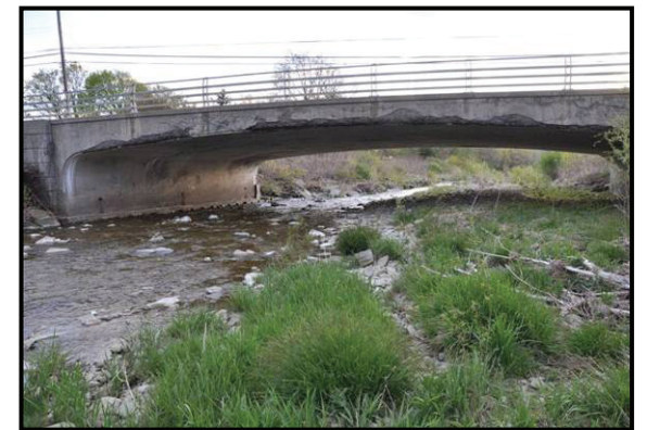
Figure 6-5. Reinforced Concrete Arch
