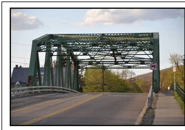
Figure 6-6. Steel Through Truss
