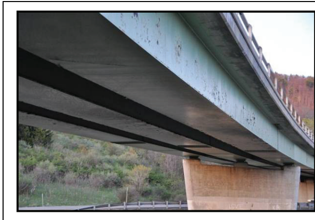
Figure 6-4. Steel Box Girder
