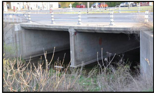
Figure 6-11. Concrete Box Culvert
