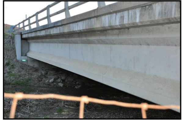
Figure 6-3. Prestressed Concrete Girder
