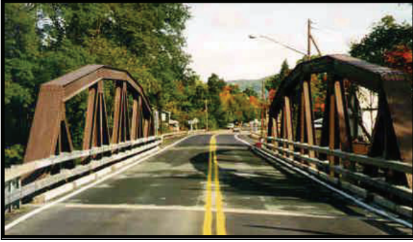
Figure 6-8. Steel Pony Truss
