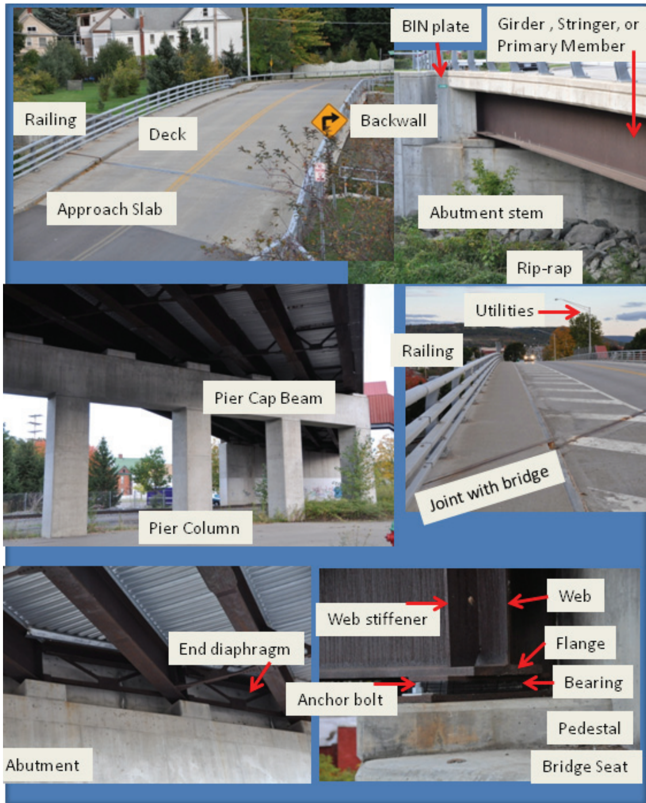
Figure 6-1. Bridge Terminology Reference Sheet (O'Connor)
