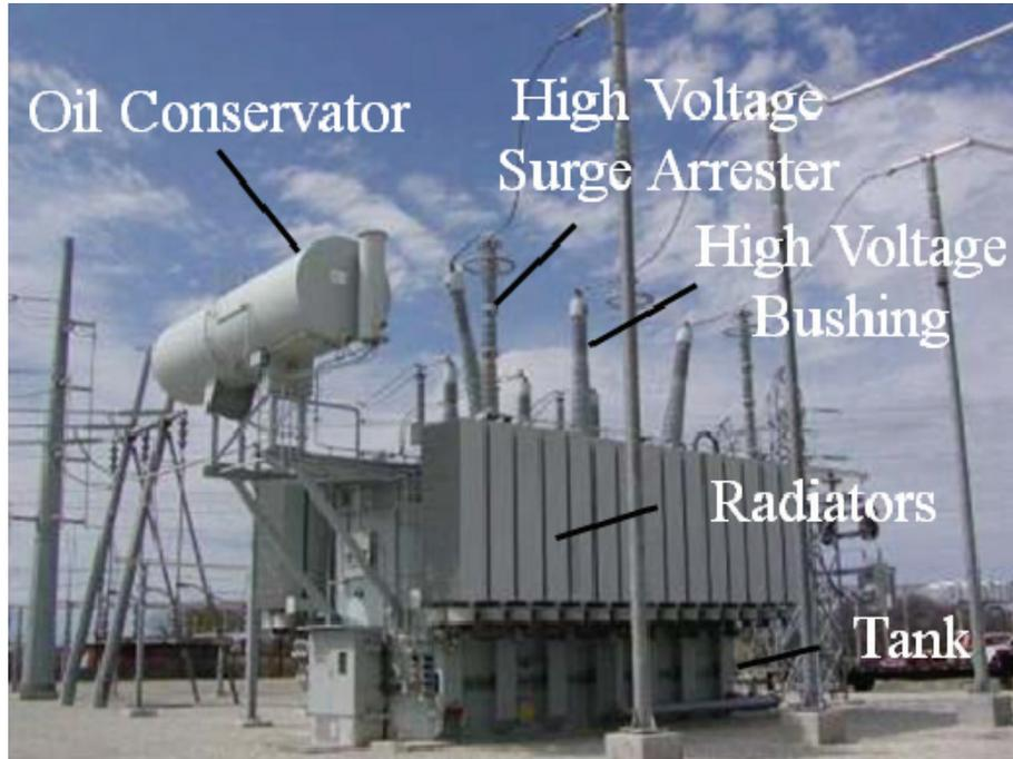
**Figure 2-1 Typical three phase high voltage transformer**
